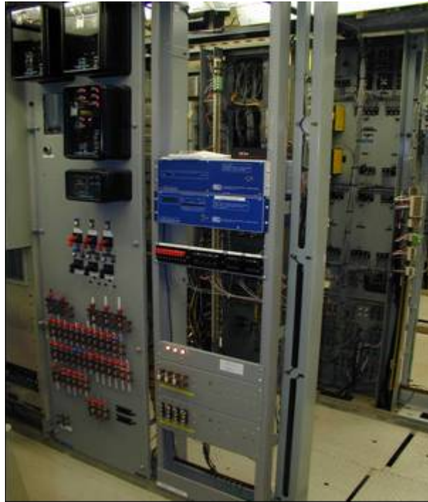
Figure 27: Digital Primary Schweitzer Relays
