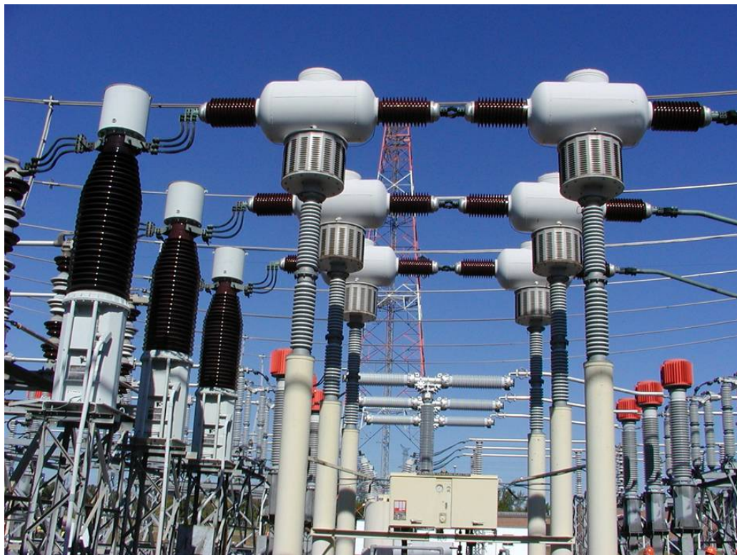
Figure 3: 230 kV Air Blast Circuit Breaker
