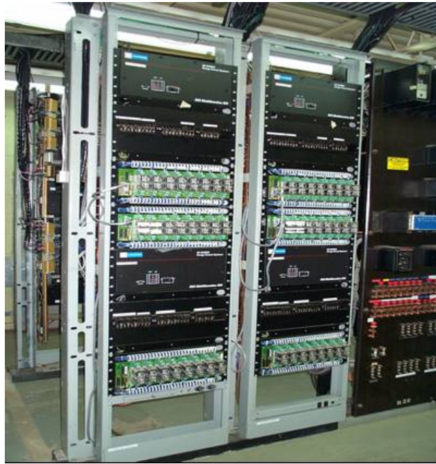
Figure 31: GE D25 Distributed RTU Installation - 1999
