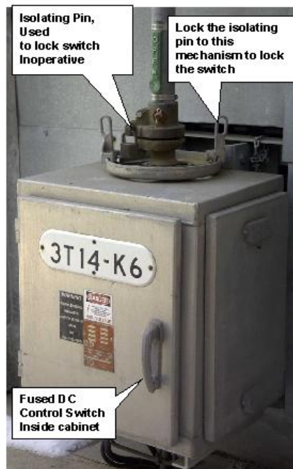
Figure 13: Motor Operating Mechanism for a Switch
