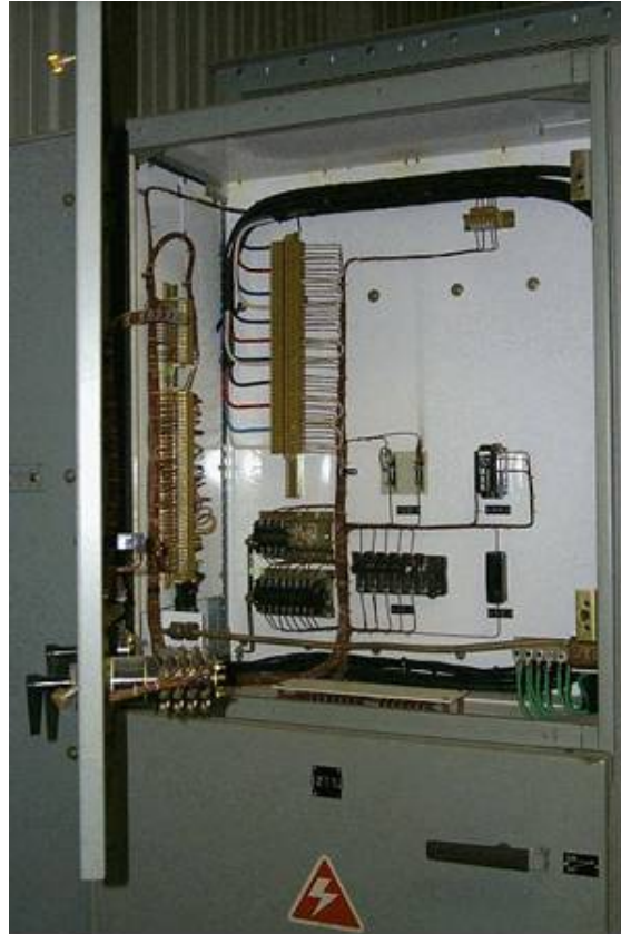
Figure 8: Control Compartment
