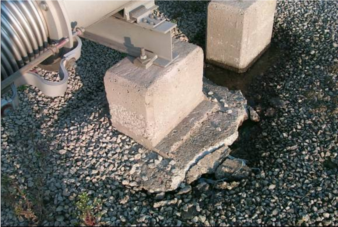
Figure 24: Damaged Footing of a SF 6 Bus Duct
