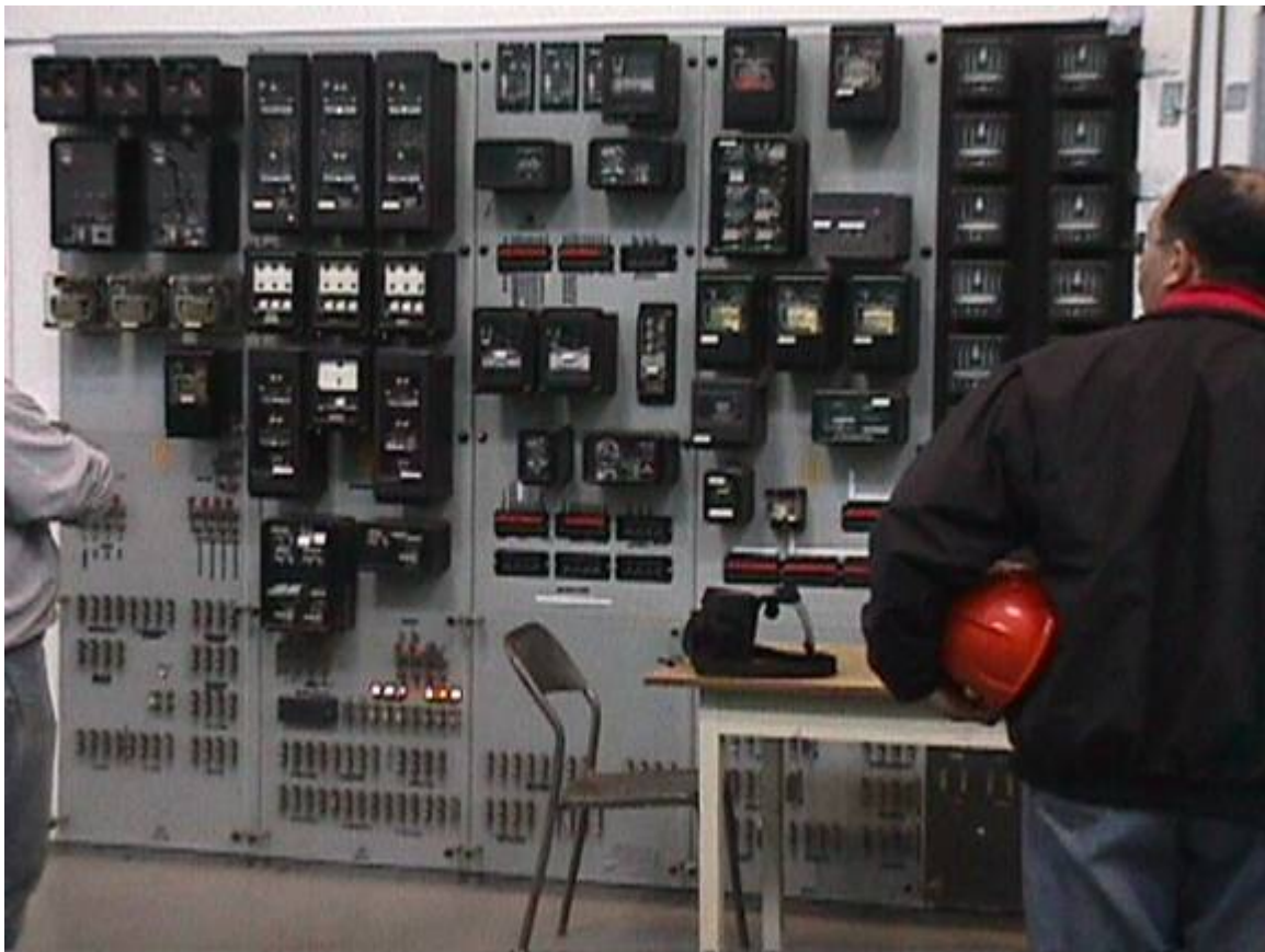
Figure 30: 24 Inch Steel-Type Panels with Protection, Auxiliary Relays, Flexitest Switches and Current Links
