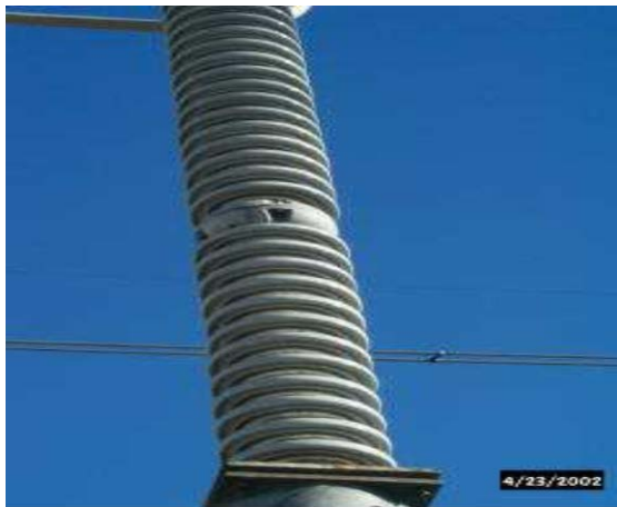
Figure 15: Station Porcelain Post Insulator
