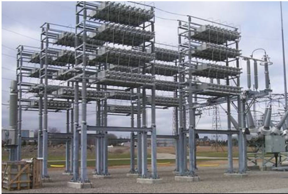
Figure 17: Capacitor Bank
