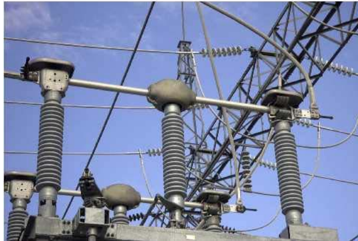
Figure 12: Center Rotating Disconnect Switch
