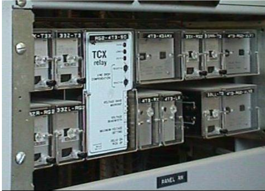
Figure 28: ASEA RX Type Auxiliary Relays
