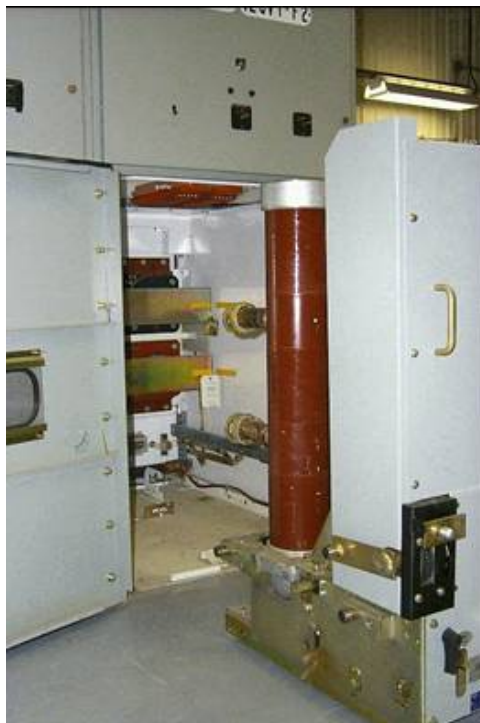
Figure 7: Circuit Breaker Withdrawn from Breaker Compartment
