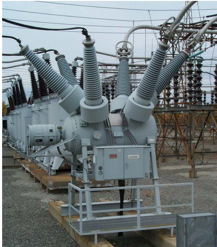
Figure 2: Dead Tank SF 6 Circuit Breaker
