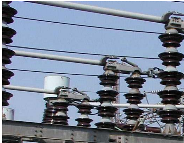
Figure 16: Station Cap and Pin Insulators
