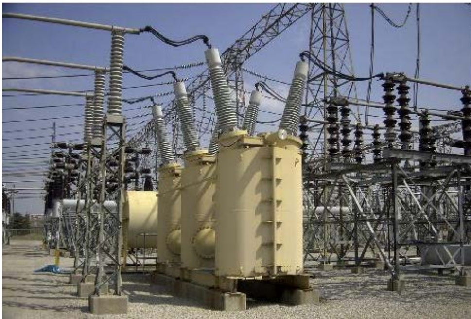
Figure 1 - Three Tank Oil Circuit Breaker
