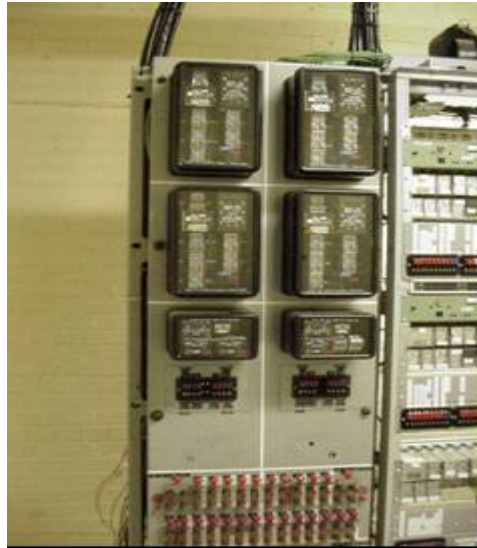
Figure 25: Electromechanical Relay Panel
