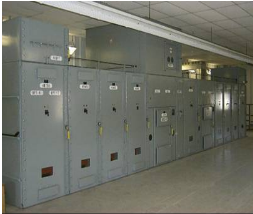
Figure 6: Typical Hydro One Metalclad Switchgear
