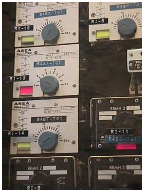
Figure 29: ASEA RR Type Auxiliary Relays
