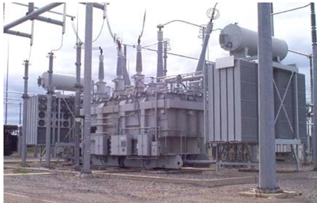
Figure 9: Typical Transmission Station Power Transformer
