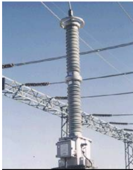
Figure 14: Capacitive Voltage Transformer
