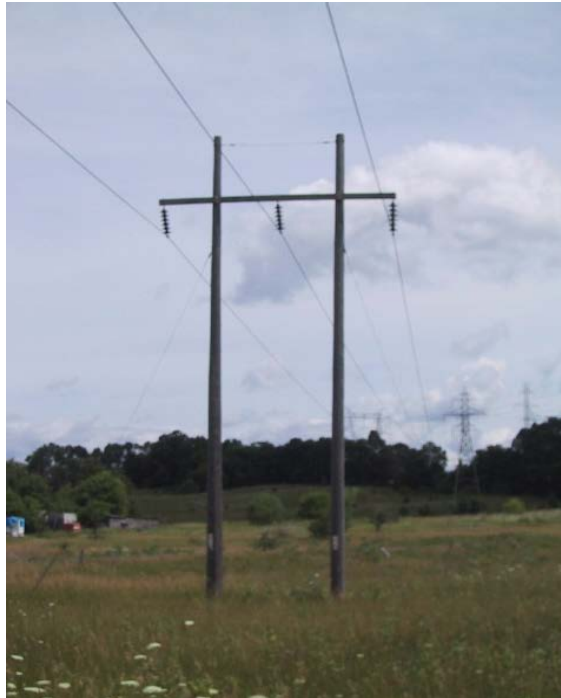
Figure 34: Transmission Line H-Frame Structure
