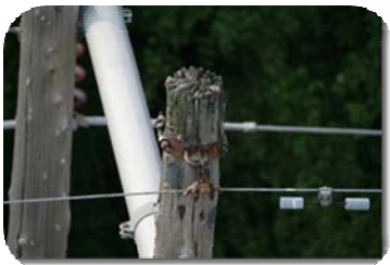
Figure 3: Pole Top Decay / Weathering
