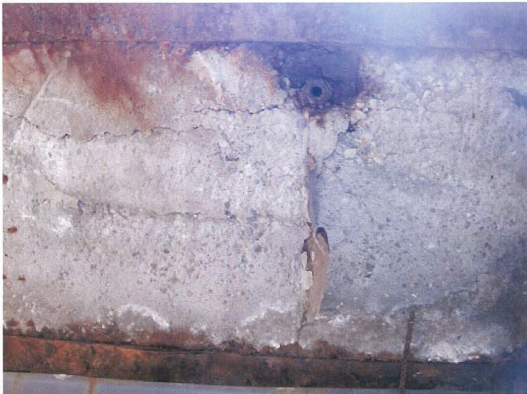
Sample of a Vault Roof slab in need of Replacement
