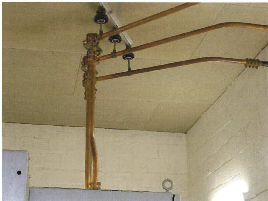
Figure 2: Open 4kV Bus.
