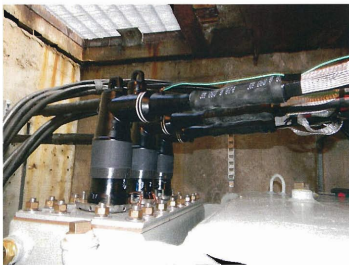
Figure 2: EPR Cable NT Connection.
