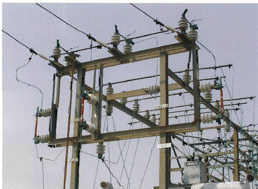
Figure 2 – Substation 97 Overhead Bus
