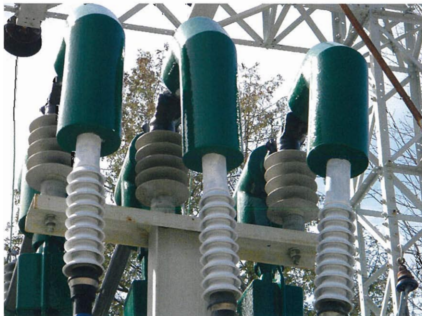
Figure 2 – Substation 35 Covered Bus.
