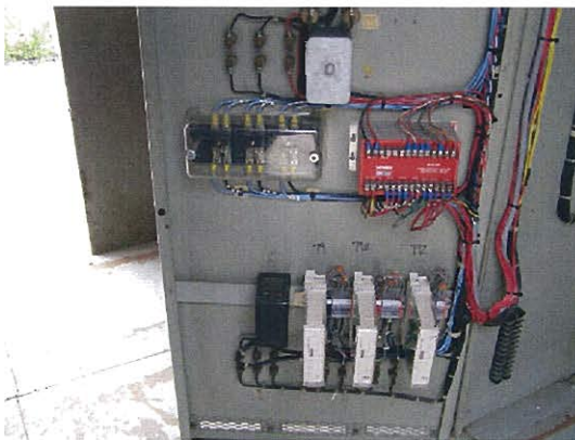
Figure 2: Substation 24 "Like-for-Like" Replacement Relays
