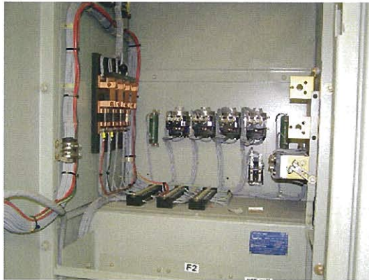
Figure 1: Substation 23 Reclosing-Timer Relays
