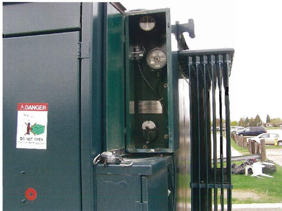
Figure 2: On-line Temperature Monitoring Device
