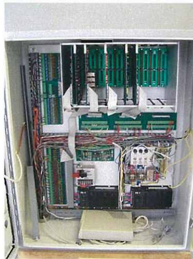
Figure 1 – Rantech Circuit-Board RTU
