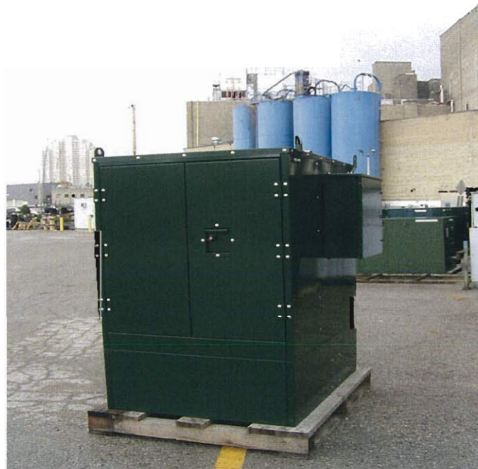
Figure 2 – Replacement T1-L Switch
