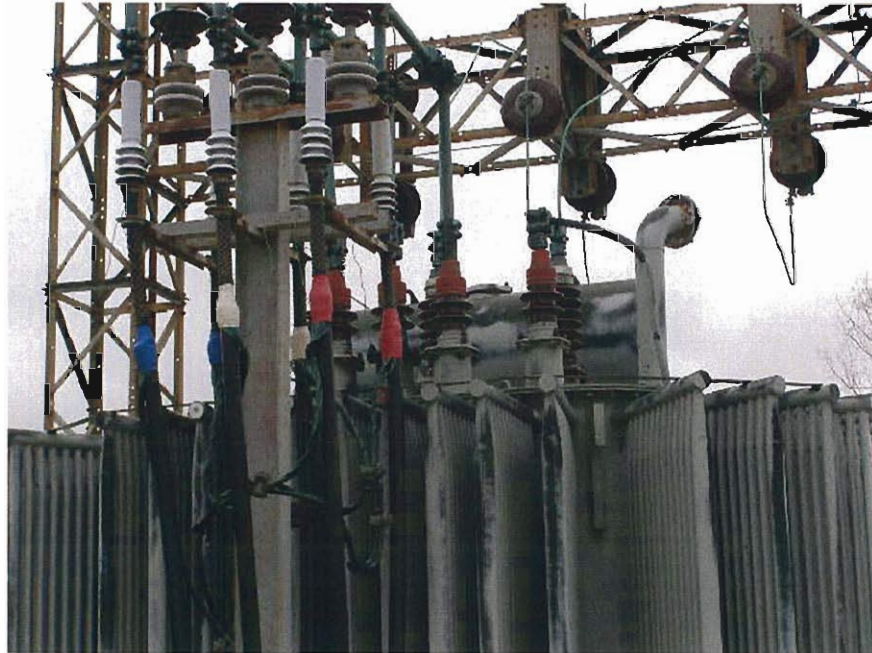
Figure 1 – Substation 49 Exposed Bus.
