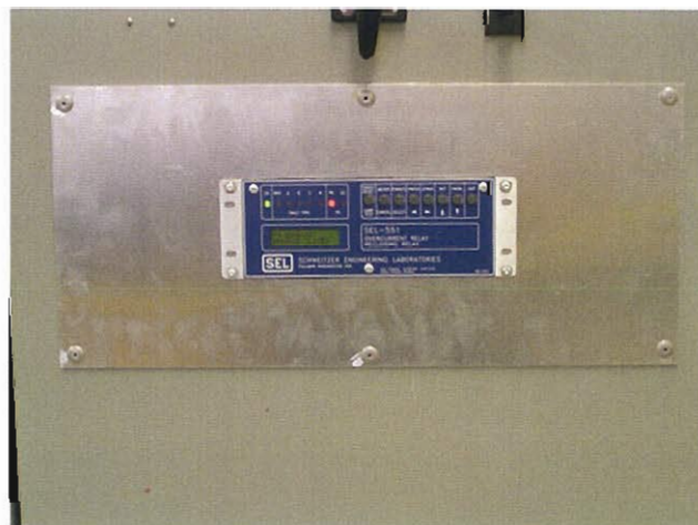
Figure 3: Intelligent Electronic Device (IED) Replacement
