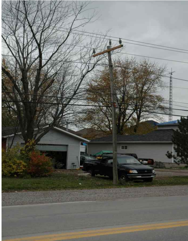
Figure 20: HONI's pre-existing 35-foot class 5 pole with newly constructed 27.6/16 kV crossarm framing on south side of Rymal Road East.
