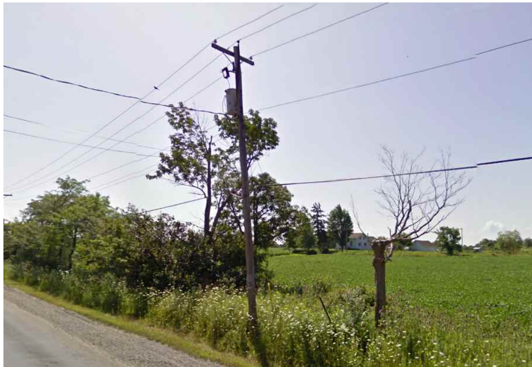
Figure 9: Rural 8.32/4.8 kV distribution system
