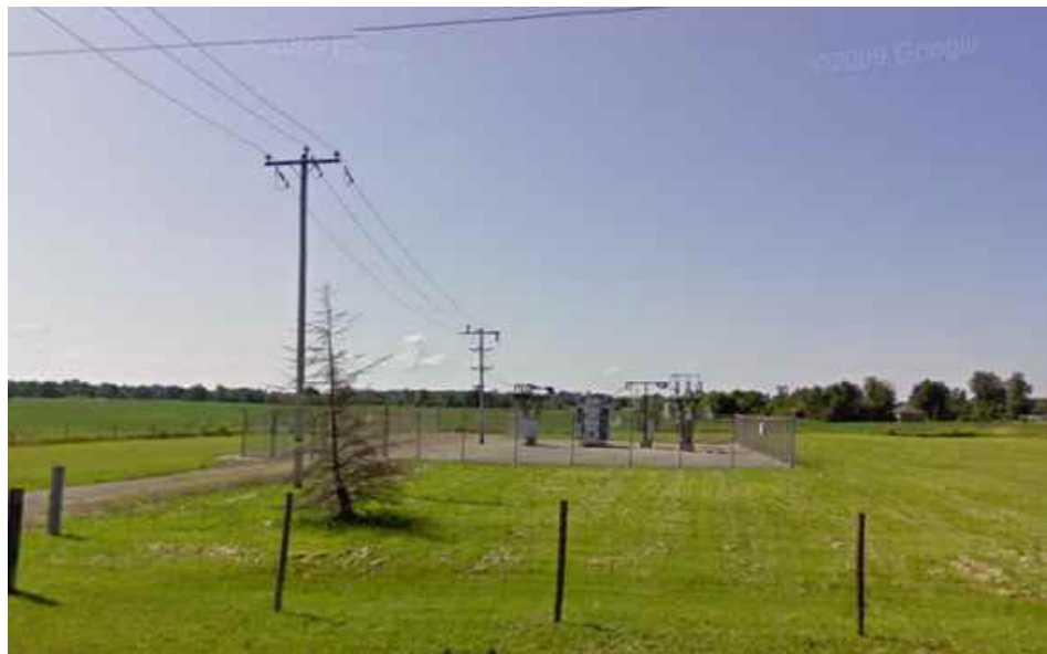
Figure 7: Dickenson DS and 27.6/16kV supply circuit
