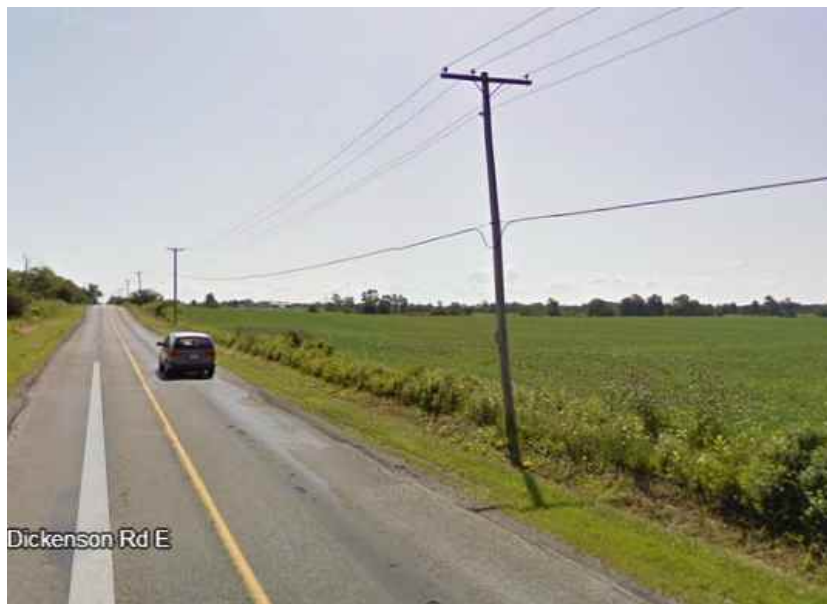
Figure 10: 8.32/4.8kV feeder along Dickenson Road
