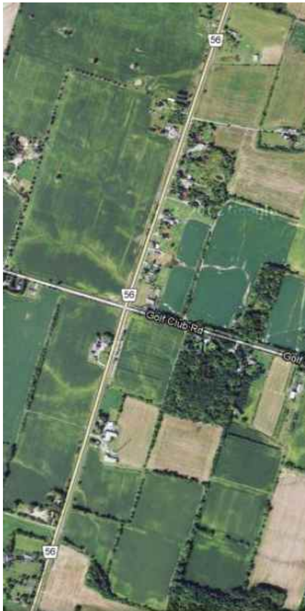
Figure 17: Showing Customers that exist along the approximate 3.1 km stretch between 1314 Highway 56 and Rymal Road East.
