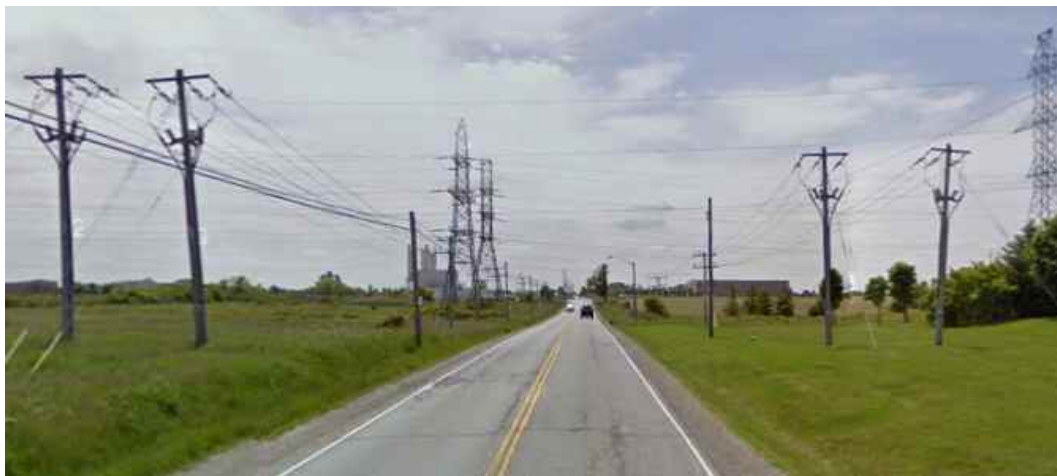
Figure 3: Four circuits tracking south
