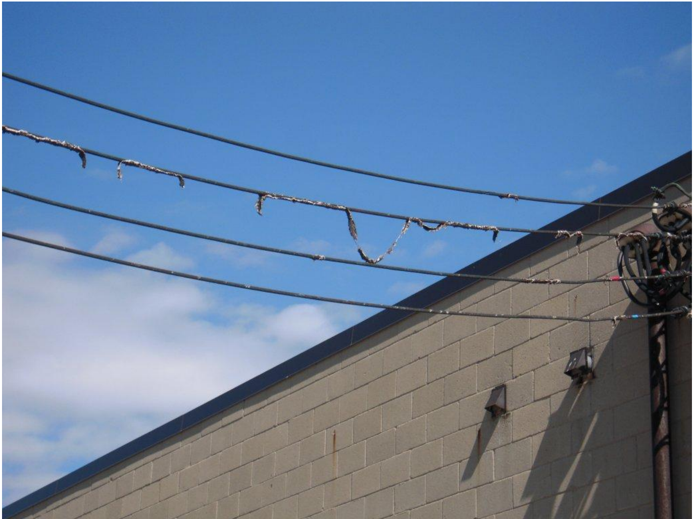
Figure 6 Line damage
