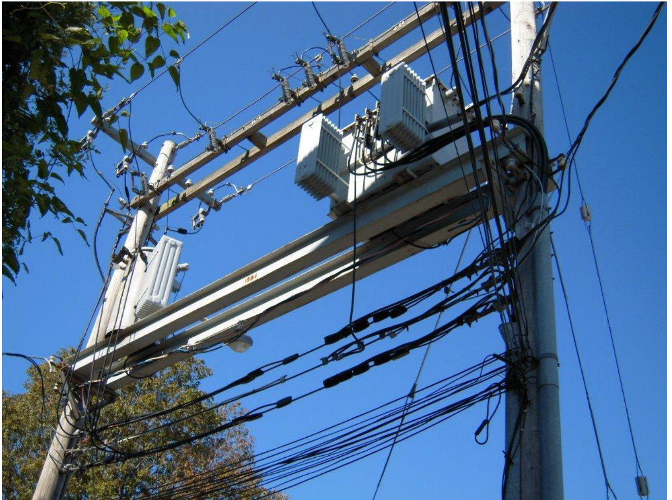
Figure 7 Transformer tied to frame
