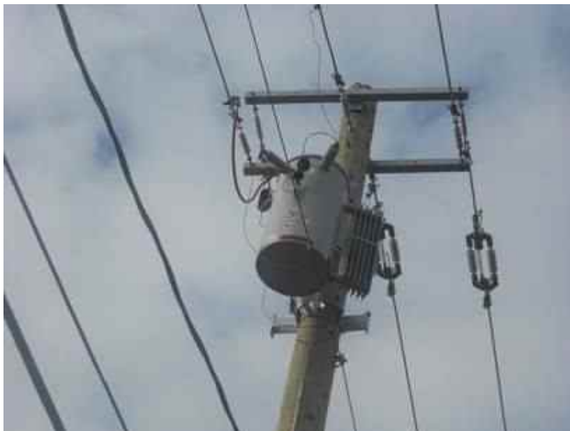
Figure 19: 4.8kV to 16kV “Rabbit” located east of Fletcher Road on the south side of Rymal Road East.
