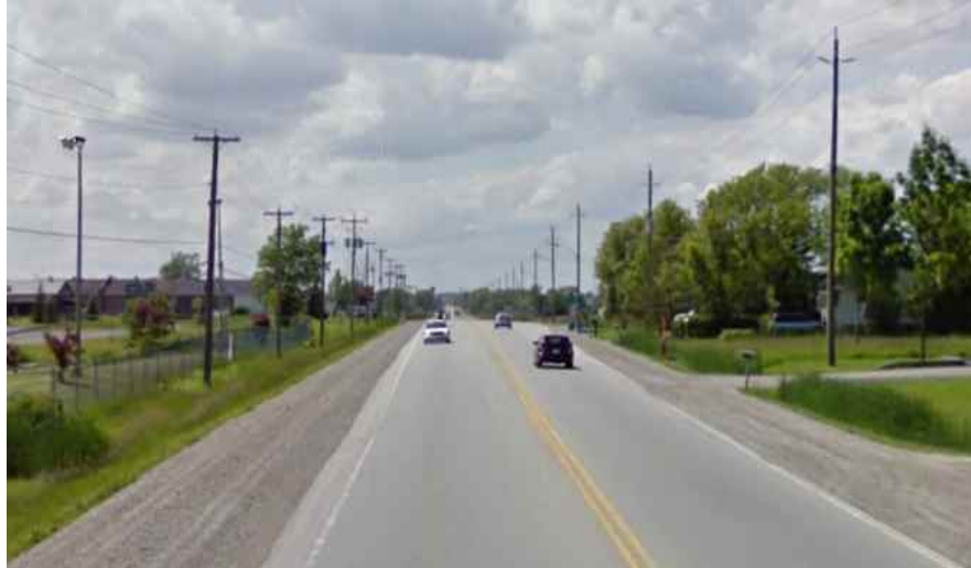
Figure 18: HONI's 8.32kV line on the south side (left) of Rymal Road paralleling Horizon Utilities' 27.6/16kV line along the north side (right).
