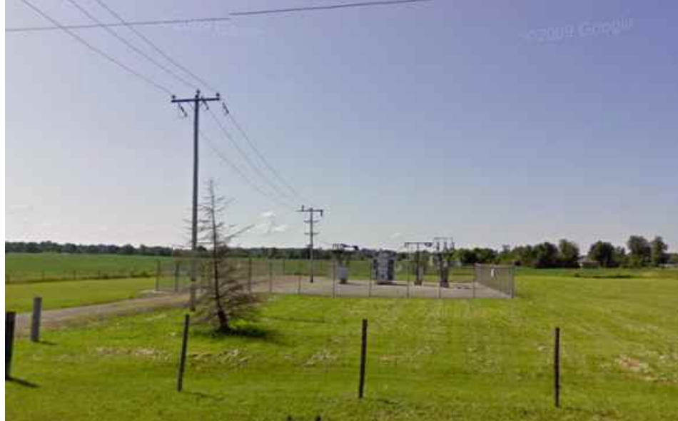
Figure 7: Dickenson DS and 27.6/16kV supply circuit
