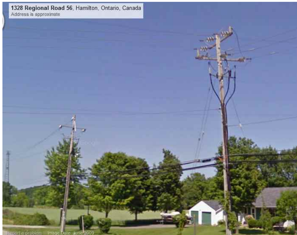
Figure 15: 8.32/4.8kV feeder reaches Highway No. 56
