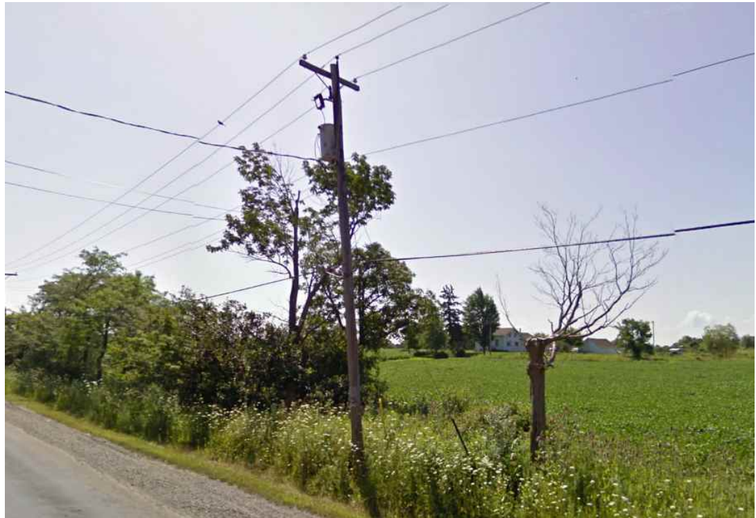
Figure 9: Rural 8.32/4.8 kV distribution system
