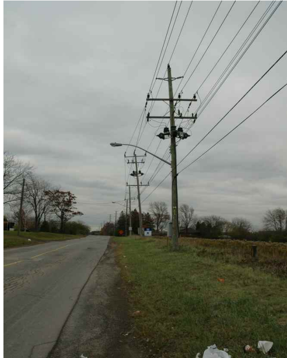
Figure 6: Demarcation point. Primary metering
