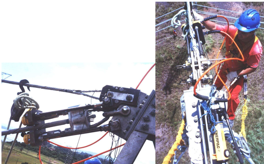
Picture # 11 – General overview Maintenance of a Cross-Rope tower
