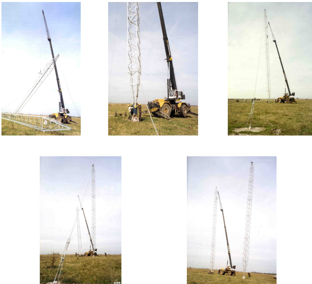
Picture # 10 – General overview of a 500 kV Cross- Rope tower field assembly
