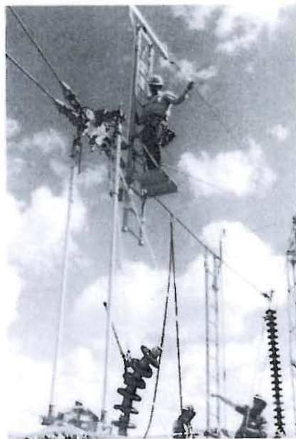
Fig. 7. Replacing the insulator string followed the reverse sequence.
