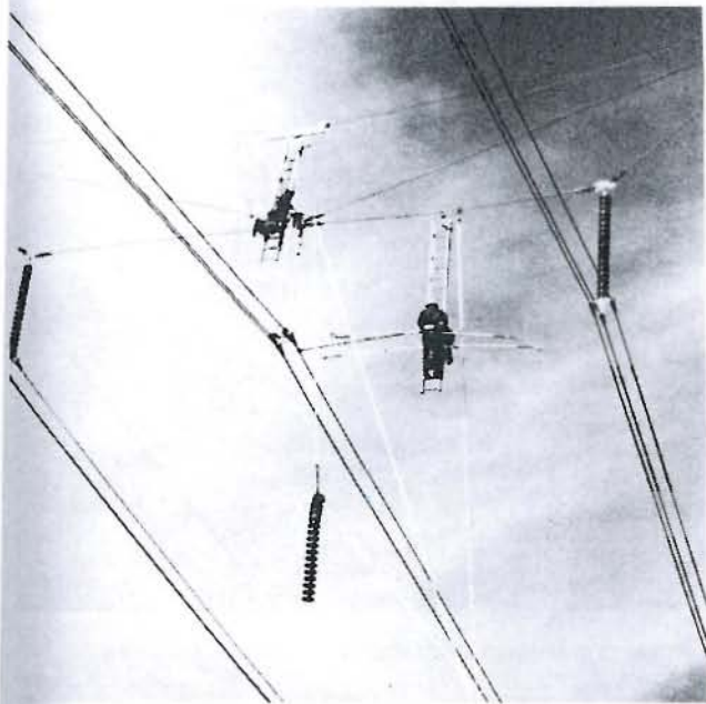
Fig. 4. A 16-ft hot stick was attached to the center phase and secured to the ladder.
