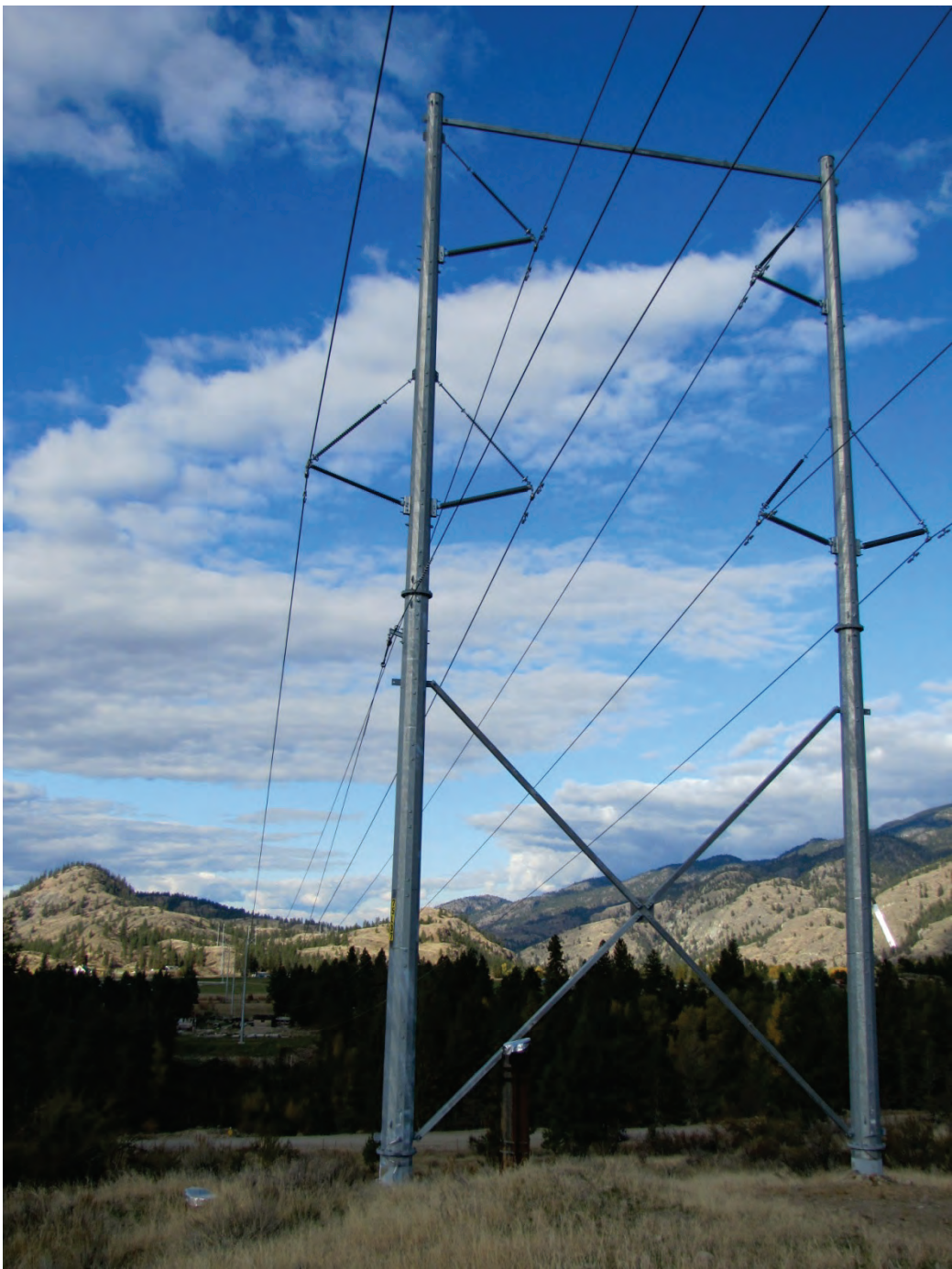
Photo 6 - 75/76 Line North from Shuttleworth Creek
