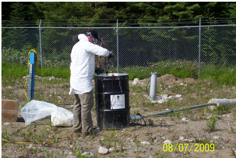
Photo 1: Preparing ORC slurry prior to pumping into amendment distribution system
