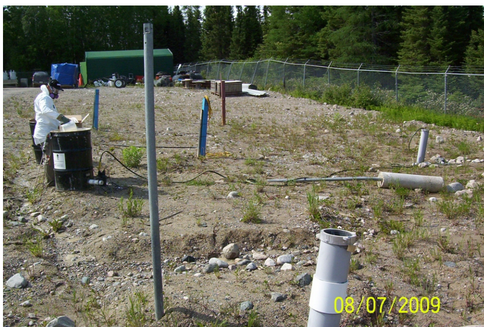
Photo 2: Pumping ORC solution into amendment distribution system
