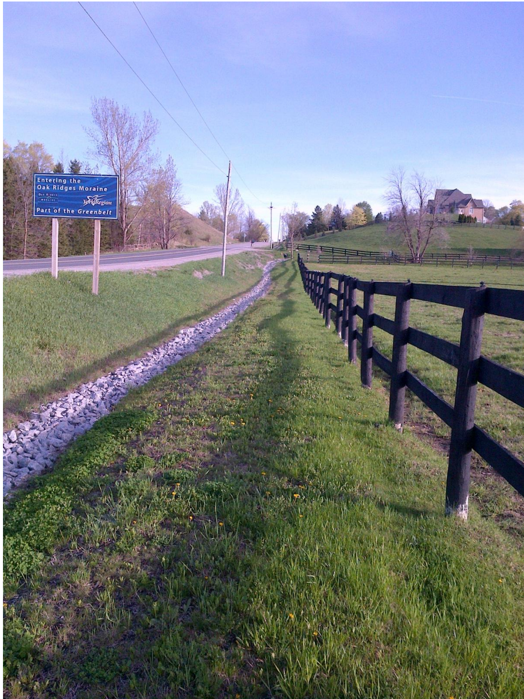
Photo 1 Steep Drainage Channel Stabilized with Rip-Rap on West Ditch of Jane St, Approaching Davis Drive (May 6, 2013)
