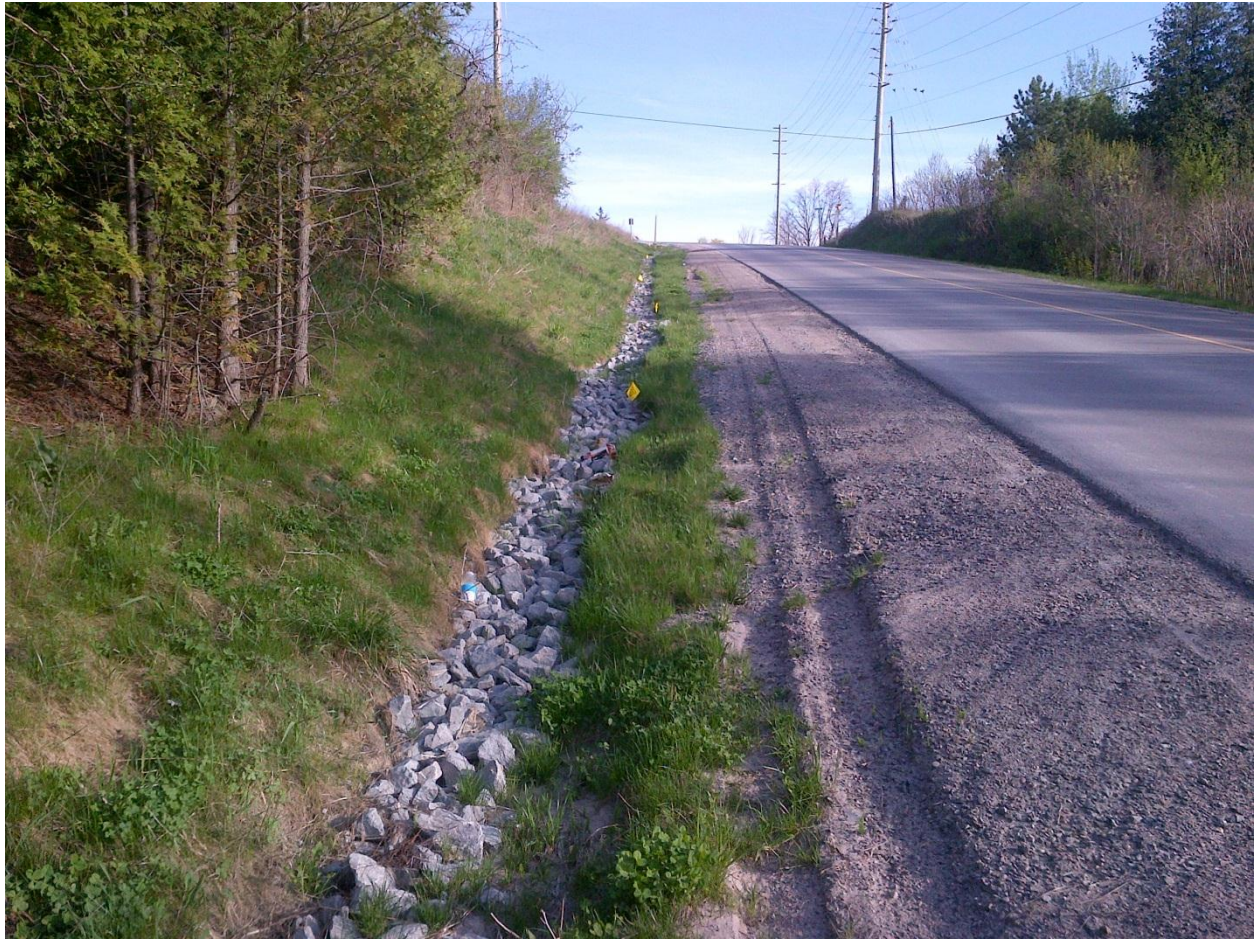
Photo 6 Rip-Rap Installed within the Drainage Ditch in 2012 on the East side of Dufferin Street, Directly North of Miller's Side Road (May 6, 2013)
