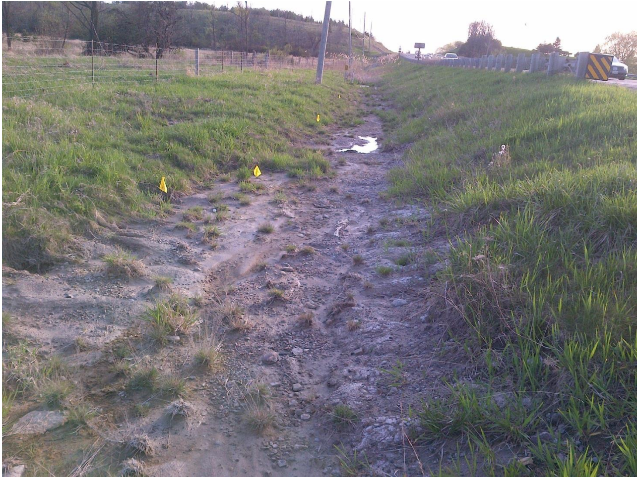
Photo 2 Drainage Ditches Leading into WC6 Remains without Full Vegetation Re-establishment (May 6, 2013)
