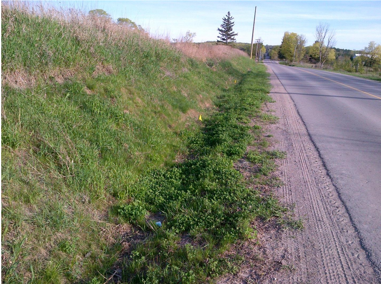
Photo 5 Slope Stability of a Former Sloughing/Soil Creep Area South of Miller's Side Road on Dufferin Street (May 6, 2013)
