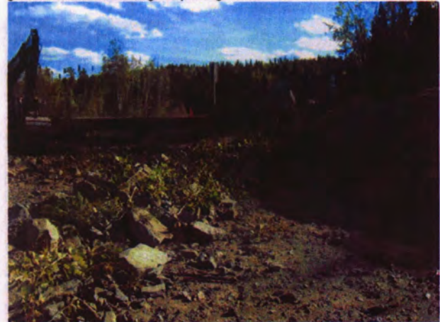
Photo 8: Migration Corridor - Woody debris was placed on the migration corridor to provide added cover. The corridor could have been constructed using any natural material, blast rock and woody debris was chosen for its availability.
