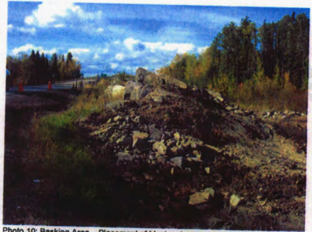
Photo 10: Basking Area - Placement of blast rock on south facing slope will provide a basking area and cover for basking snakes after emergence in the spring
