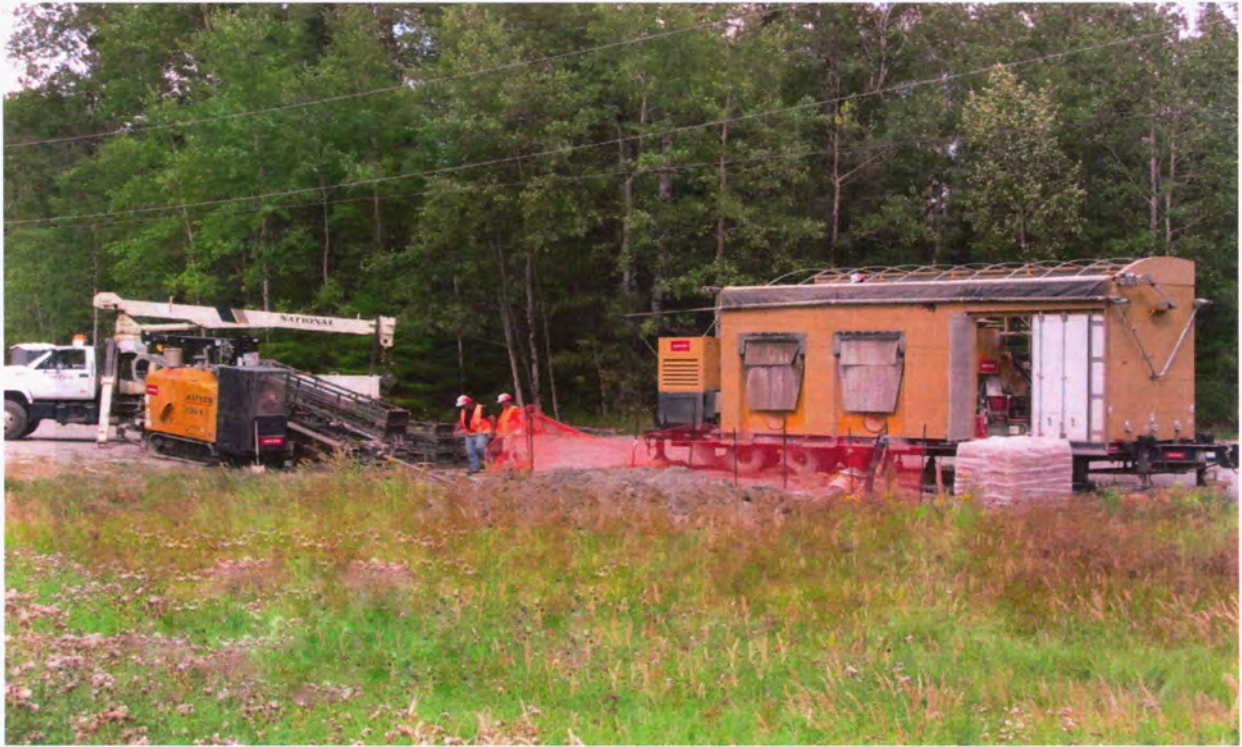
The horizontal directional drill unit, pictured to the left and the drilling mud reclaimer, pictured to the right, successfully installed 338 metres of pipe across the Chukuni River along Hwy 105. The same unit successfully installed 263 metres of pipe through solid rock at the Chukuni River located along Hwy 125.
