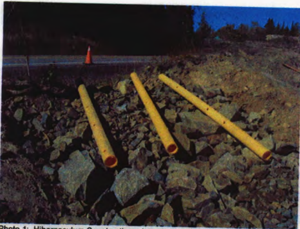
Photo 1: Hibernaculum Construction – base layer of blast rock installed with 8' – 10' sections of crush resistant piping with random holes drilled in it placed on top. The blast rock will form the void spaces of the hibernaculum with the piping providing access points to the hibernaculum.
