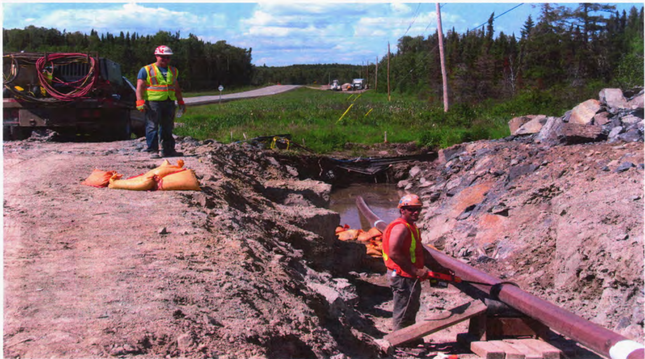
Many wet areas along the right-of-way were installed by drilling under the wetland.
