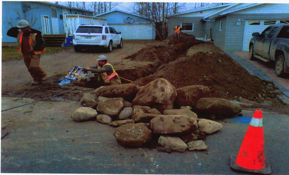
A service line is being installed to a home in the community of Balmertown.
