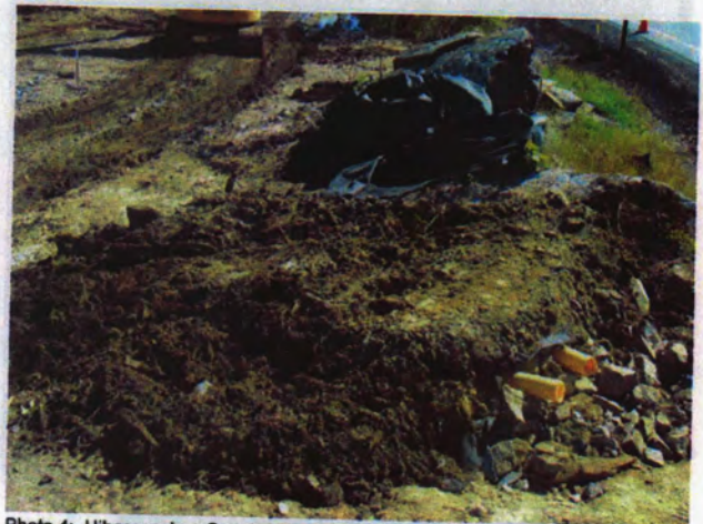
Photo 4: Hibernaculum Construction – Initial placement of soil over the hibernaculum. The soil placement is required to provide insulation to the hibernaculum to prevent complete freezing though the winter. A layer of soil approximately 1.3 m (4') is required.
