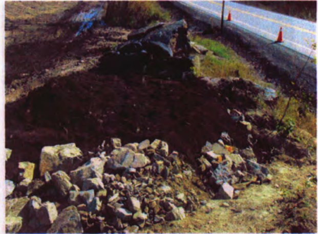
Photo 6: Hibernaculum Construction – Placement of top soil over the hibernaculum to add to the insulating layer and provide a suitable base for plant growth of the future seeding and plantings.
