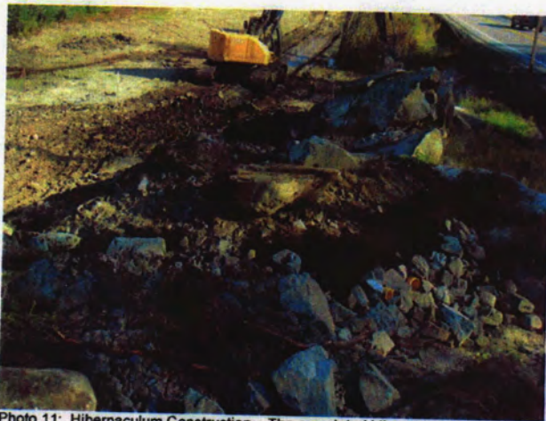
Photo 11: Hibernaculum Construction - The completed hibernaculum with boulder placements on top for add basking area, cover and visual improvement. Entrance pipes can be covered by blast rock to improve visual aspects but must remain clear of smaller debris which could block access to the hibernaculum.
