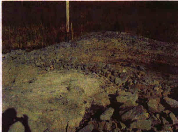
Photo 7: Migration Corridor - Installation of the blast rock which forms the structure of the migration corridor for snakes moving to and from the hibernaculum. The corridor will provide cover for snake movement prior to the re-vegetation of the gas line corridor.
