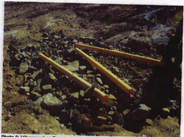
Photo 2: Hibernaculum Construction – Crush resistant piping arranged for placement of the top layer of crush rock, which will finish the interior construction of the hibernaculum.
