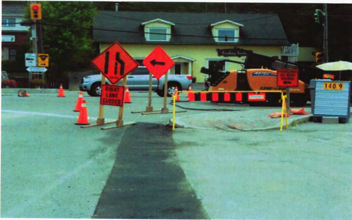
Pipelines were installed by excavation (trench backfilled and pavement patched in foreground) and by trenchless technology (horizontal directional drill in background).
