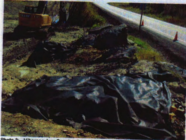
Photo 3: Hibernaculum Construction – Access piping completely encased with blast rock and covered with geotextile ready for the placement of soil. The geotextile will prevent the void spaces from infilling with soil.
