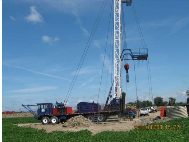
Service Rig Over a Well
