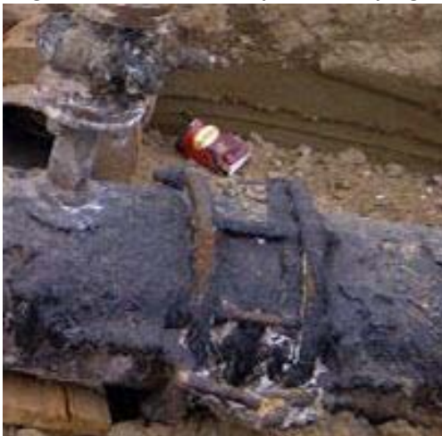
Figure 2: Unrestrained Compression Coupling
