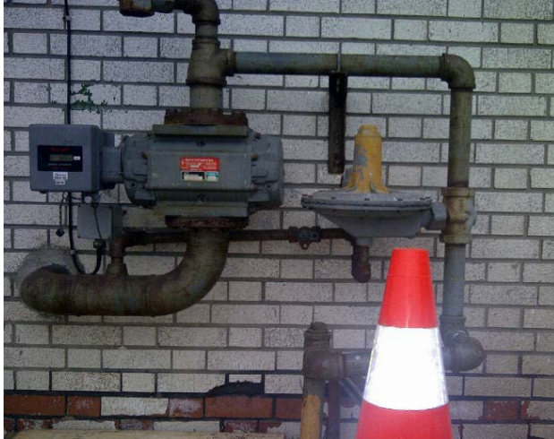
Figure 1: Typical CLR Rotary Meter Set with Single Regulator
