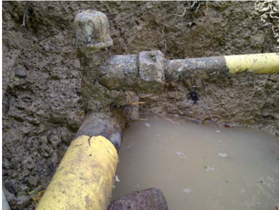
Figure 1: Compression Outlet Service Tee installed Figure 2: Compression Outlet Service Tee
