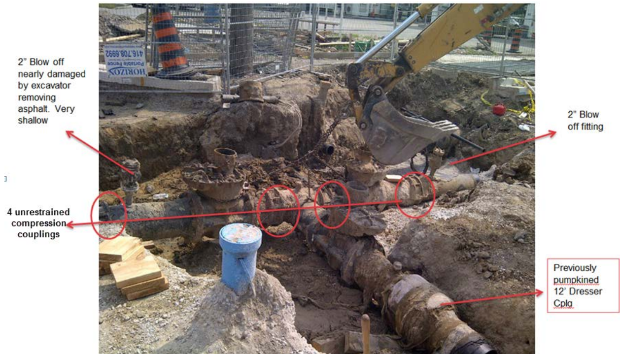
Figure 4: Construction reveals compression couplings at Martin Grove & Burnhamthorpe Rd
