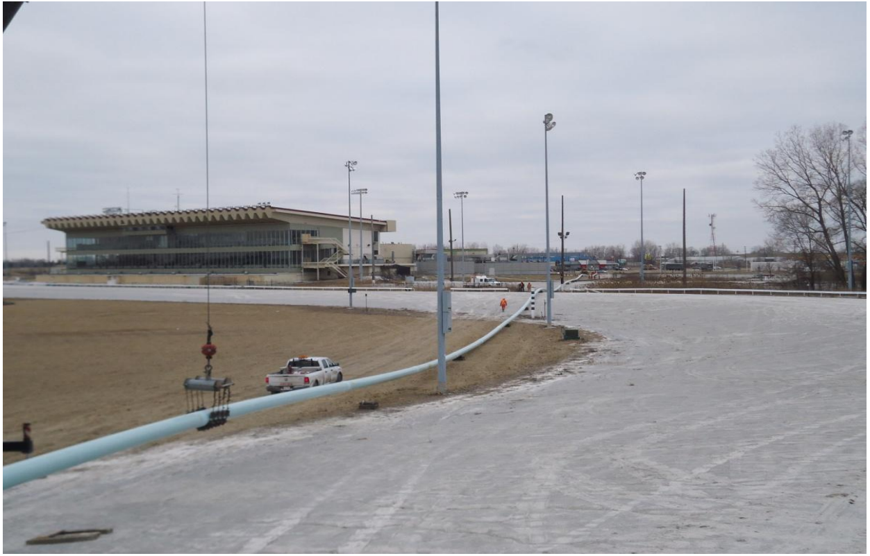
The pipe was stung out across the race track property, welded together and pulled into place as one section.
