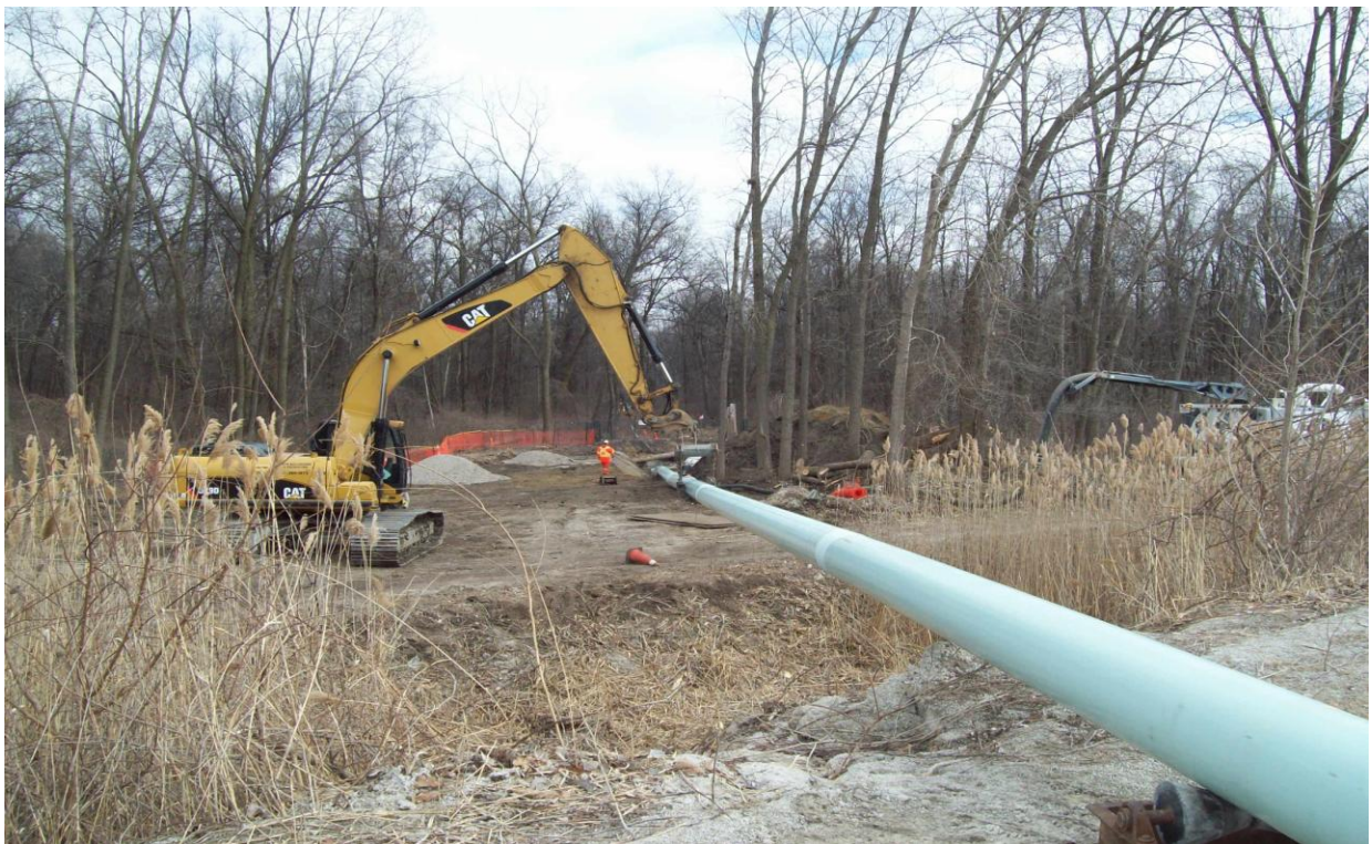
During installation the pipe is placed on rollers located both on the ground as well as attached to machinery. This allows for a smooth motion during the pulling process.
