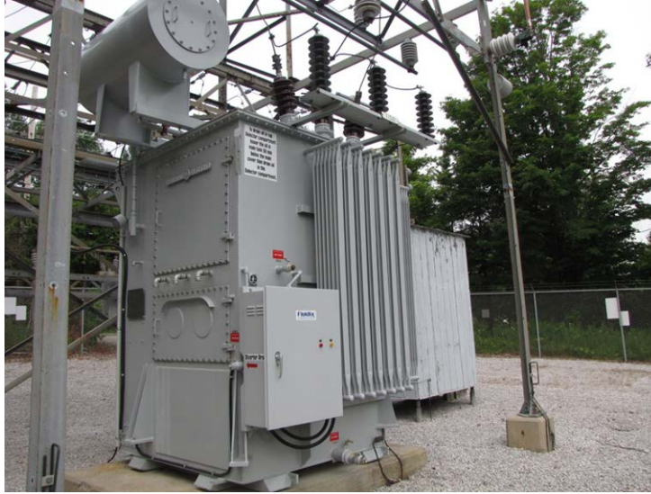
Figure 1: Picture of a Station Transformer
