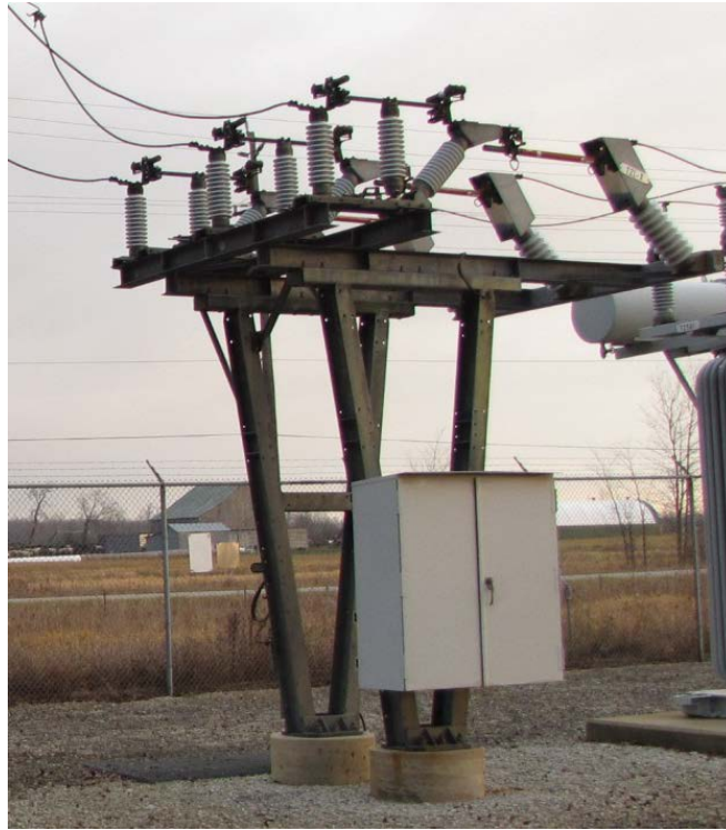
Figure 7: Picture of a Station Switch and Fuse Combination
