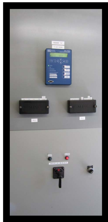
Figure 5: West Feeder Replacement Multifunction Protection Relay
