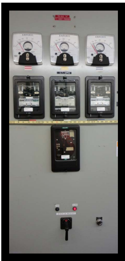
Figure 4: West Feeder Original Single Function Electromechanical Relays
