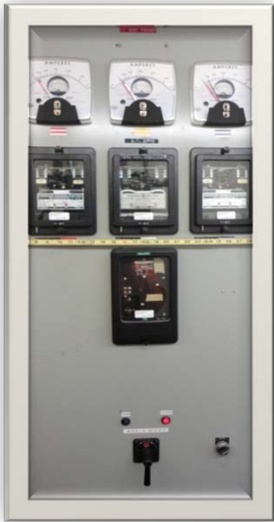
Figure 2: West Feeder Original Single Function Electromechanical Relays
