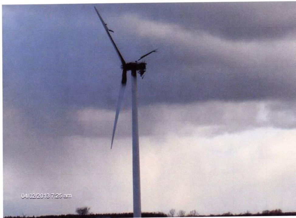
Scorched wind turbine near Goderich on April 2, 2013. Contributed photo
