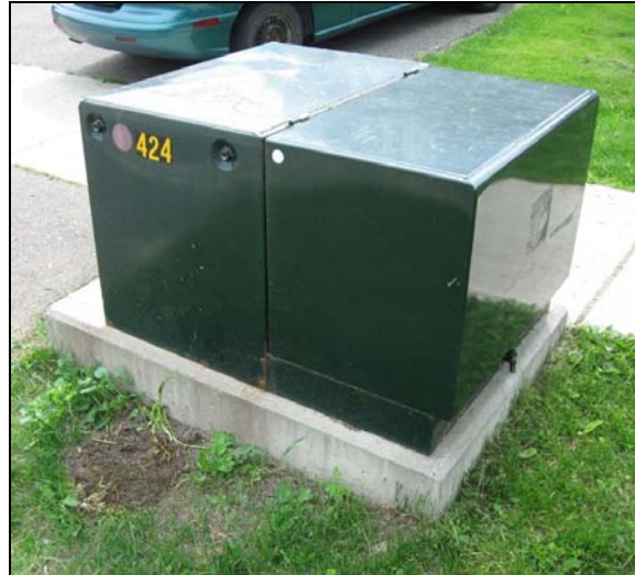
Picture – Pad Mounted Transformer
