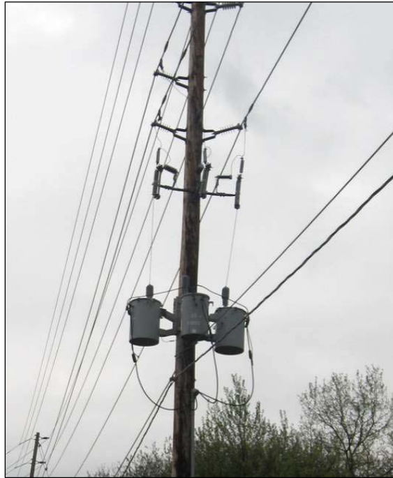
Picture - Pole Mounted Transformers
