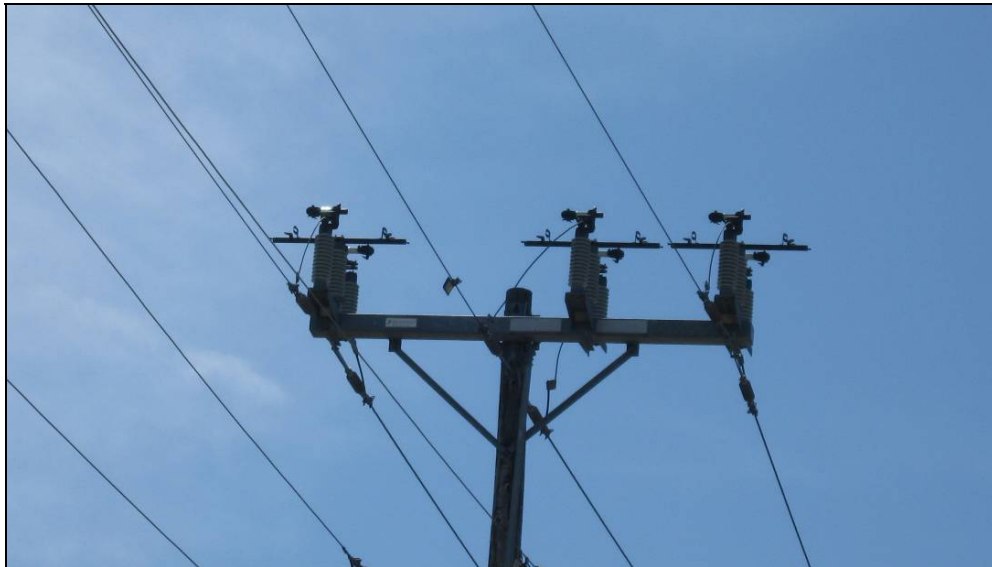
Picture: Pole Top Load Break Switch
