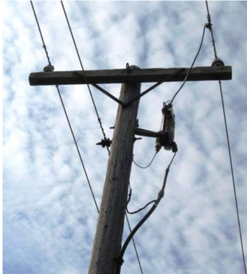
Riser Pole from section 3.1.7
