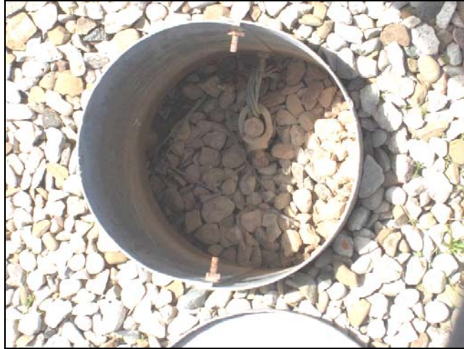
Picture - Station Ground Rod
