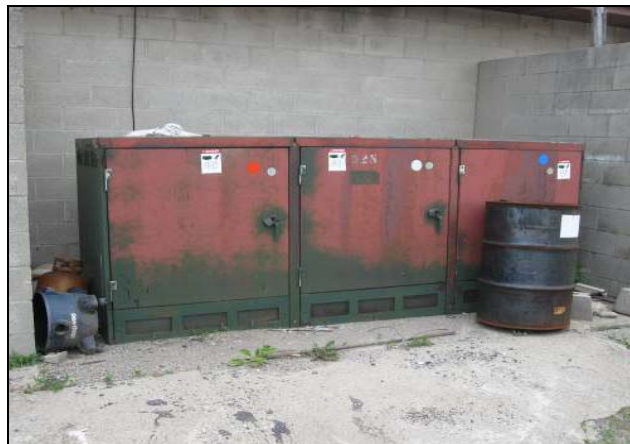
Picture – Transpad Transformer
