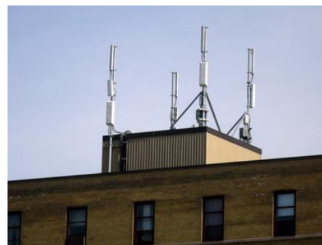
Figure 17 - Macro Cell site on rooftop
