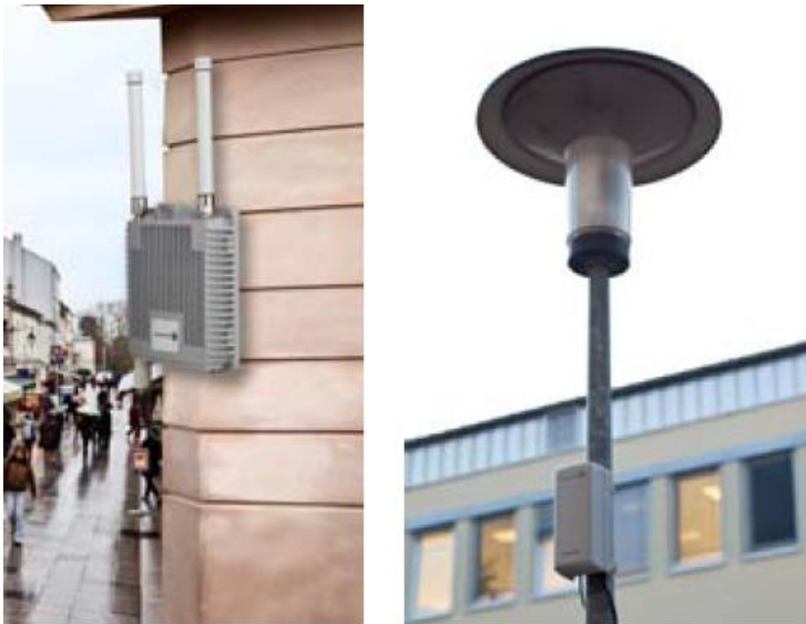
Figure 20 - Images of various attachment options for small cell equipment
