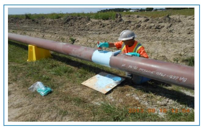
When the sandblasting of the joint is complete, the area is protected using an epoxy coating which will dry very hard. The coating is then inspected to ensure the thickness is consistent with company standards.
