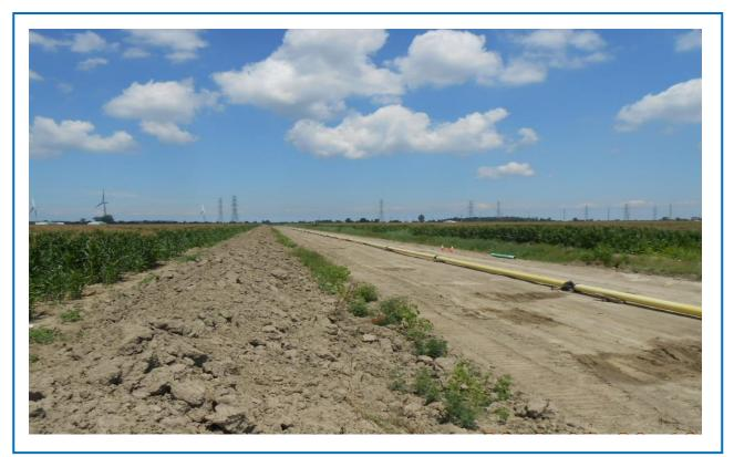
Upon completion of the topsoil stripping, the pipe is strung out along the easement to be welded together.
