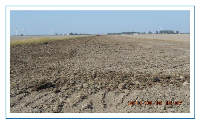
Following backfilling, the topsoil is replaced and the area was cultivated to relieve residual compaction.
