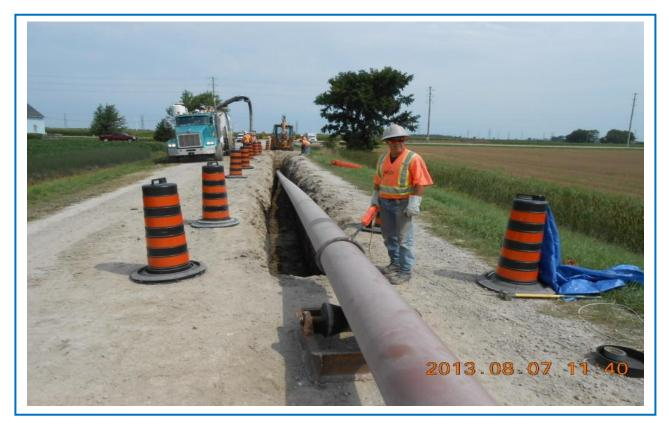
Prior to lowering of the pipe into the trench or while pulling the pipeline during a directional drilling operation, the pipe is "jeeped". An electrically charges spring is wrapped around the pipe and can detect minute flaws in the coating. When detected, the flaws are immediately repaired.
