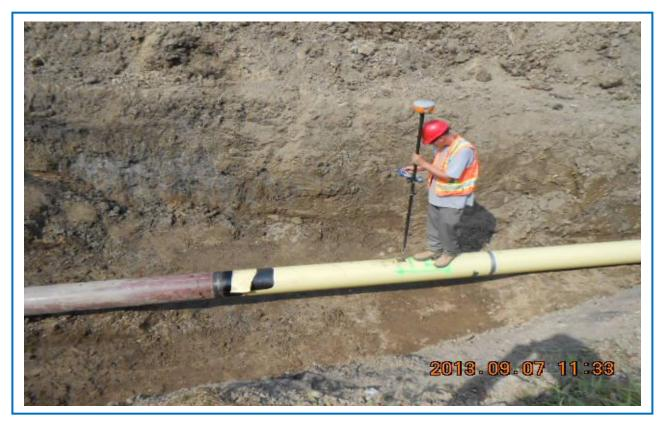
Following the installation of each pipeline section, the pipe is surveyed along its length to ensure accurate records are maintained.
