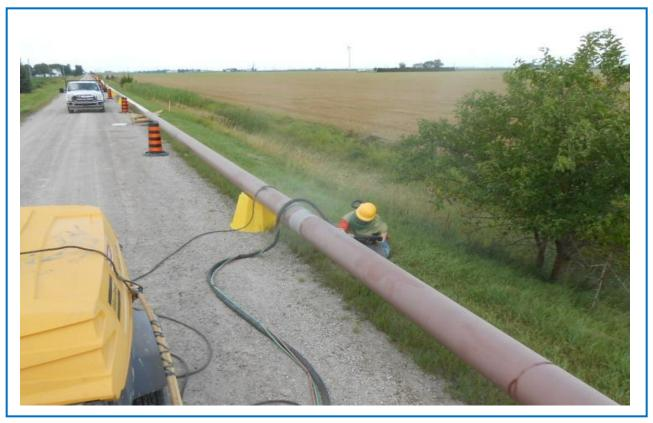
After two sections of pipe have been welded together, the area is sand blasted to remove any impurities and rust. For safety, the worker must wear protective clothing and a helmet with a separate air supply.
