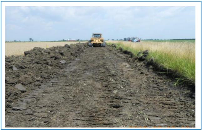
Measurements are taken to distinguish between topsoil and subsoil. A dozer is then used to perform the operation of separating the two layers.
