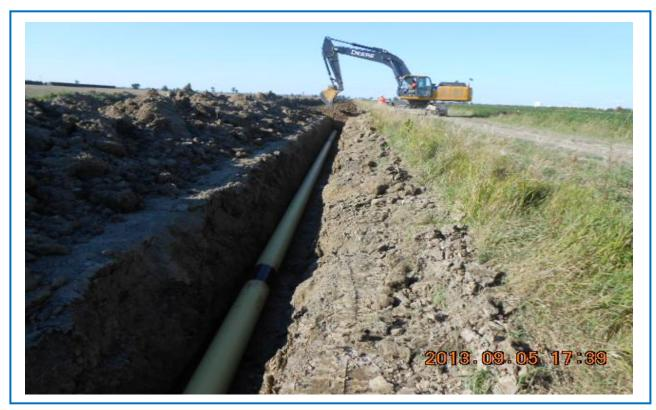
Once the pipeline has been installed the trench is backfilled using an excavator.
