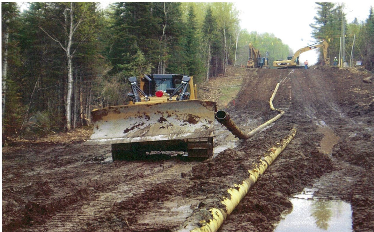
Prior to installing the new NPS 12 inch pipeline the existing NPS 10 pipeline was removed. Once the pipeline is removed, the trench is backfilled and the area is prepared for the installation of the new pipeline. Although conditions were wet, construction continues as work is taking place in an area with no agricultural potential.
