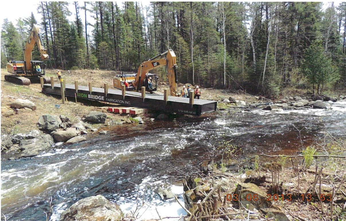
One of the first activities of construction is to install temporary vehicle accesses across watercourses. Above a bridge is being installed across Ferguson Creek.
