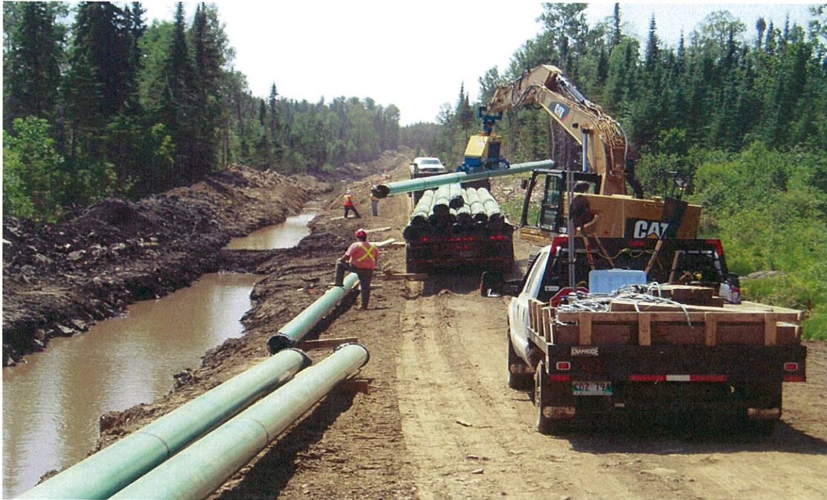
The new NPS 12 inch pipeline is being off loaded and strung along the pipeline easement. Prior to installing the pipe, water is removed from the trench and is discharged through a filtration device before its release into the surrounding environment.
