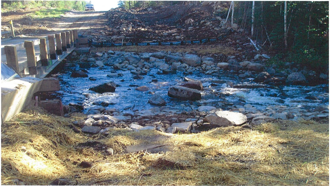
Ferguson Creek following the installation of the pipeline. The creek bed was capped with large rock to resemble pre construction conditions.
