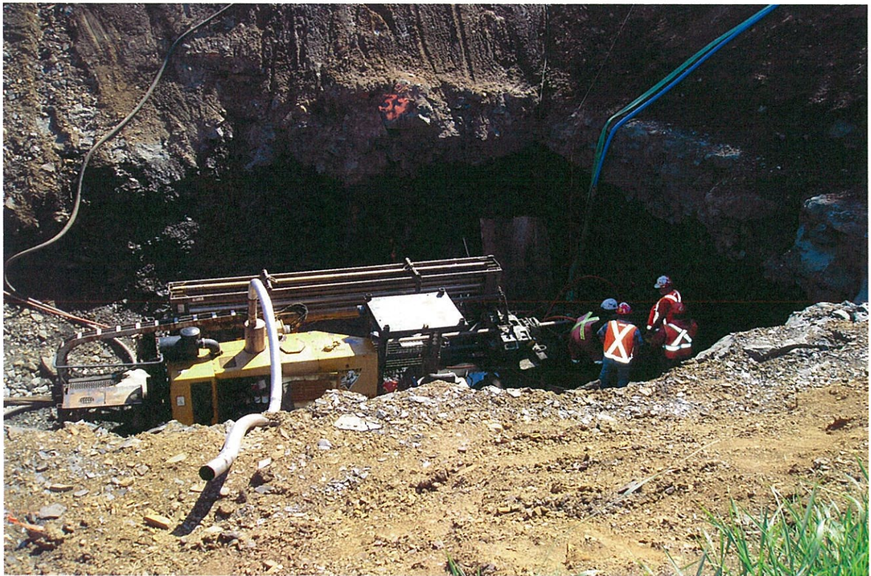
The McIntyre River and John Street crossings were proposed to be crossed by open cut. After further investigation by Union and its Contractor the crossings were completed by horizontal bore.
