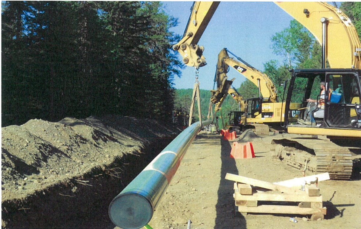
The new NPS 12 inch pipeline is being off loaded and strung along the pipeline easement. Prior to installing the pipe, water is removed from the trench and is discharged through a filtration device before its release into the surrounding environment.
