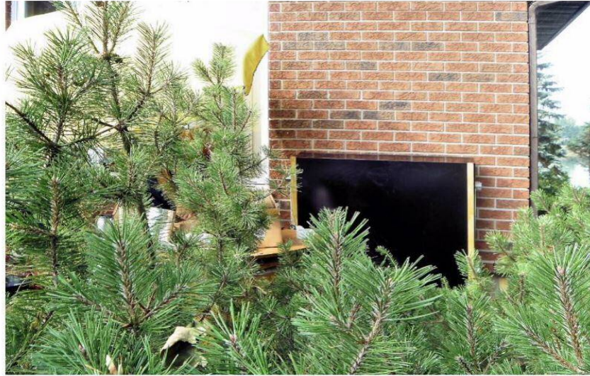
Figure 4. Air-heat exchanger. The 50 kW air-heat exchanger transfers heat into the ground loop of the test-bed system.
