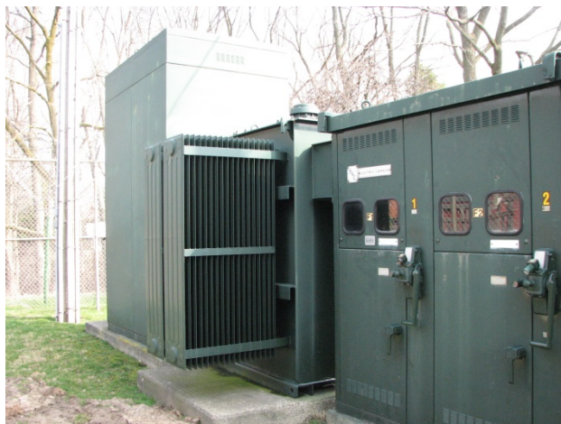
Substation Transformer
