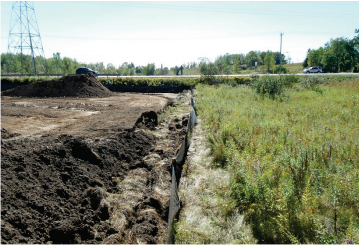
Photo 1: September 18 – East side of Highway 6; perimeter silt fencing along northern workspace limit as viewed facing west
