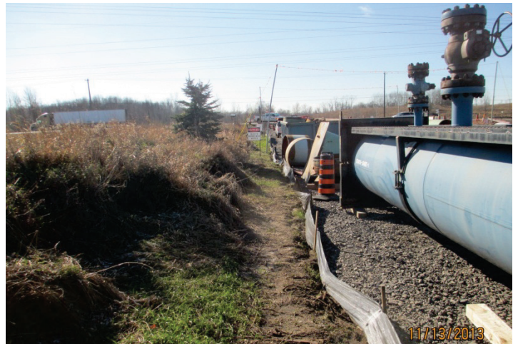
Photo 6: November 13 – East side of Highway 6; perimeter silt fencing along the southern workspace limit as viewed facing west
