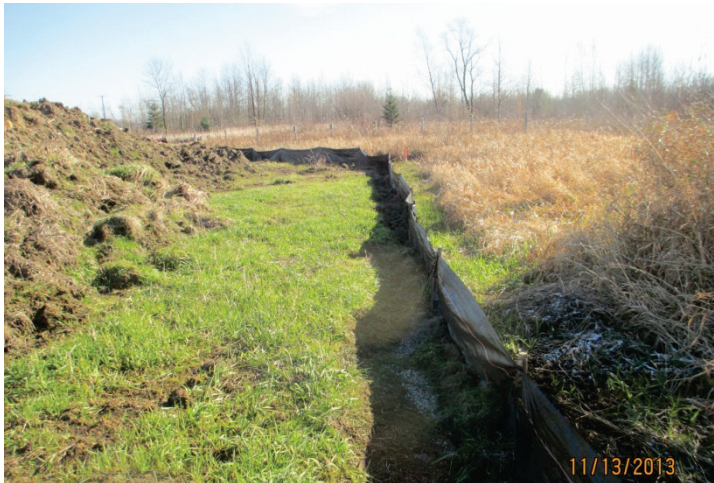
Photo 10: November 13 – West side of Highway 6; perimeter silt fencing along the northern workspace limit as viewed facing east.
