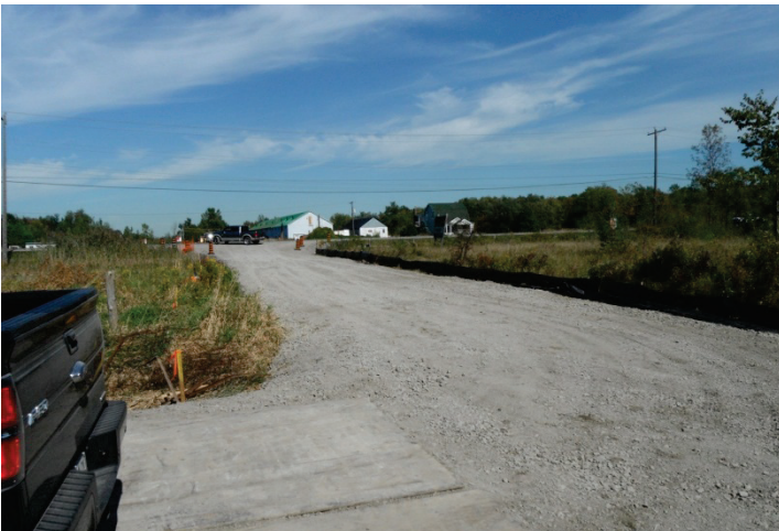
Photo 5: November 13 - West side of Highway 6; perimeter silt fencing along the southern workspace limit as viewed facing east
