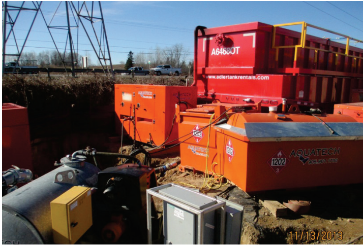
Photo 8: November 13 – Sediment settling tank and equipment used for de-watering and filtering sediment prior to water discharge to the natural environment
