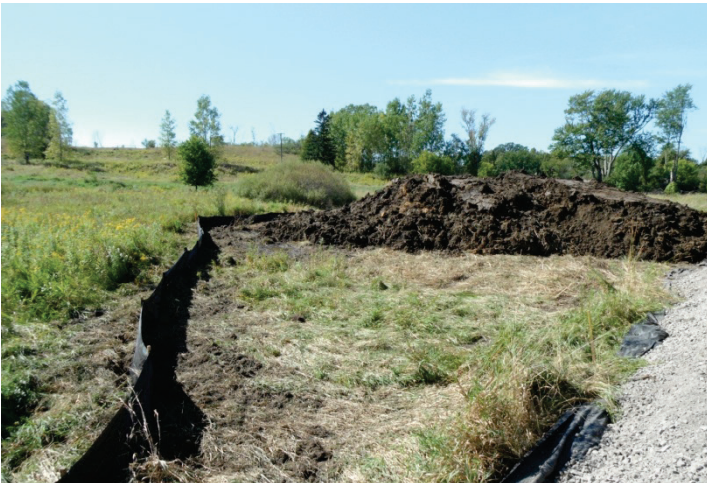
Photo 3: September 18 – West side of Highway 6; perimeter silt fencing along western workspace limit as viewed facing north
