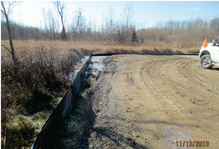
Photo 9: November 13 – West side of Highway 6; perimeter silt fencing on the southern workspace limit as viewed facing east
