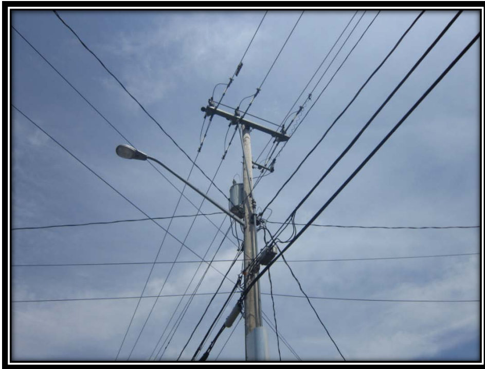
Complex Primary Pole - Considerable Attachment including air break switch, transformer, street light, third party telecommunication attachments, secondary conductor and guying.
