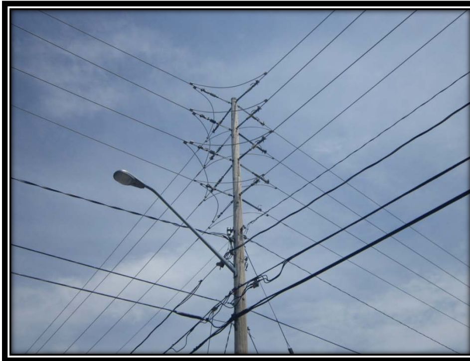
Complex Primary Pole to Replace - Considerable attachments including two separate three phase circuits, street light, third party telecommunication attachments, secondary conductor and guying.
