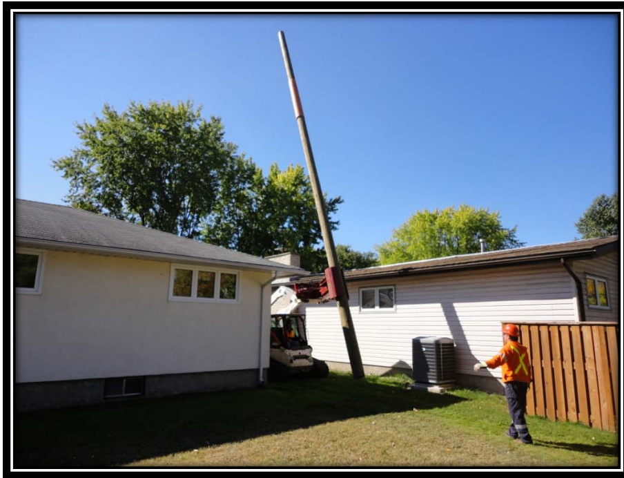
Poor Accessibility - Back Lot Construction requiring use of "Pole Claw"
