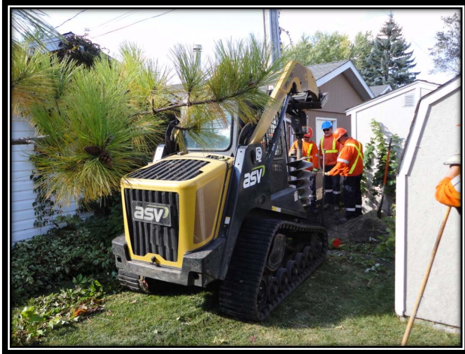
Poor Accessibility - Back Lot Construction requiring use of Bob Cat Auger
