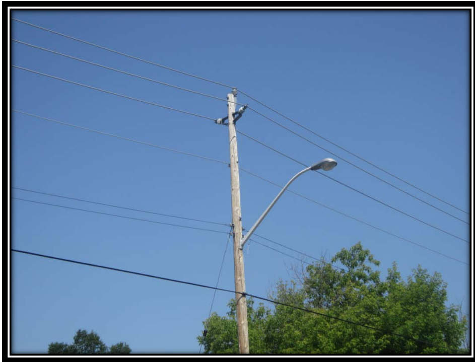
Standard Primary Pole - Attachments include primary three phase circuit, street light, third party telecommunication attachments, secondary conductor and guying
