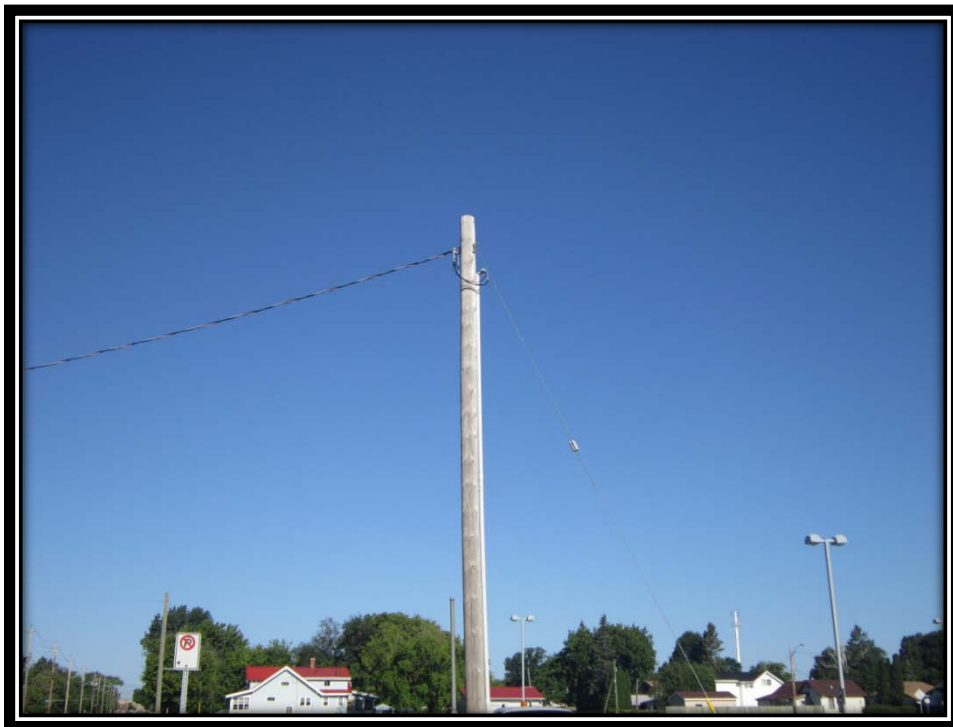
Basic Secondary Pole - Accessible secondary pole with only two attachments including secondary conductor and down guy.
