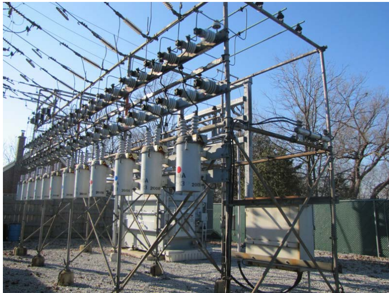
Figure 6: Picture of Station Reclosers
