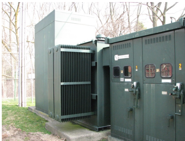
Substation Transformer
