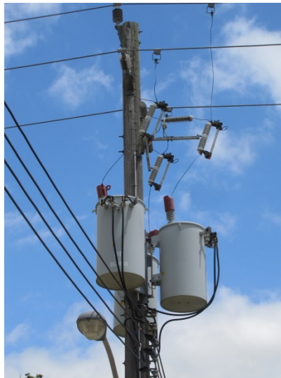
Pole-mount Transformers
