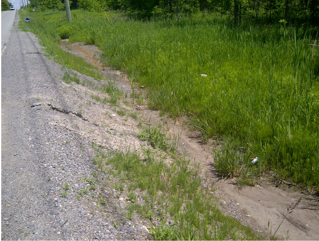
Photo 9: Approx. 40m east of 1898 Baseline Road on the south side
