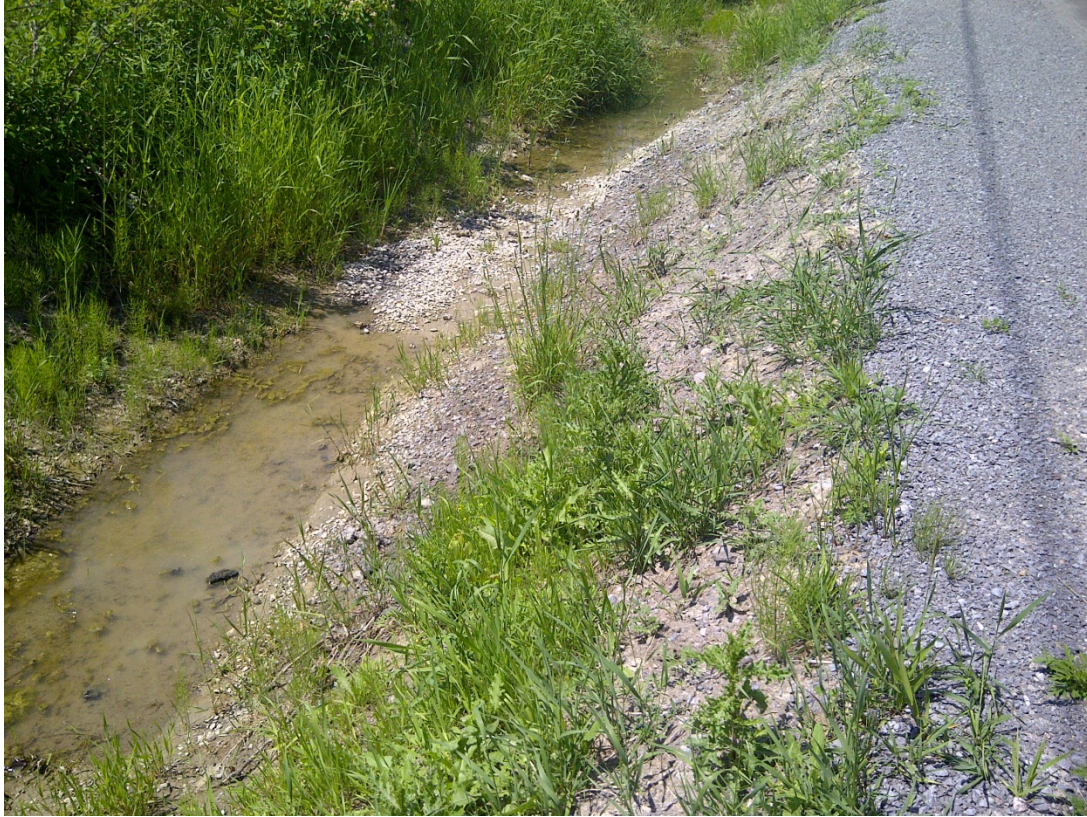
Photo 15: Approx. 180m north of 1387 Solina Road
