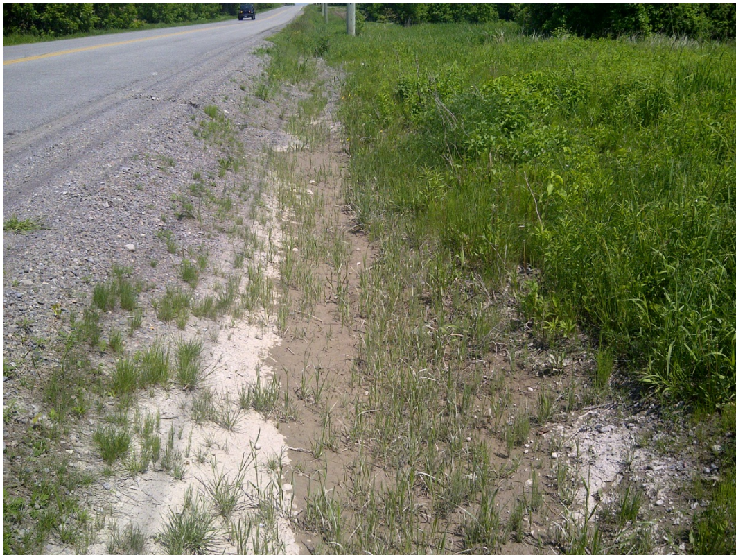
Photo 10: Approx. 150m east of 1898 Baseline Road on the south side
