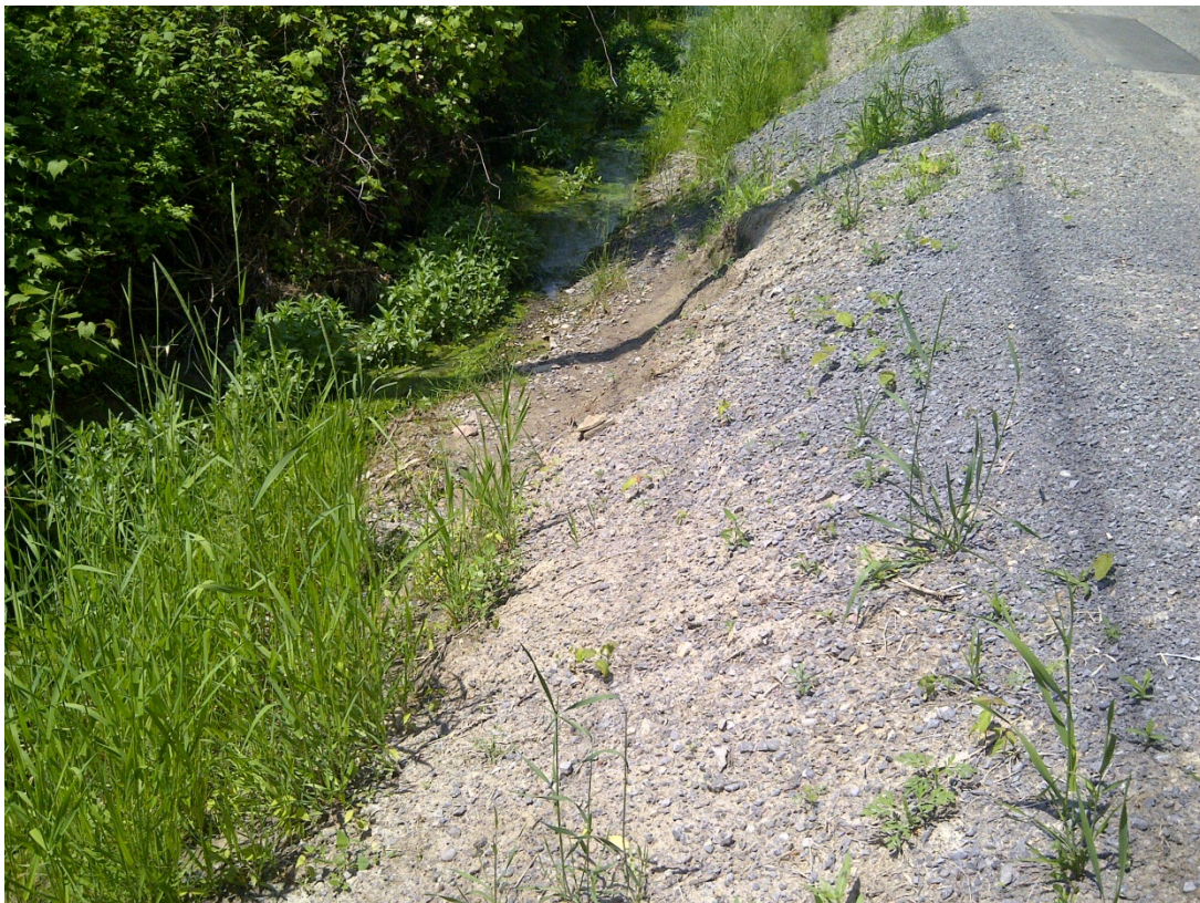
Photo 14: Approx. 150m north of 1387 Solina Road
