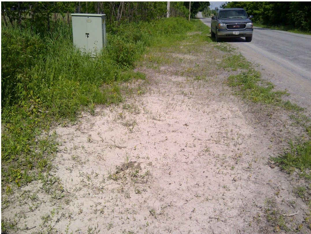
Photo 20: North East corner and East side of Old Scugog Road at Concession Road 4
