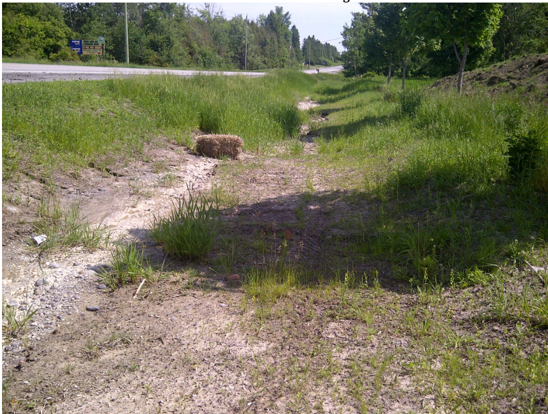
Photo 22: Approx. 200m south of Concession Road 4 on Regional Road 57
