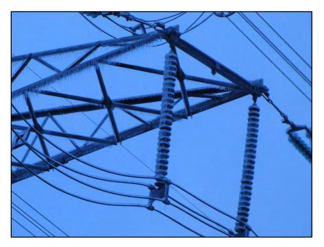
Insulators for a 500 kV transmission circuit in the GTA that is covered in ice.
