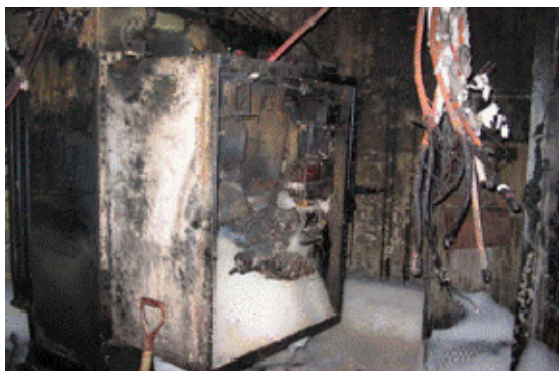
Figure 36: Damaged network unit and burned AILC cables. (March 24, 2007)
