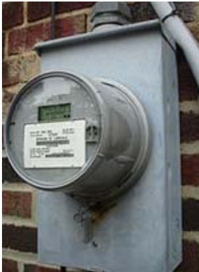
Figure 57: Smart meter installation at customer location.
