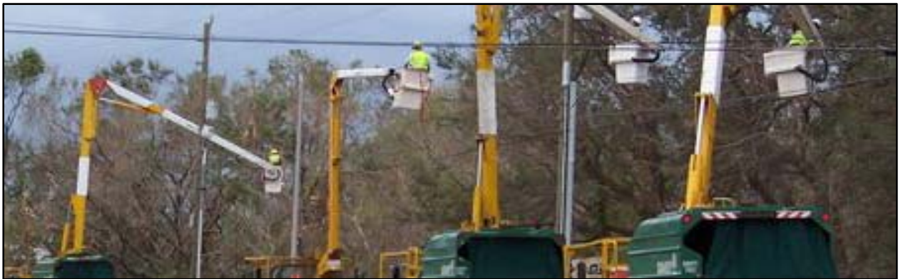
Figure 20: Tree Trimming of an Overhead Feeder
