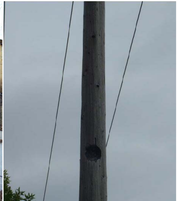
Figure 6: Woodpecker hole on a pole
