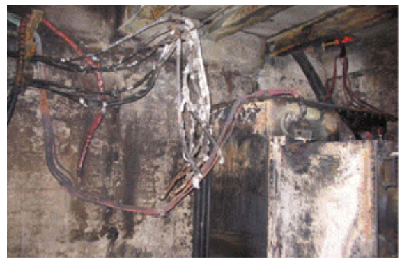
Figure 36: Damaged network unit and burned AILC cables. (March 24, 2007)
