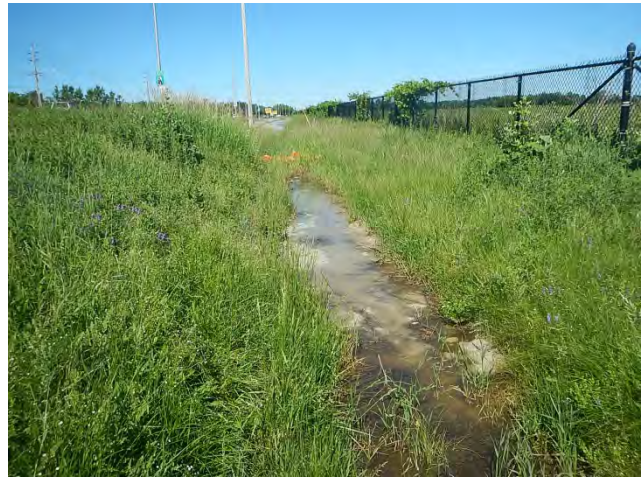
Photo 22: Spill with remnant material on West Hunt Club Road. Note sandbag isolation measures in background.
