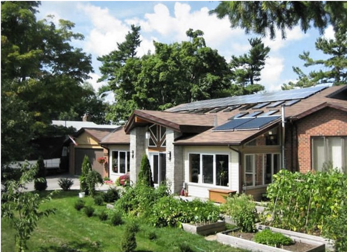
Figure 4 The "testbed" system. The store is buried under the lawn (six boreholes, 20 metres deep). The air-heat collector is behind the bushes on the right. The heat pump is in the basement. A pair of solar collectors is mounted on the roof (lower right).
