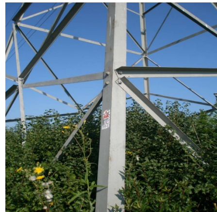
Figure 35C: Steel Tower Recoated
