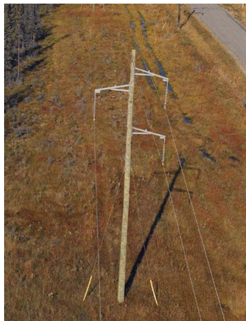
Figure 29B: Wishbone Structure
