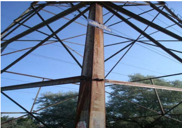
Figure 35B: Steel Tower with Corrosion
