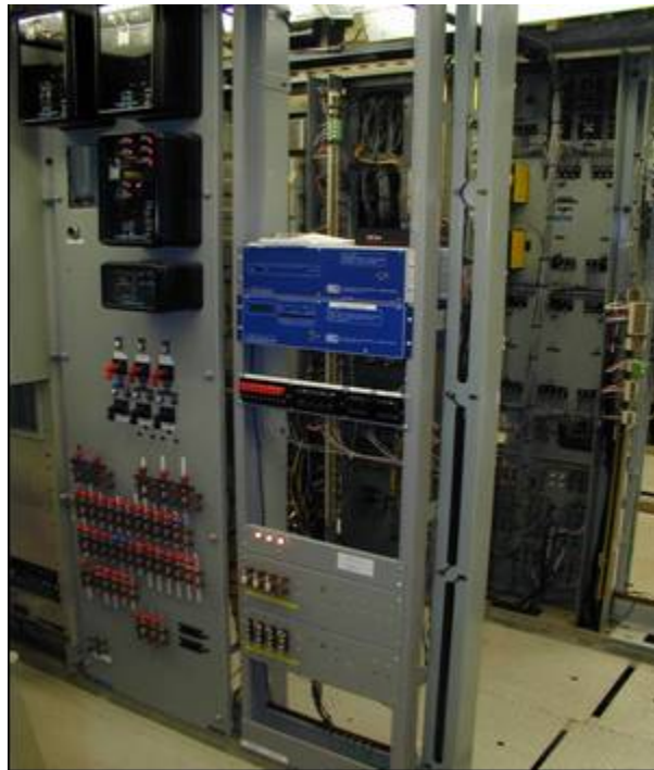
Figure 17C: Microprocessor Based Protection Scheme
