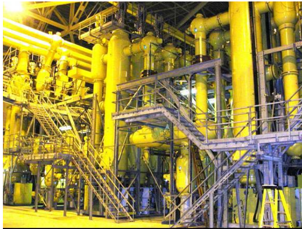
Figure 11E: 500kV GIS Circuit Breakers
