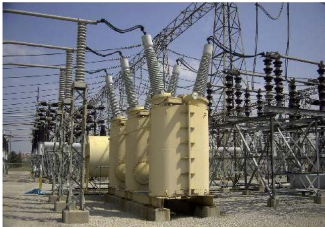
Figure 11A: Oil Circuit Breaker
