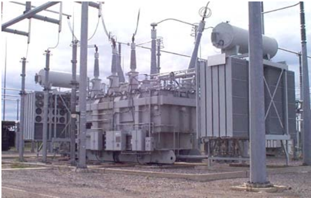
Figure 6: 500/230 kV Autotransformer
