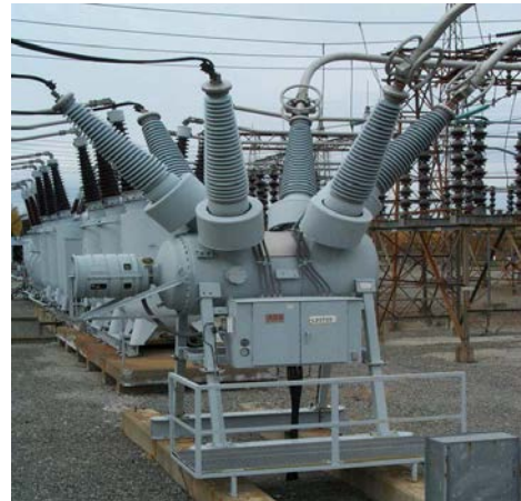
Figure 11B: SF6 Circuit Breaker
