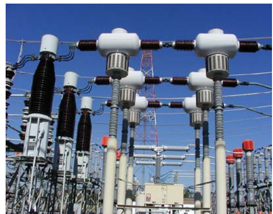
Figure 11D: Air Blast Circuit Breakers
