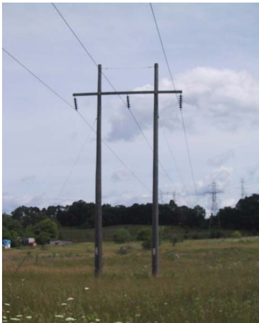
16 17 Figure 29A: Wood Pole H-Frame Structure
