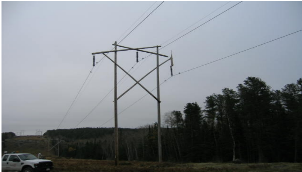
Figure 29C: 230 kV Gulfport Structure (with defective/failed cross-arm)
