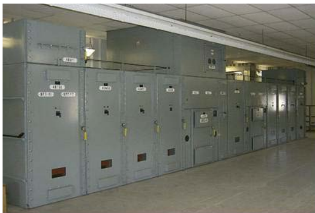
Figure 11C: Metalclad Circuit Breakers
