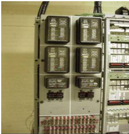
Figure 17A: Electromechanical Relay Panel
