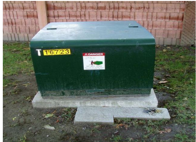
Pad mounted transformer
