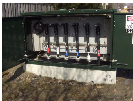
SF 6 Pad mounted switch
