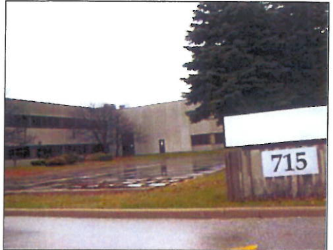
Subject viewed from driveway off Milner
