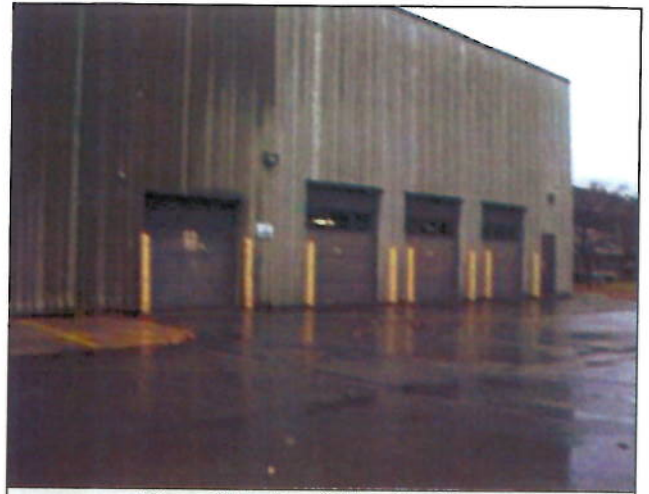
Rear shipping (drive-in doors
