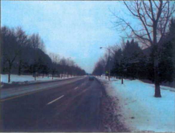
VIEW EAST ALONG MILNER ROAD
