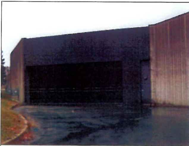
Trucking doors off Milner (exit)
