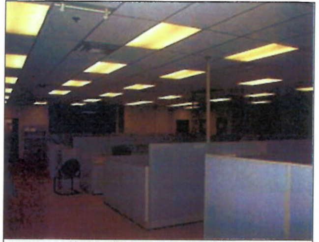
Open office area - second floor
