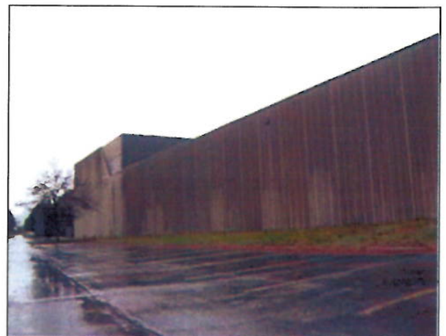
Rear view of Subject (40' and 23' height)
