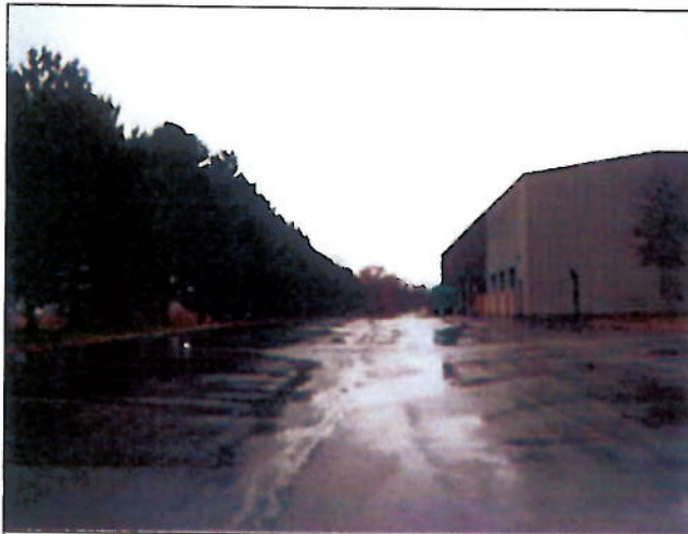
View along rear of Subject (401 to left)
