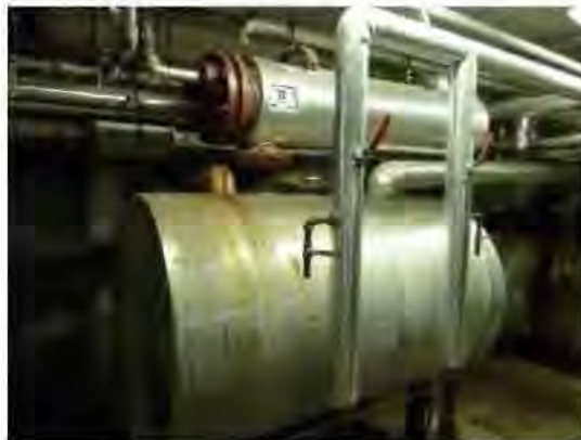
CR Flash Steam/Process Hot Water Heat Exchanger
