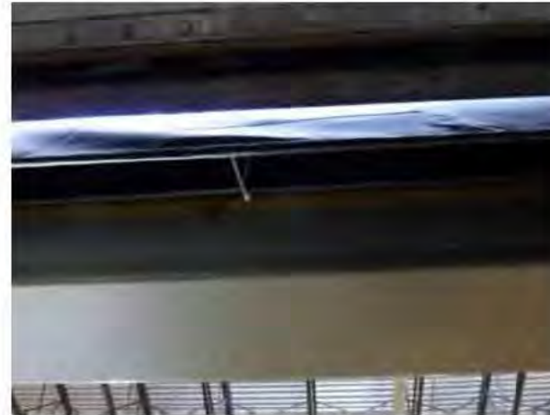
Example of top seal gap at dock
