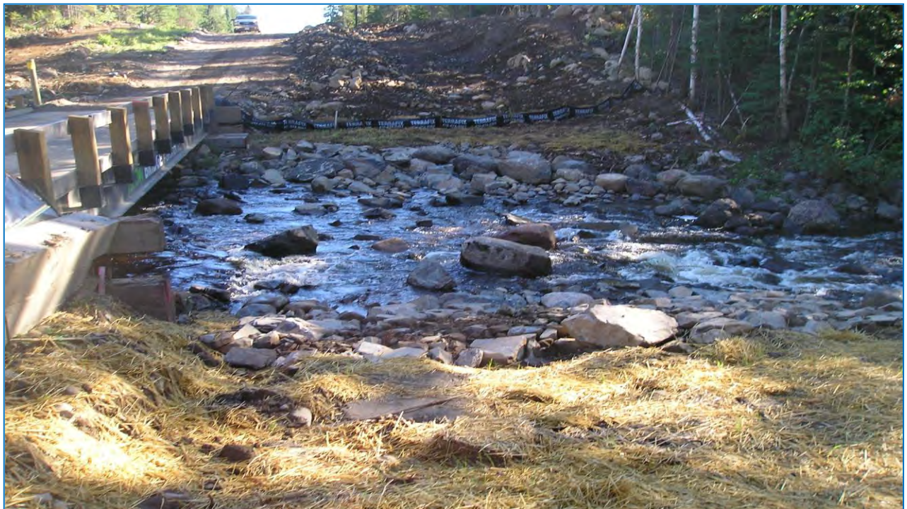
Ferguson Creek following the installation of the pipeline. The creek bed was capped with large rock to resemble pre-construction conditions.
