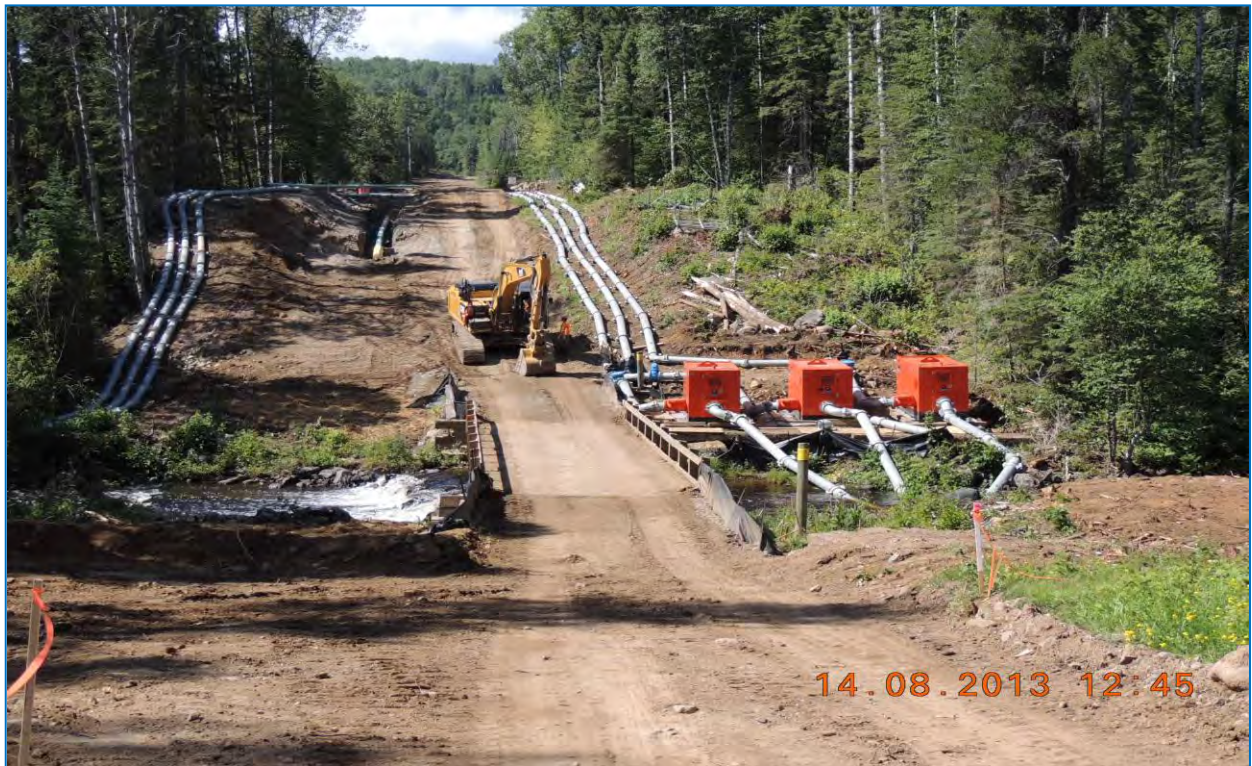
Ferguson Creek was completed using a dam & pump crossing method. Water flow is maintained by pumping the water around the construction area and discharging flow back into the watercourse downstream of the construction site.
