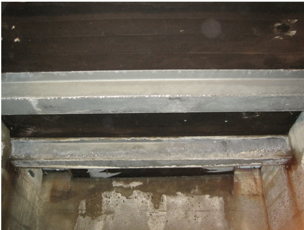
Figure 2-6 A Beam (Roof) with Life Grade Score “B”
