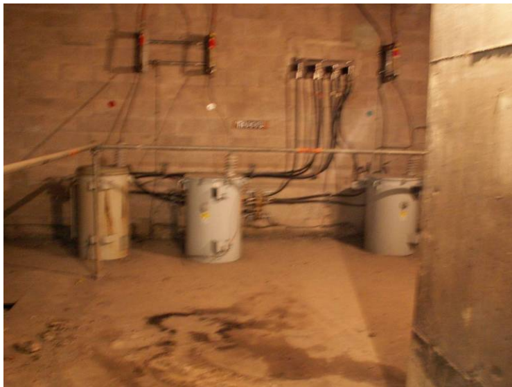
Figure 4-36 Example Building Vault Transformer
