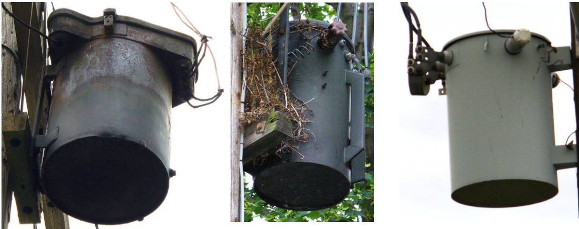
Figure 4-30 Example Pole Mounted Transformers
