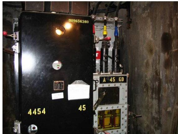
Figure 4-16 Example Transformer/Protector Units
