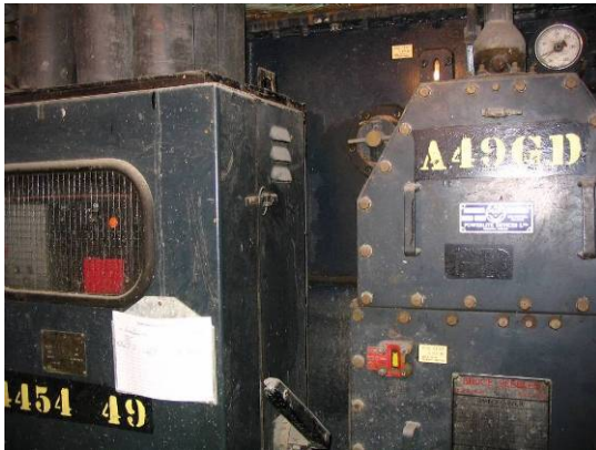
Figure 4-16 Example Transformer/Protector Units
