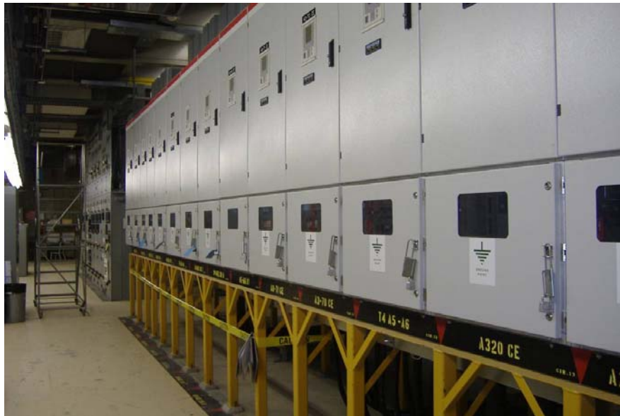
Figure 4-6 Example 13.8 kV Switchgear
