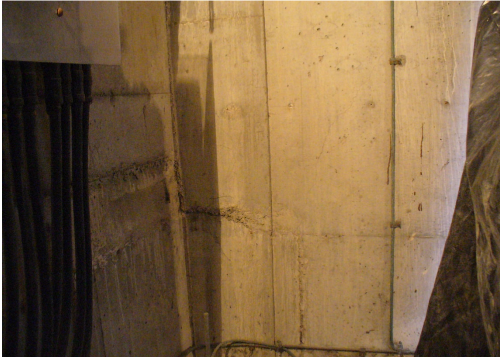
Figure 2-3 A Wall with Life Grade Score "C"
