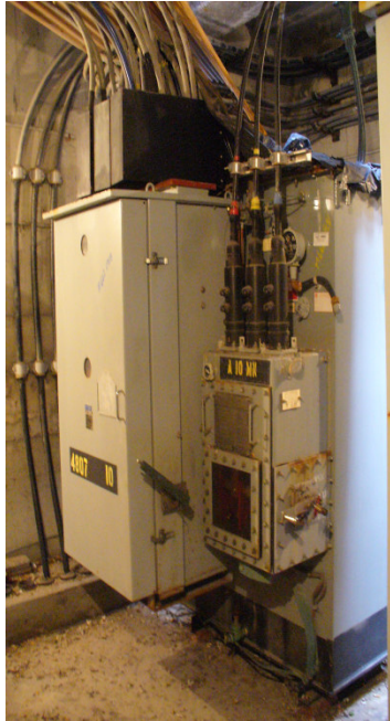
Figure 4-3 A Network Protector with Life Grade Score “C”
