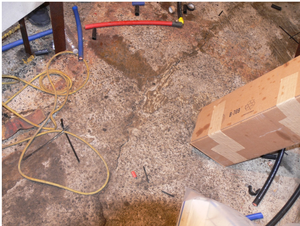
Figure 2-8 A Bottom Slab (Floor) with Life Grade Score "D"
