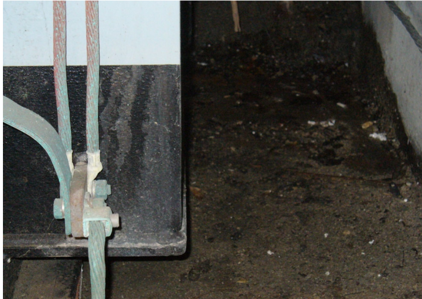
Figure 3-2 A Transformer with Life Grade Score "B"
