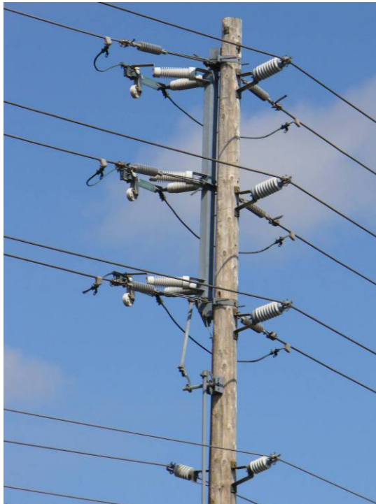
Figure 4-22 Example Manual Overhead Switch
