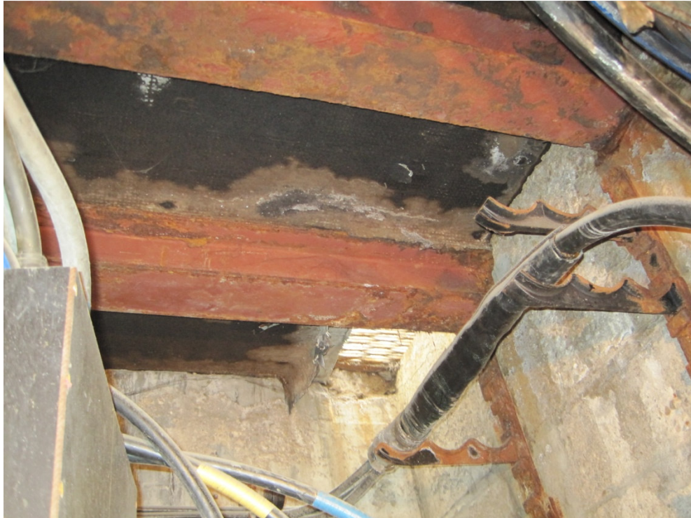
Figure 2-7 A Beam (Roof) with Life Grade Score "C"
