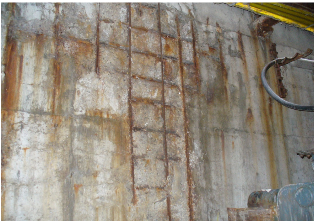
Figure 2-4 A Wall with Life Grade Score "D"
