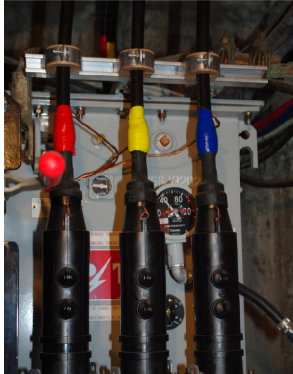
Figure 3-1 A Transformer with Life Grade Score "A"
