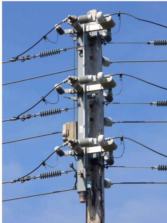
Figure 4-20 Example Remotely Operated Overhead Switch
