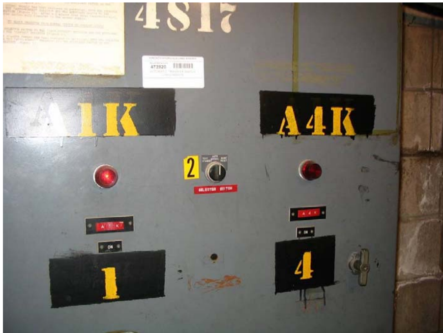
Figure 4-26 Example Auto Transfer Switch
