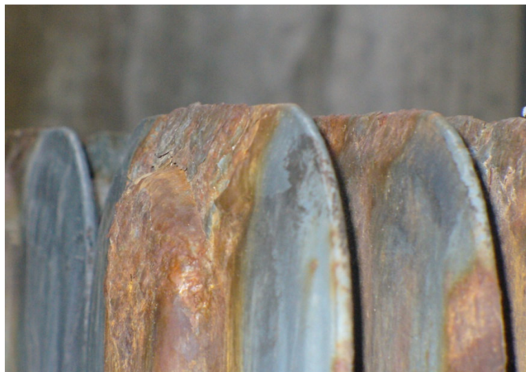
Figure 3-4 A Transformer with Life Grade Score "D"
