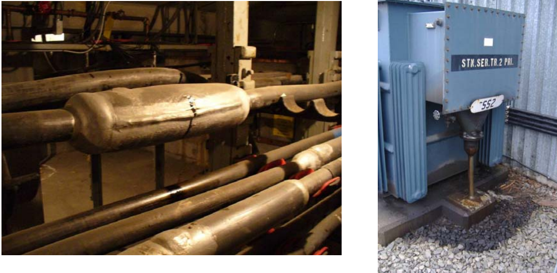
Figure 4-42 Examples of Oil Leaks
