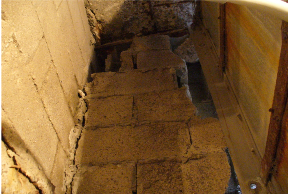
Figure 2-5 A Wall with Life Grade Score “E”
