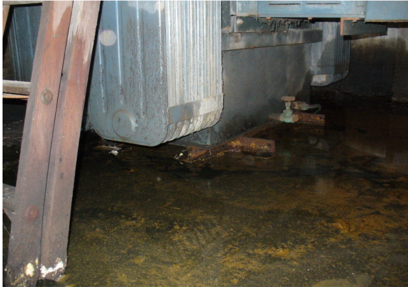
Figure 3-5 A Transformer with Life Grade Score “E”
