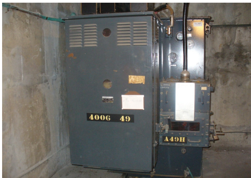
Figure 4-2 A Network Protector with Life Grade Score "B"
