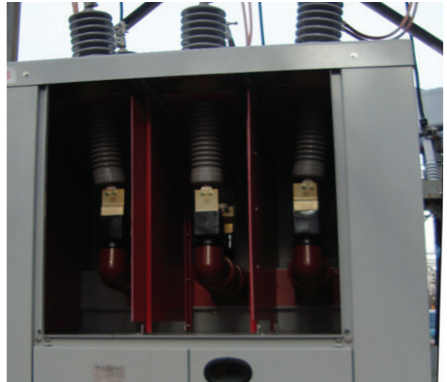
New standard outdoor vacuum circuit breaker.
