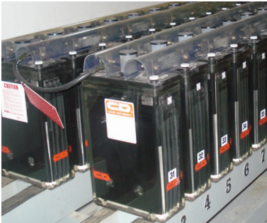
Legacy battery type requiring replacement. Batteries have a typical useful life of 10 years. Ref: E6.19, p. 8.
