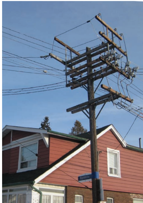
Pictured left: Box construction pole prior to conversion. Pictured right: The same pole after conversion to standard 13.8 kV configuration.
