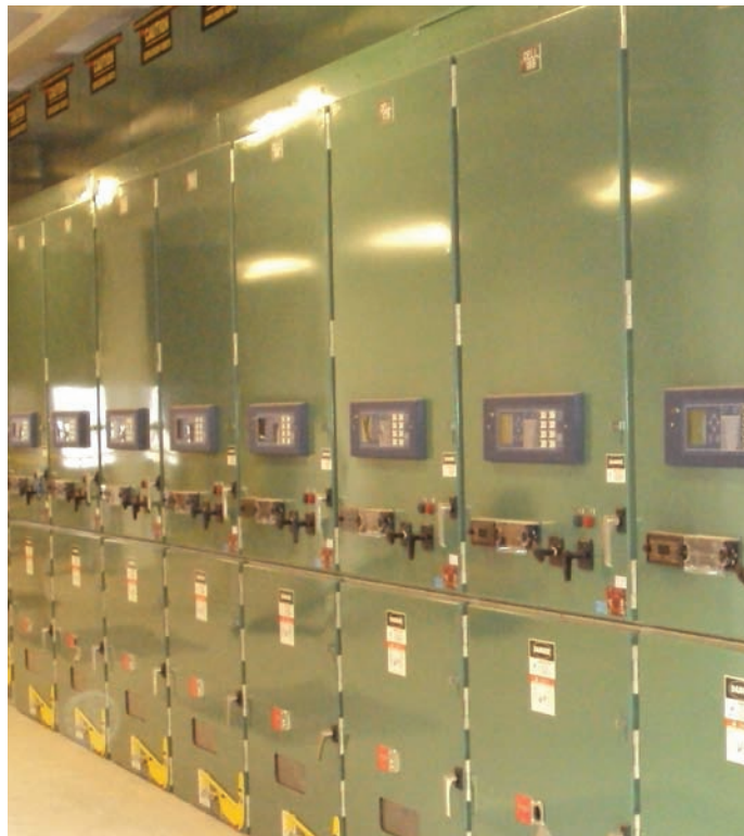
New type C arc-resistant metal-clad switchgear with vacuum circuit breakers.
