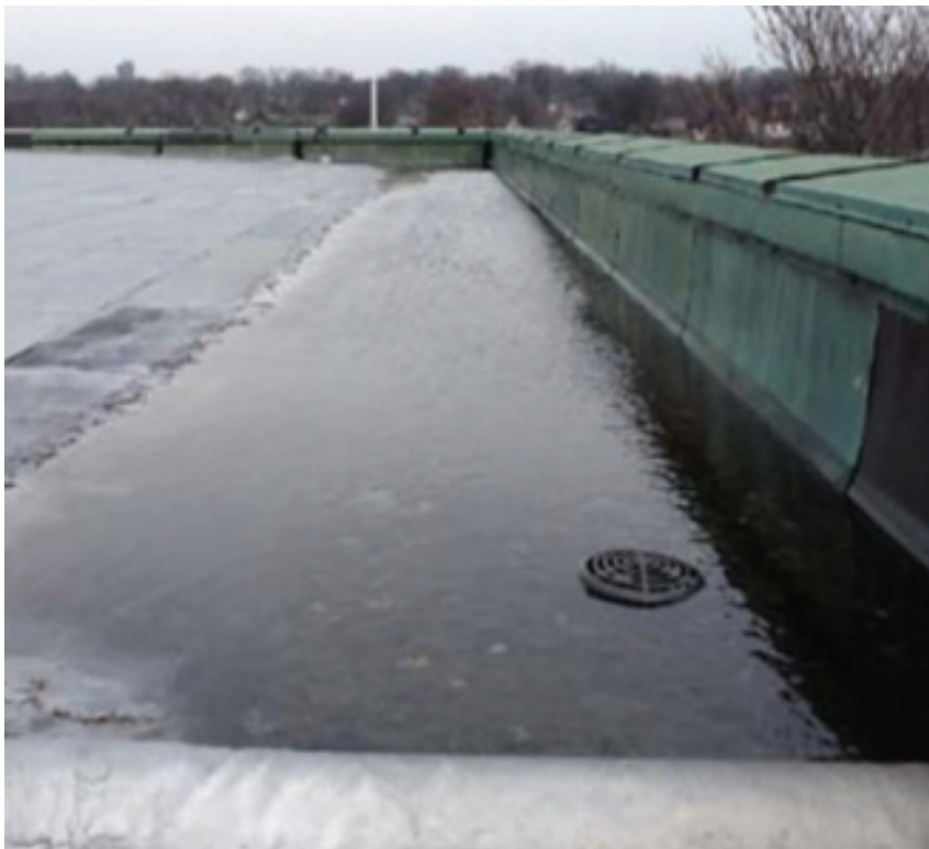
Excessive water accumulation on the roof of Carlaw TS. Ref E6.18, p. 11 and 13.
