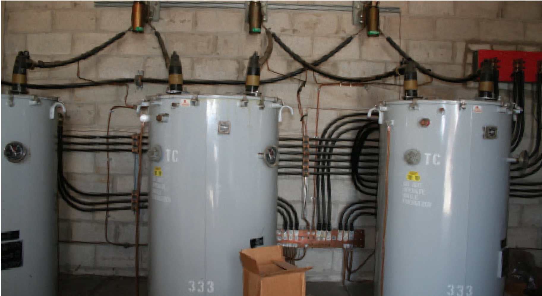
New building vault transformer. Ref: E6.1, p. 9.
