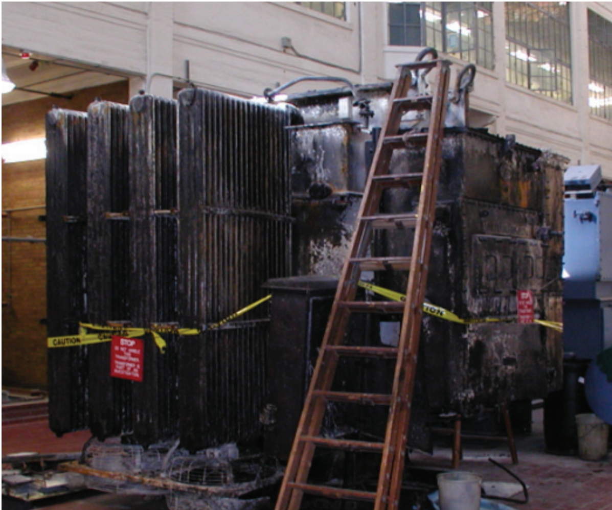
This transformer (pictured above) was damaged in a fire caused by a neighbouring transformer. Toronto Hydro is proposing to install fire systems in stations with two or more transformers. Ref: E6.17, p. 21.
