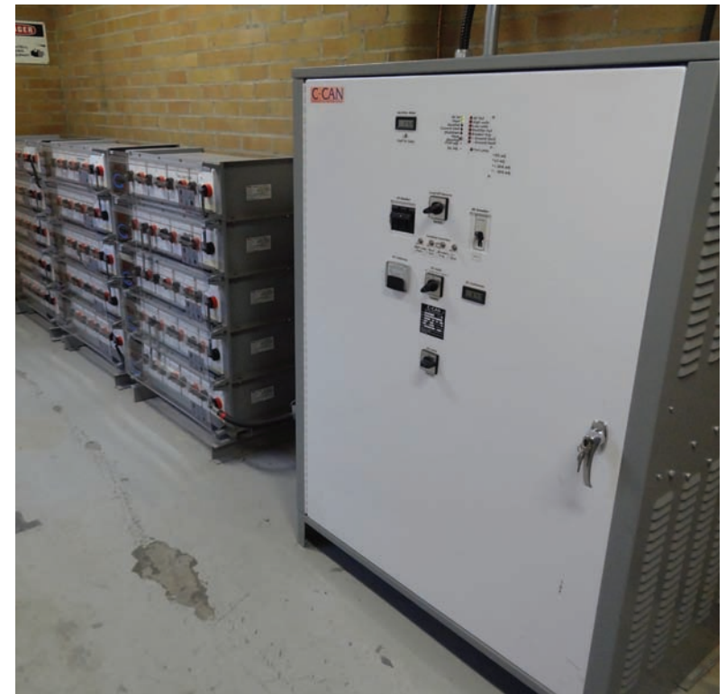
Typical set up of 400Ah battery system (Battery bank on left and charger on right).
