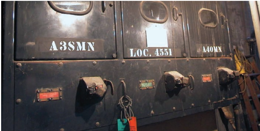
Obsolete Powerlite switches (picture left) were installed in the mid-1960s and are no longer manufactured. Remaining switches will be replaced due to age, obsolete configuration and safety concerns. Ref: E6.3, p. 1.
