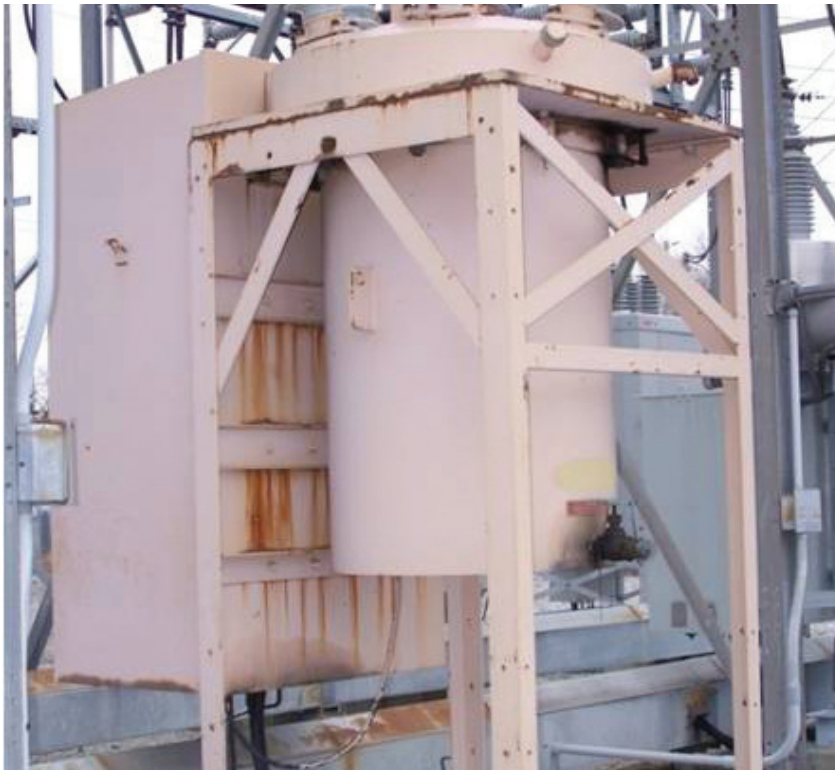
Typical aged and obsolete KSO oil circuit breaker. Ref: E6.15, p. 6 and 9.
