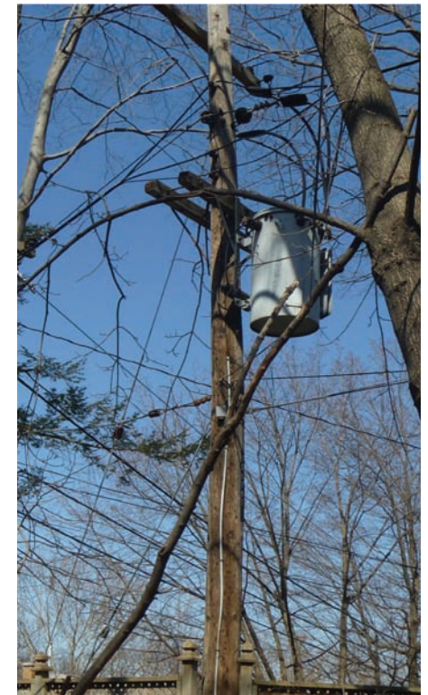
Clearance not met; fence makes it difficult to access pole.
