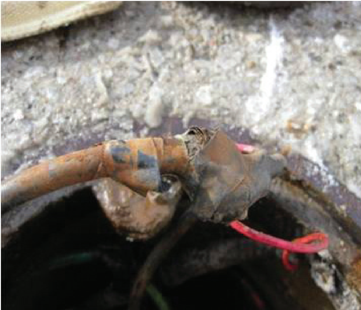
Legacy conductive handwells with defective conductors (pictured above) can become a public safety hazard. Ref: R7.5, p. 9.
