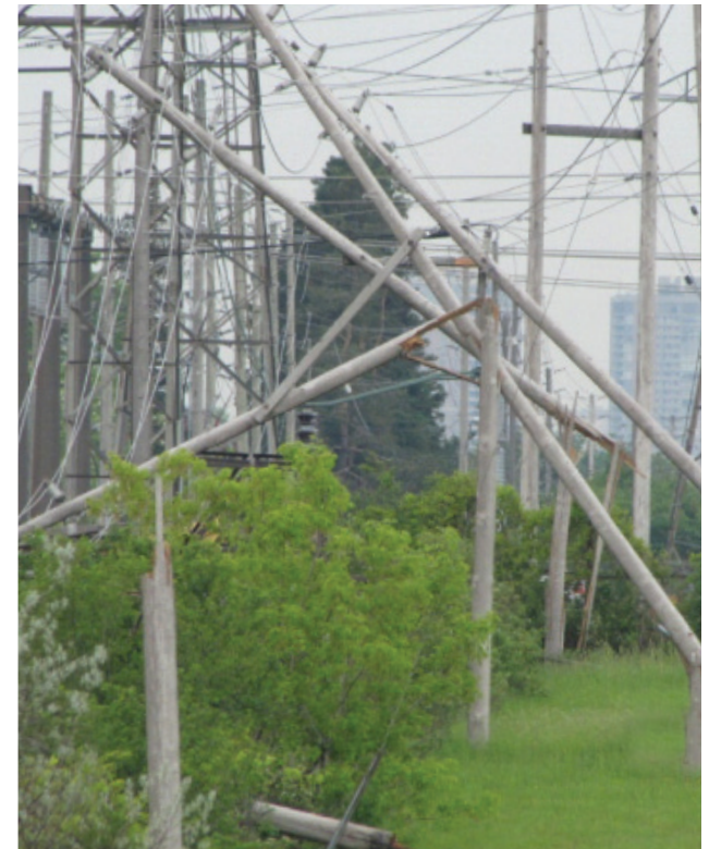
Example of catastrophic pole failure.
