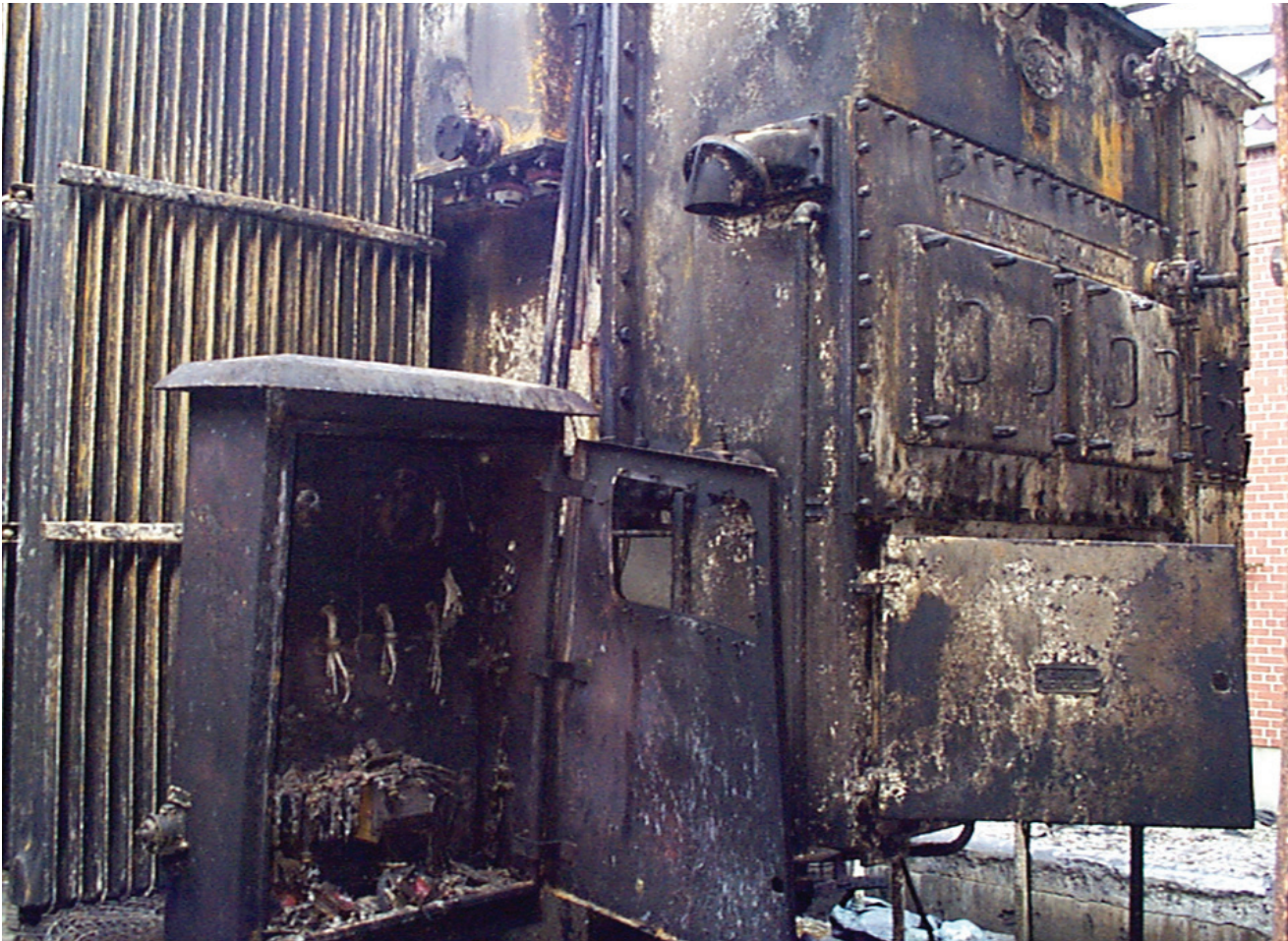
Failed power transformer at Dupont MS. Ref: E6.14, p. 20.
