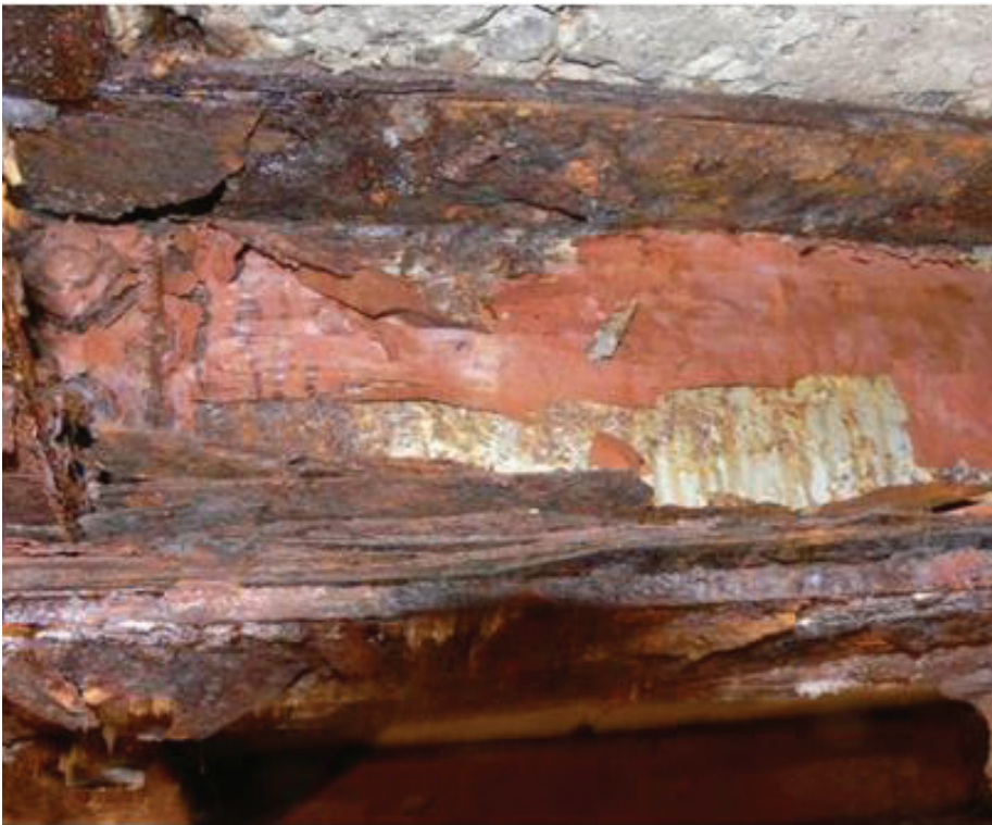
Corroded i-beams. Ref: E6.9, p. 17.
