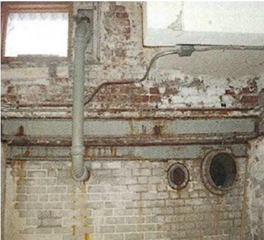
Corrosion on the foundation walls of Terauley station.
