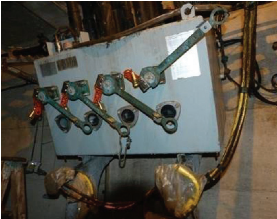
Existing submersible vintage URD switch. Ref: E6.1, p. 18 and 1.
