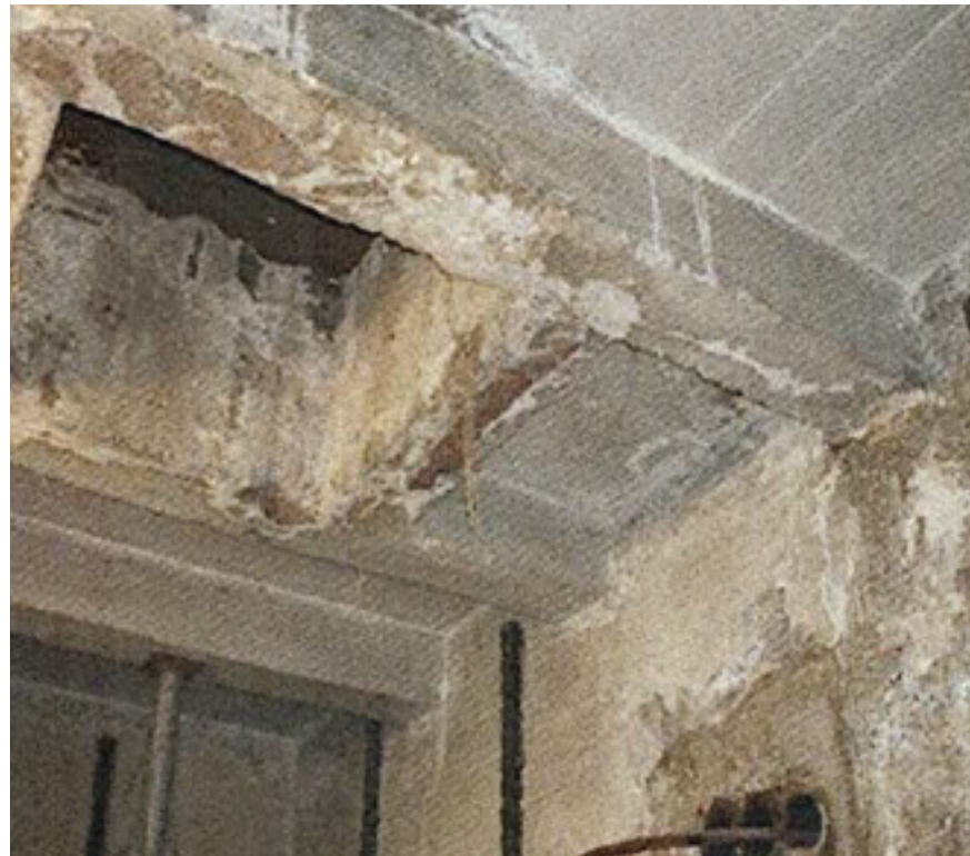
Cable chamber wall and roof framing deterioration at High Level station. Ref: E6.18, p. 17 and 20.
