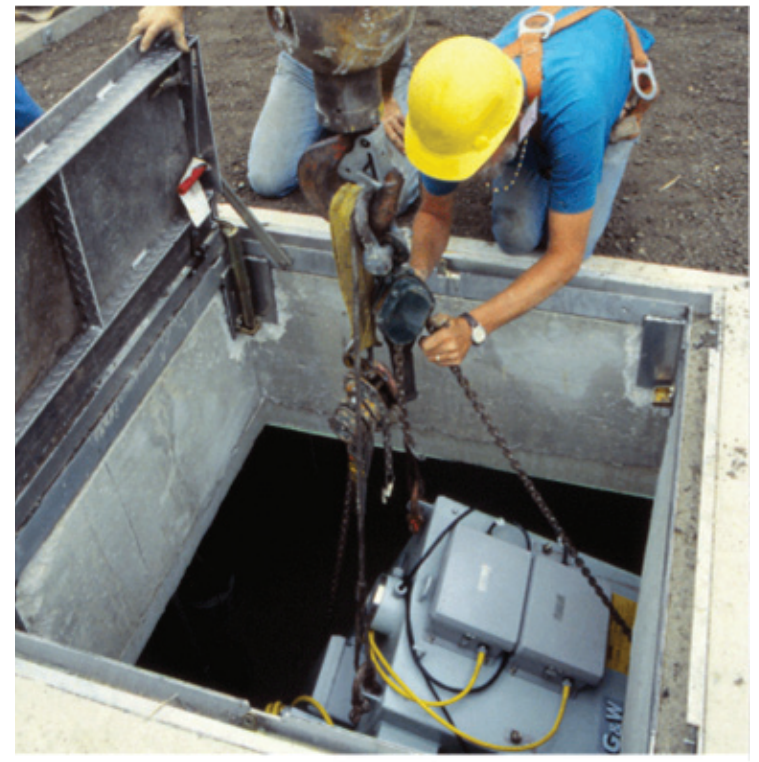
New submersible and/or building vault SF6-insulated switch.
