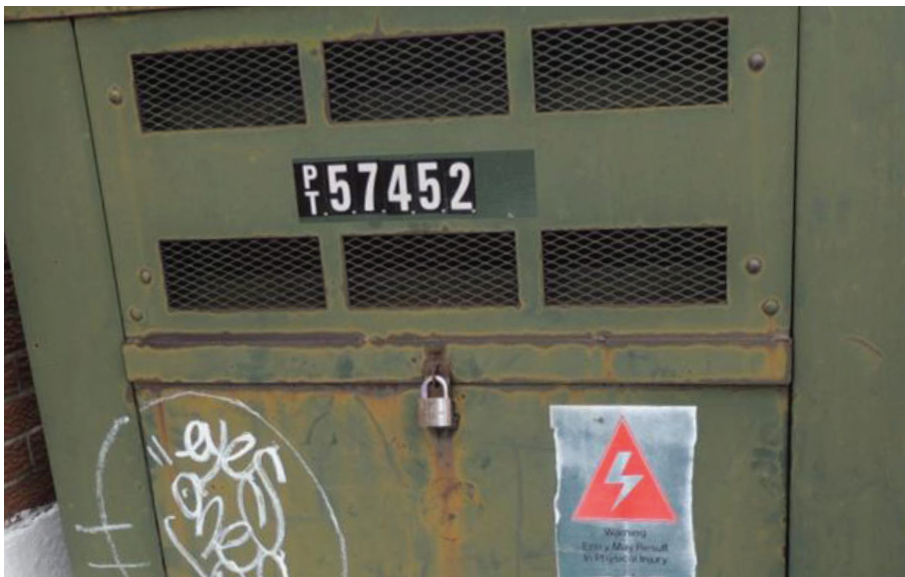
Corroded and damaged transclosure enclosures. Transclosures are an obsolete underground transformer type with no like-for-like replacement options. These assets are difficult to restore in the event of an outage. Ref: E6.3, p. 24.
