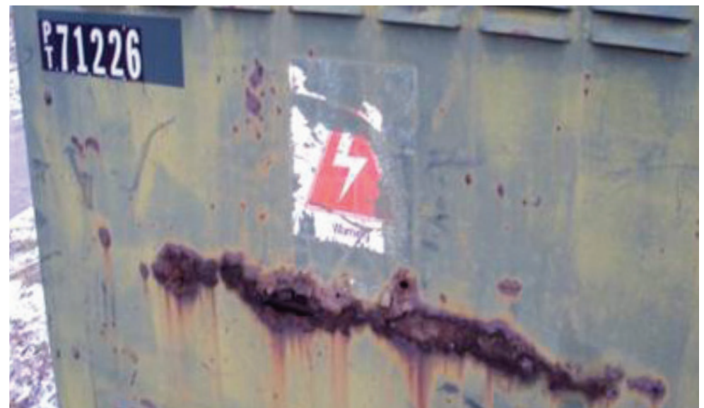
Corroded and damaged transclosure enclosures. Transclosures are an obsolete underground transformer type with no like-for-like replacement options. These assets are difficult to restore in the event of an outage. Ref: E6.3, p. 24.
