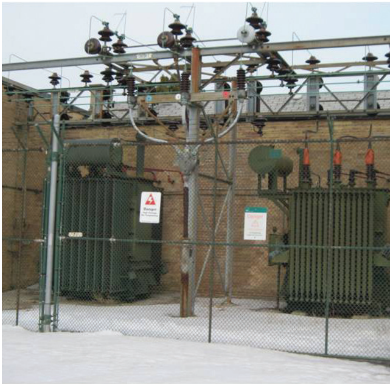
The transformers and overhead bus structure (pictured above) are obsolete and have reached their end-of-life. Ref: E6.14, p. 9 and 7.
