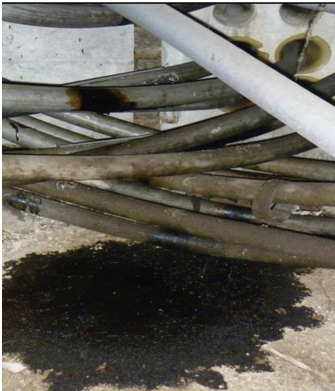
Leaking PILC cable with oil pooled on floor of chamber. Ref: E6.2, p. 6 and 1.
