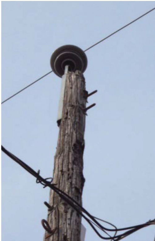
Pole-top cracking. Ref: E6.4, p. 17, 7 and 35.
