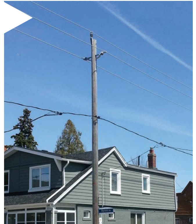
Pictured left: Box construction pole prior to conversion. Pictured right: The same pole after conversion to standard 13.8 kV configuration.
