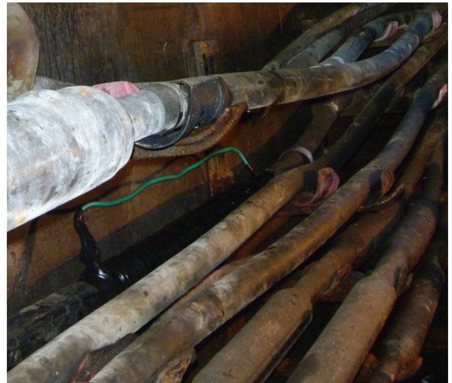
Cable chamber with properly racked cables.
