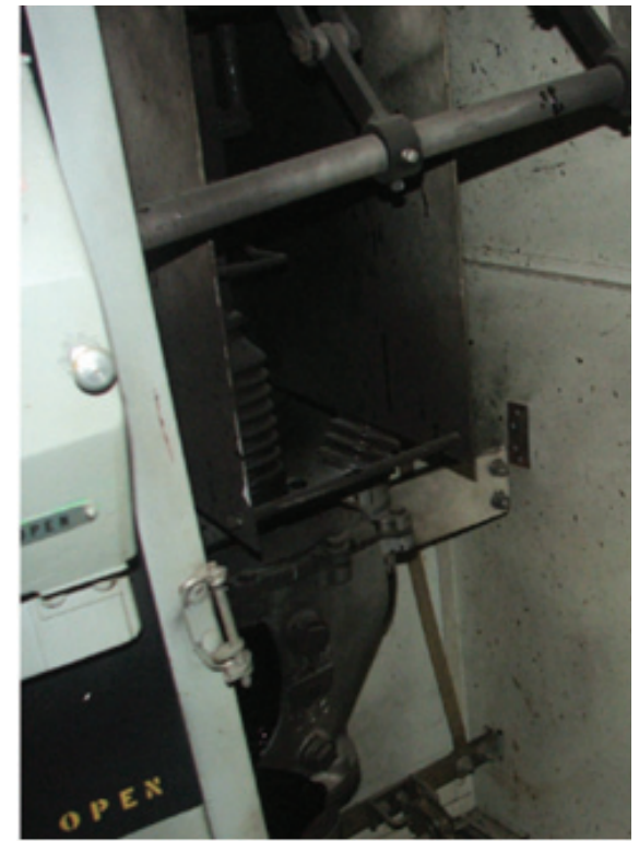
Impact of an internal arc fault in switchgear at Terauley TS.
