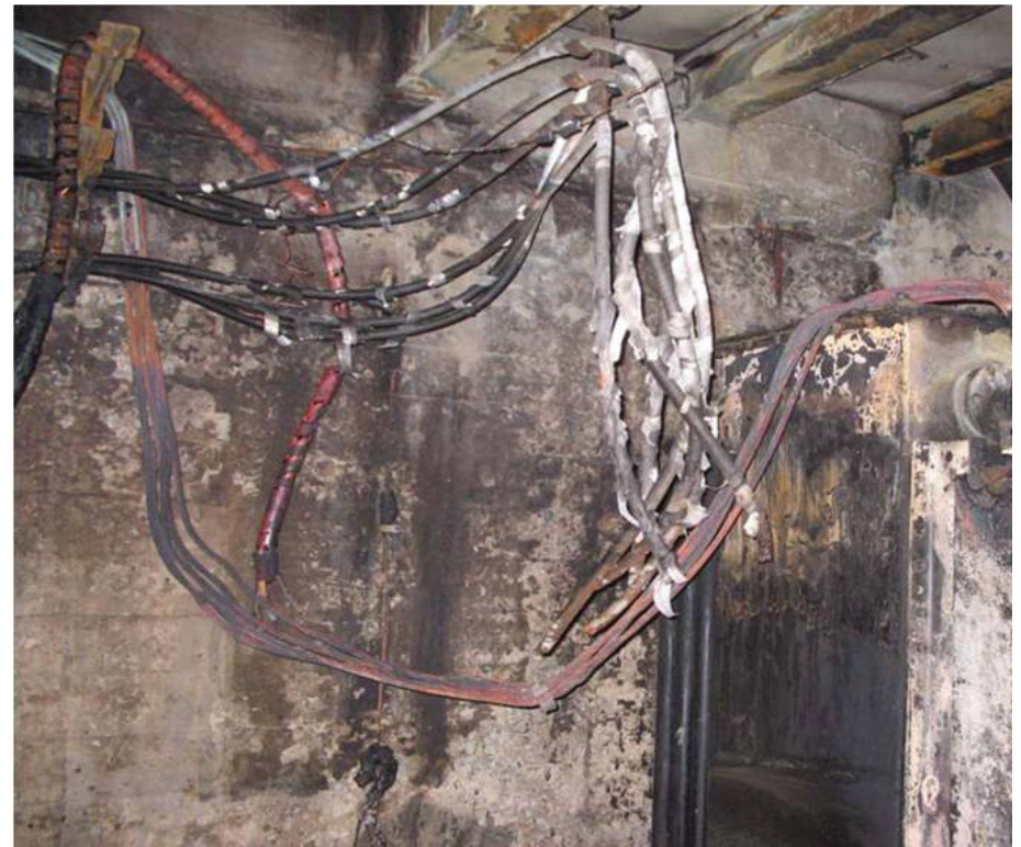
Burnt AILC secondary cables. Ref: E6.20, p. 8.
