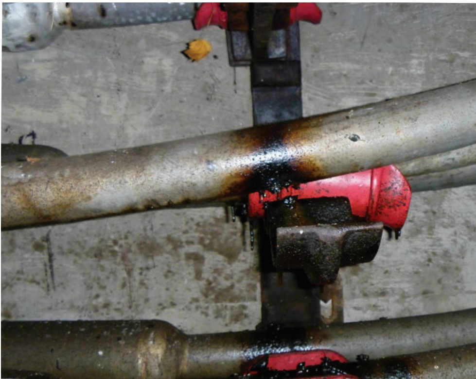
Oil leaking from PILC cable. Ref: E6.2, p. 13 and 10.
