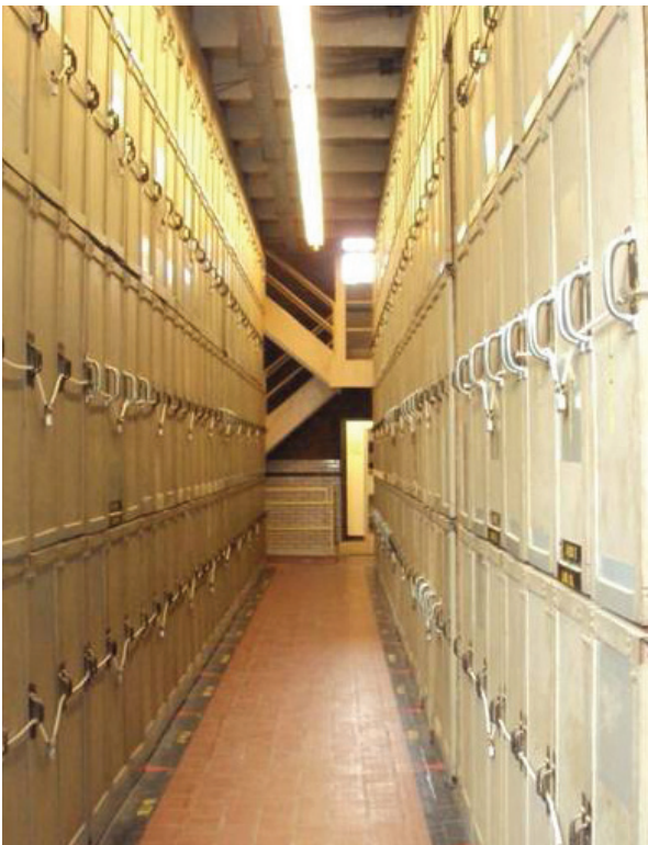
Aged and obsolete non-arc resistant brick structure TS switchgear at Carlaw TS. Ref: E6.13, p. 6, 10 and 29.
