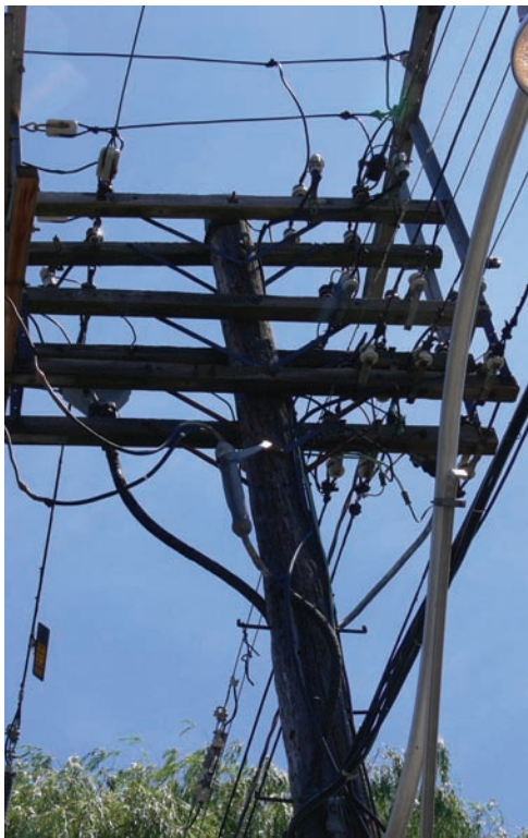
Typical box construction design features a number of live, tightly packed circuits. Ref: E6.7, p. 1 and 6.
