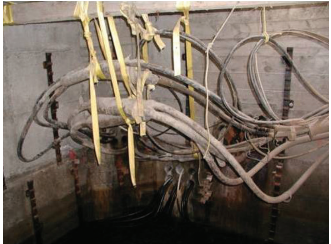
Cable chamber with cables that require piecing out.
