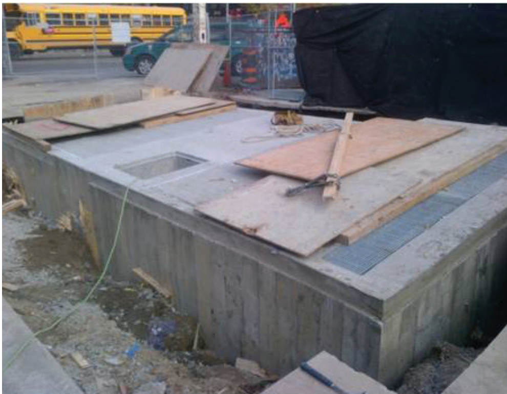
Completed vault rebuild. Ref: E6.9, p. 12.
