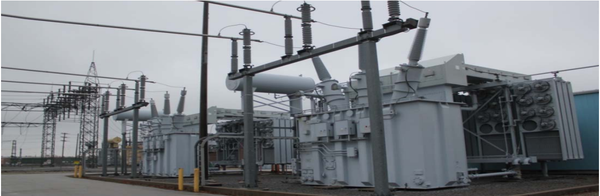
1 Figure 62: The station yard at Cavanagh TS
