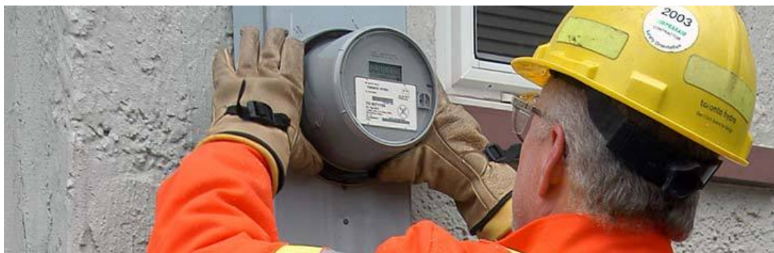
FIGURE 1: TORONTO HYDRO CREW MEMBER INSTALLING SMART METER AT A RESIDENTIAL LOCATION
