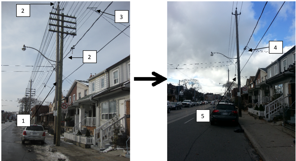
FIGURE 18: EXAMPLE OF BOX CONSTRUCTION CONVERSION JOB. (1) NEW POLES ARE INSTALLED IN CLOSE PROXIMITY TO EXISTING POLES. (2) NEW PRIMARY (TOP) AND SECONDARY CABLE (MIDDLE) INSTALLED (NOT ENERGIZED). (3) NOTE THAT CUSTOMERS STILL SUPPLIED FROM 4.16 KV BOX SERVICE, AND NOT NEW 13.8 KV/27.6 KV SERVICE. (4) CUSTOMERS ARE SWITCHED OVER TO NEW SERVICE. (5) ONCE ALL LOAD FROM CIRCUITS RUNNING THROUGH BOX POLES ARE DE-ENERGIZED, BOX CONSTRUCTION INFRASTRUCTURE (POLES, CIRCUITS, SWITCHES, TRANSFORMERS) CAN BE REMOVED.
