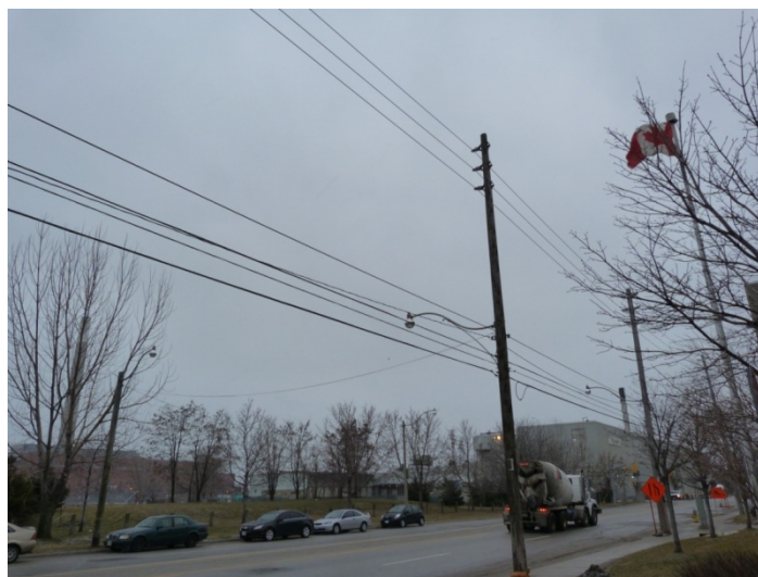
12 FIGURE 3: TYPICAL CURRENT CONSTRUCTION STANDARD 13.8 KV OVERHEAD FEEDER
