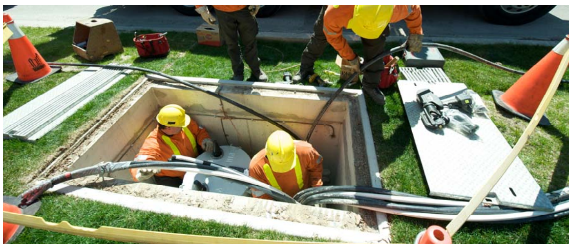
FIGURE 1: TORONTO HYDRO CREWS INSTALL A NEW UNDERGROUND TRANSFORMER
