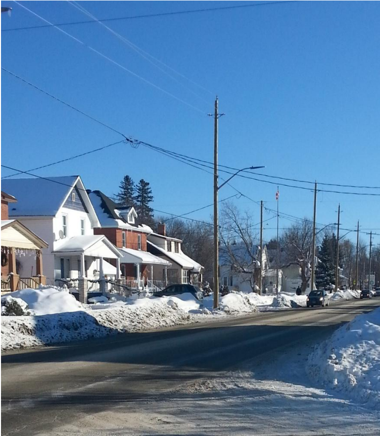
1. Corner of Cassells and Princess looking North – Jan, 2015. These are the poles and wires following replacement work re voltage conversion.
