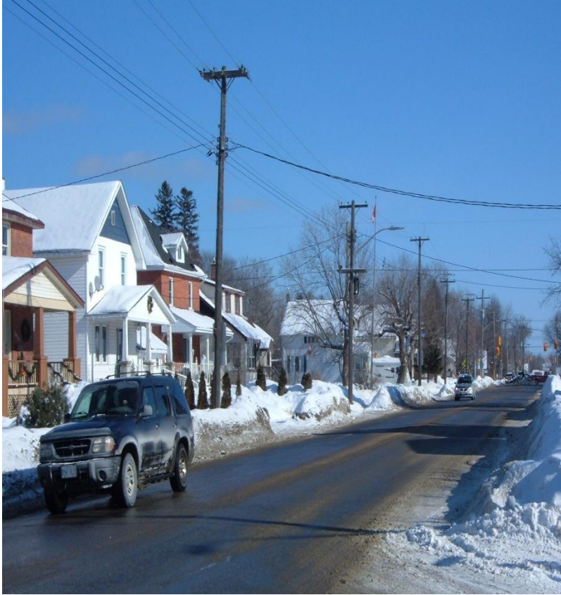
2. Corner of Cassells and Princess looking North – Feb, 2013. These are the poles and wires before any replacement work re voltage conversion.
