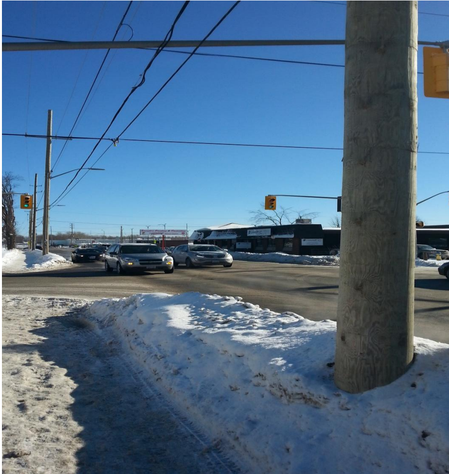
3. Cassells and Olive looking North – Jan 2015. The remaining new pole following removal the old one.
