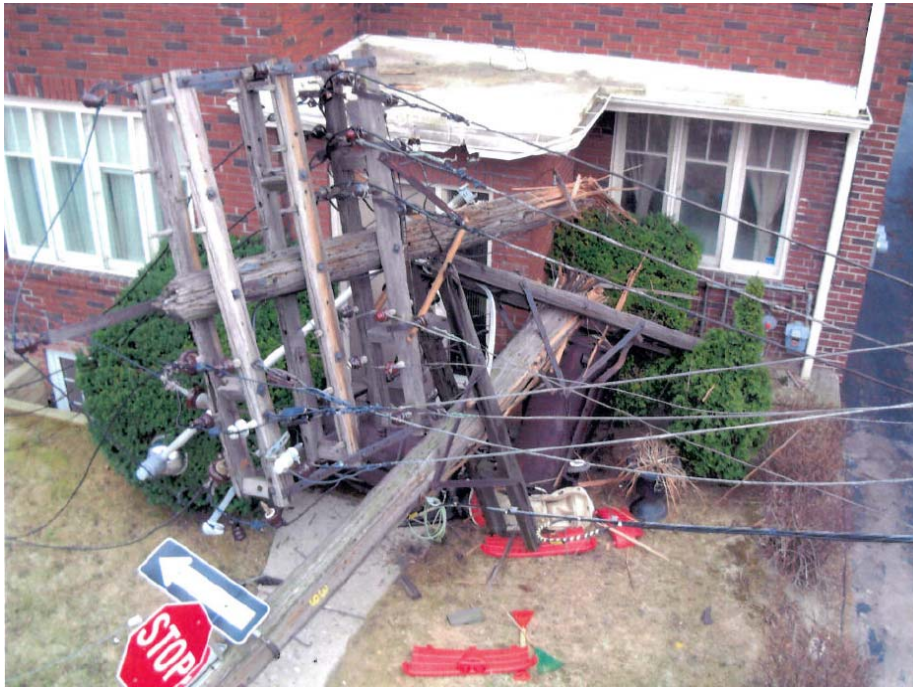
1 Figure 8: Fallen pole due to rotten base
