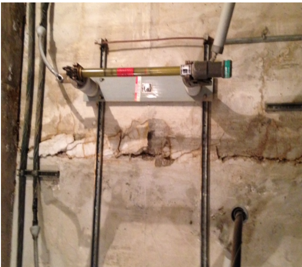
Figure 55: Cracked Walls
