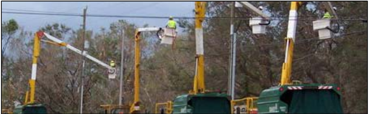
Figure 20: Tree Trimming of an Overhead Feeder
