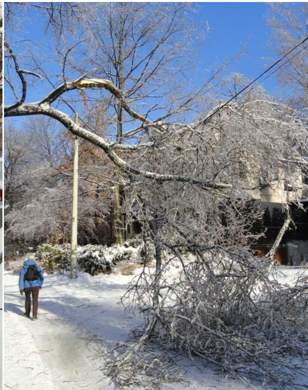
1 Figure 12: Tree branches and damage to overhead conductors caused during the 2 2013 Ice Storm.
