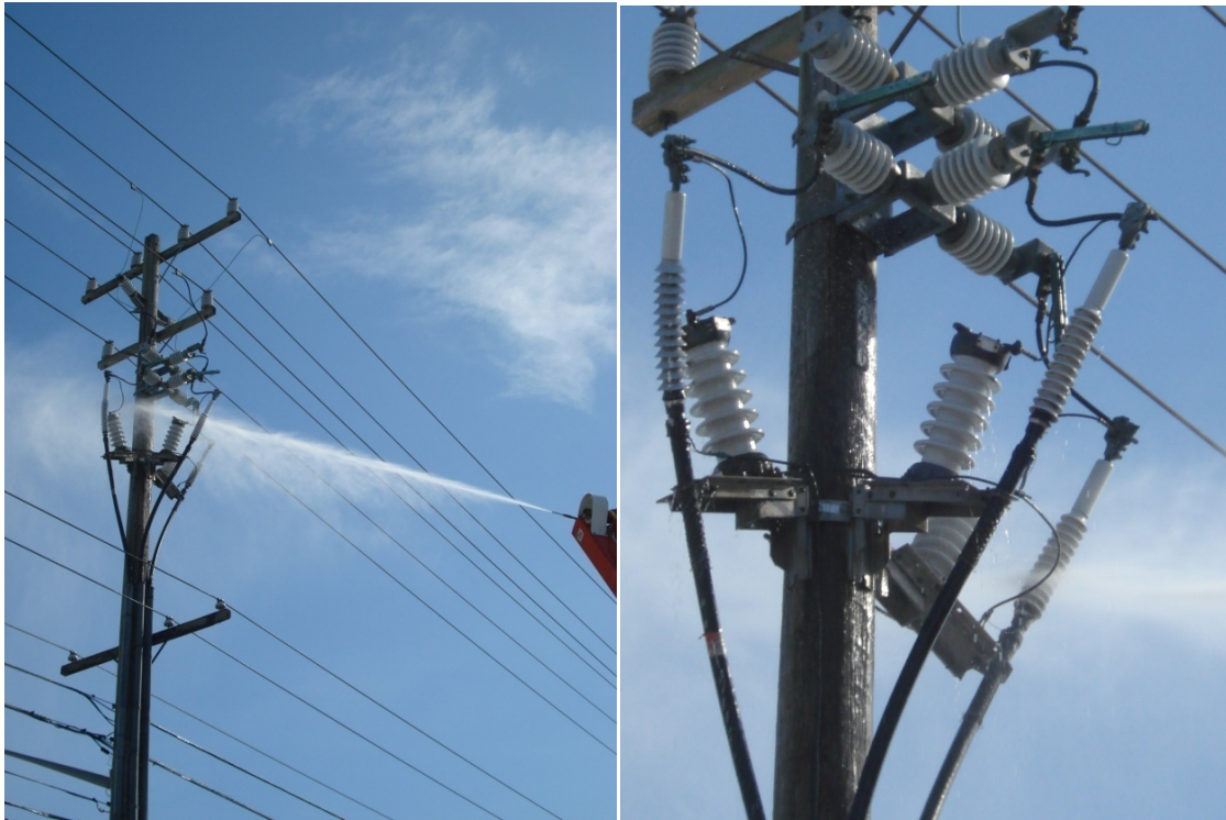
5 Figure 11: Porcelain Insulator Washed using a High Pressure Water Jet
