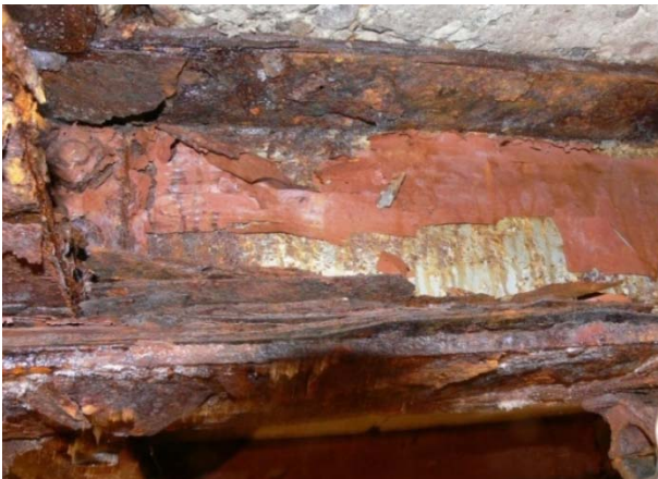
Figure 25: Corroded I-Beams
