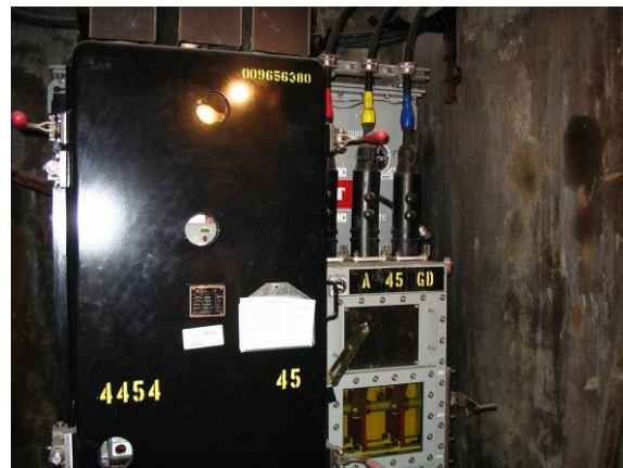
Figure 4-16 Example Transformer/Protector Units
