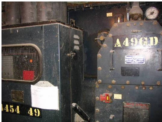
Figure 4-16 Example Transformer/Protector Units
