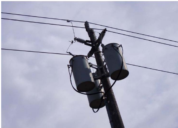
3 phase pole mounted transformers
