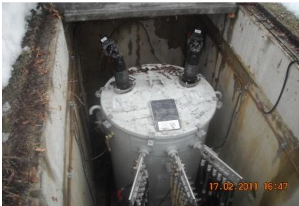
Submersible transformer
