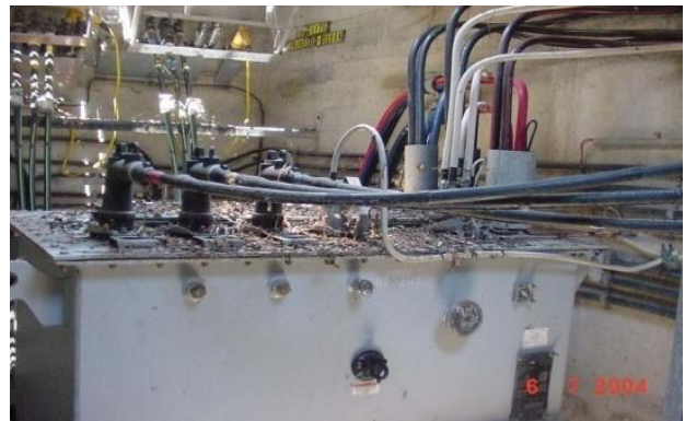
3 Phase submersible transformer
