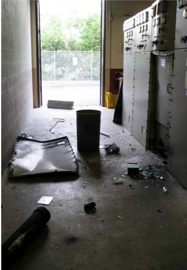
Figure 12 - Station Switchgear Explosion
