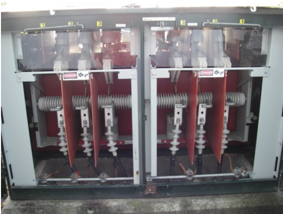
Figure 47 – Inside of air-insulated switchgear
