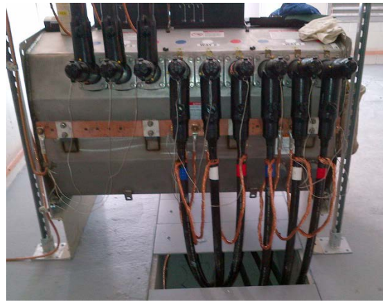
Figure 48 - Inside of SF6 underground switchgear
