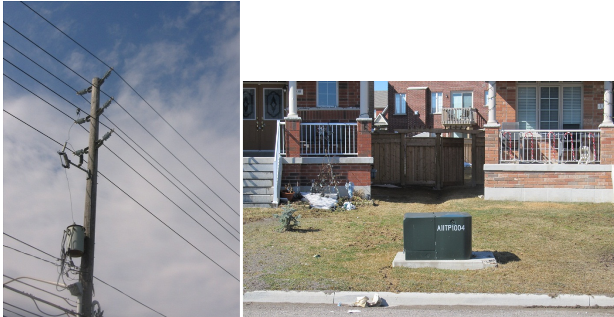
Example of overhead distribution system (left), as well as residential padmount transformer associated with an underground distribution system (right)
