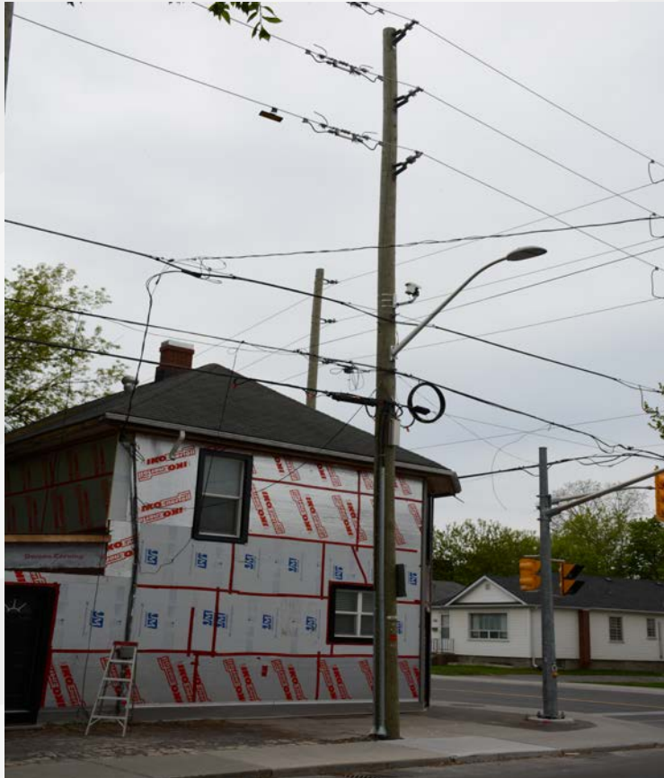
Pine Street Post Reconstruction
