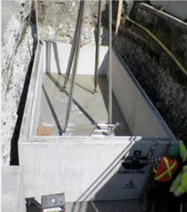
New Pre-cast Concrete Vault
