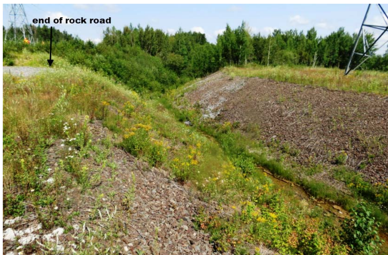
Figure 10 - Restored Site Two Years after the Removal of the Temporary Culvert
