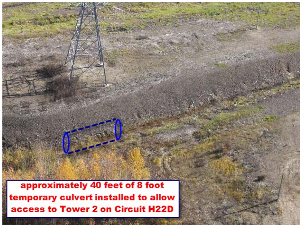
Figure 8 - Pre-Construction Site photo Showing Location of Temporary Culvert Installation
