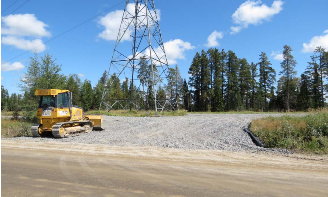
Figure 5 - Tower Pad Construction on Tower 4 on Circuit L20D
