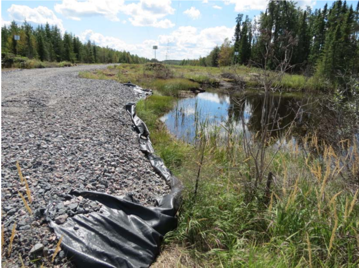
Figure 3 - Avoiding wetlands with new rock road construction
