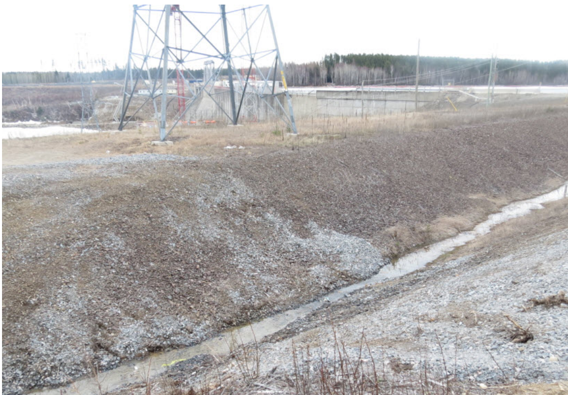
Figure 9 - Restored Site after the Removal of the Temporary Culvert
