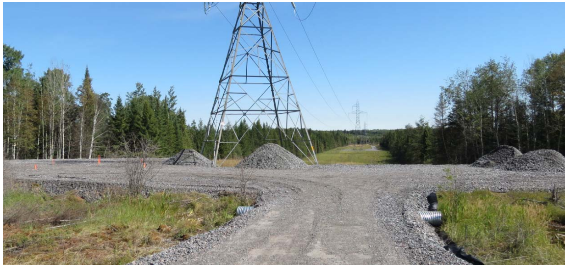
Figure 2 - Building Rock Construction Pads on circuit L20D Tower 12 (in foreground) and 13 and 14 (in background) 5
