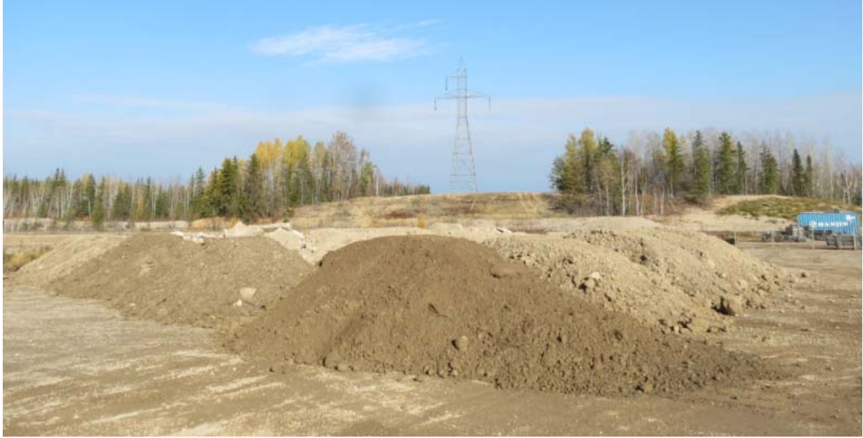
Figure 6 - Clean excavated fill piled on Hydro One transmission corridor for disposal on site
