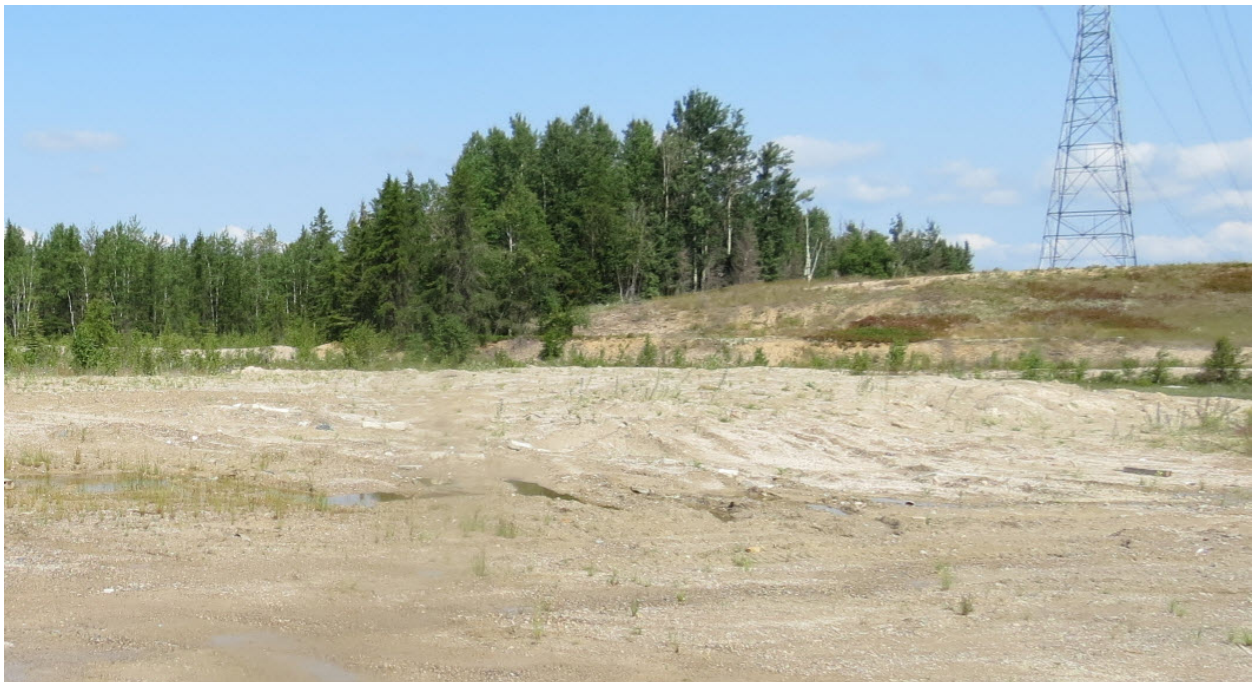
Figure 7 - Clean excavated fill spread out on Hydro One corridor for disposal on site
