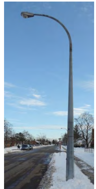
Figure 33 Typical Pole-Trans Roadway Lighting Pole
