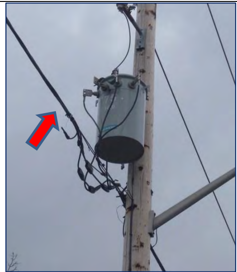
Figure 3-11 Example of Modern Spun Secondary Bus System
