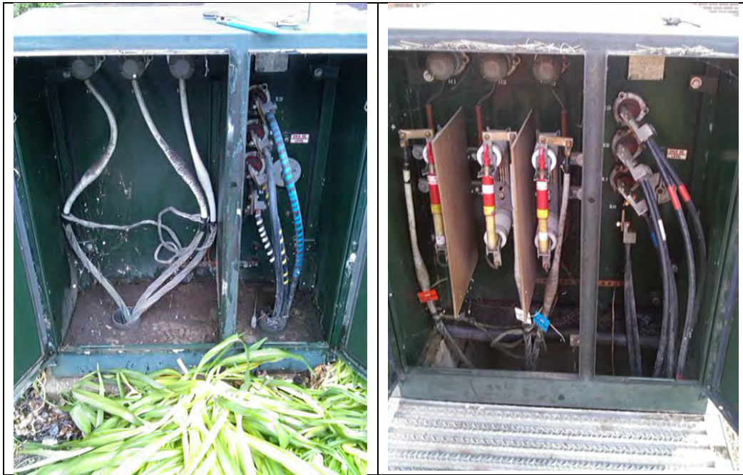
Figure 4-5 Inside Typical Live-Front Transformers
