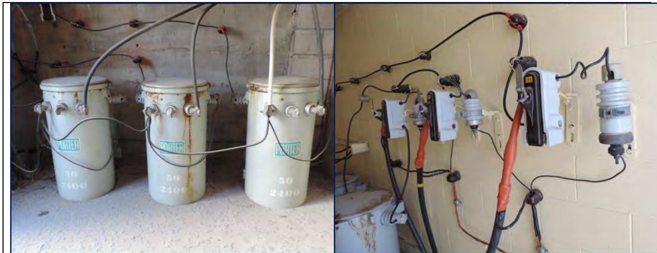
Figure B.1-1, Typical Arrangement of Distribution Transformers in Vault
