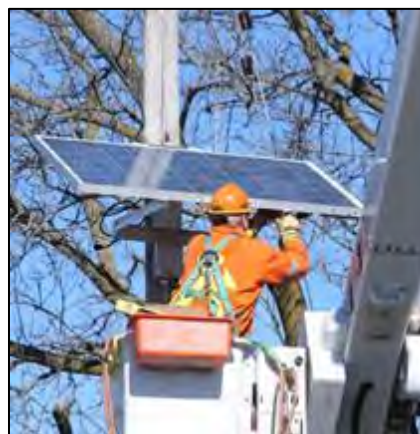
Figure 3-16 Typical solar panel being installed on pole.
