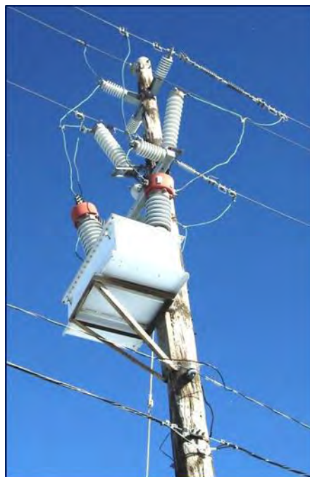
Figure 7-1 Typical Ferranti-Packard KMD46 Primary Metering Unit Installation
