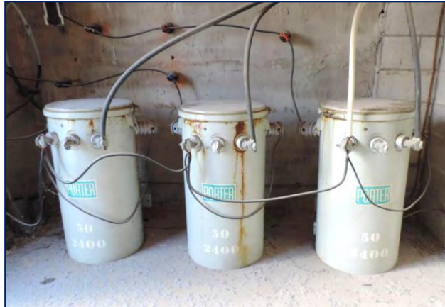
Figure 4-7 Typical Transformer Arrangement within Vault
