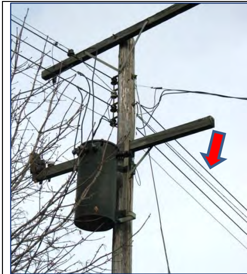
Figure 3-10 Illustration of Vintage Open Secondary Bus System
