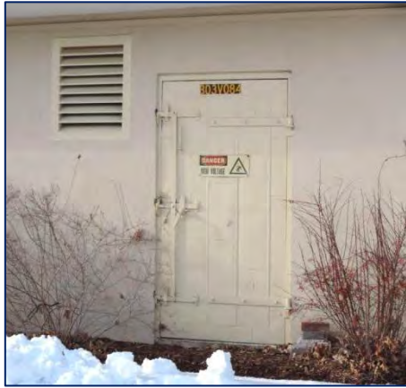
Figure 4-6 Typical Vault Access Door and Ventilation Vent
