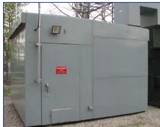
Figure 6-3 Typical Prefabricated Switchgear Building
