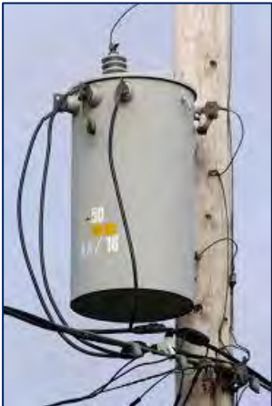
Figure 3-3 Typical Pole-Mounted Distribution Transformer
