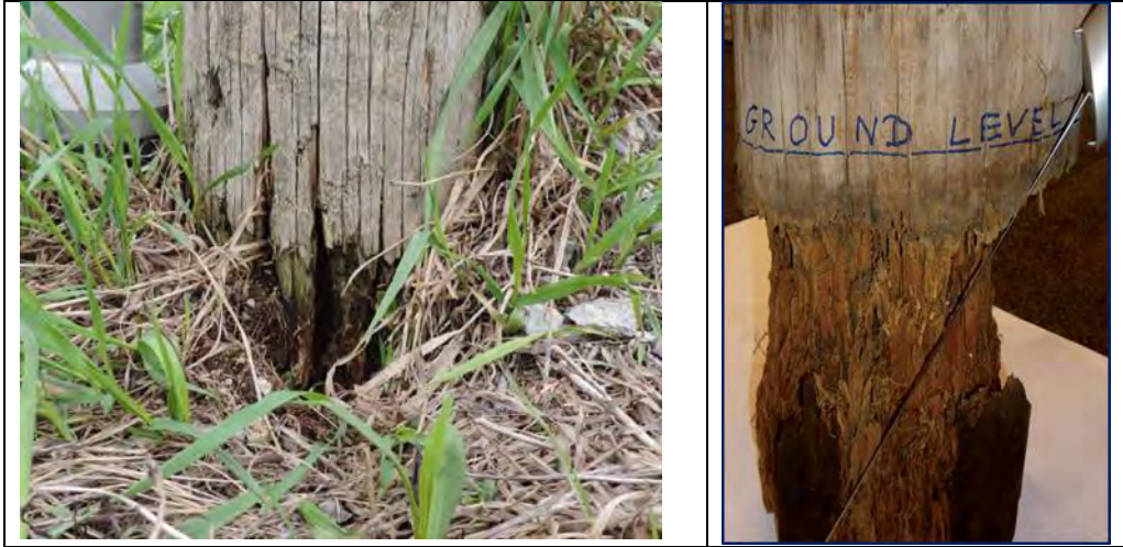
Figure 3-2 Examples of Carpenter Ant Damage (left) and Severe Ground-Line Decay (right)
